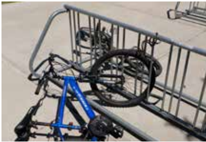
Rack does not provide 2 points of support or place to lock to frame (Photo: MIG/SvR)
