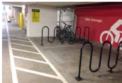
Racks do not provide 2 points of support & there is no delineated bike exit (Photo: Alta Planning + Design)
