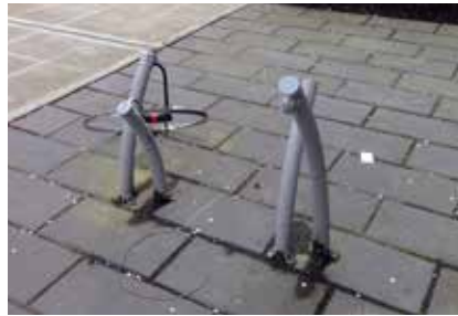
Non-intuitive rack does not provide 2 points of support (Photo: Alta Planning + Design)
