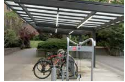
Racks under a shelter with lighting & repair station at UW (Photo: MIG/SvR)
