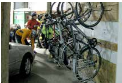
Anchoring is not theft resistant (Photo: MIG|SvR)
