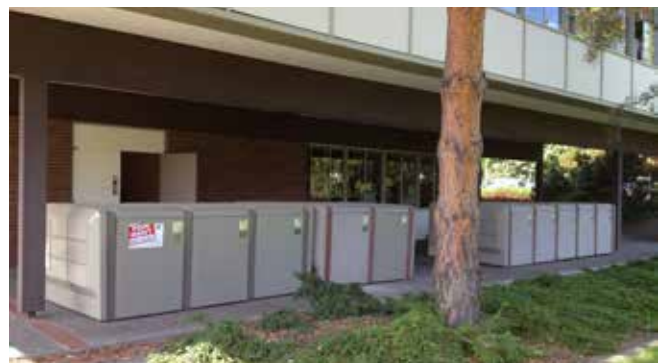
Bicycle lockers protected under building cover (Photo: Alta Planning + Design)
