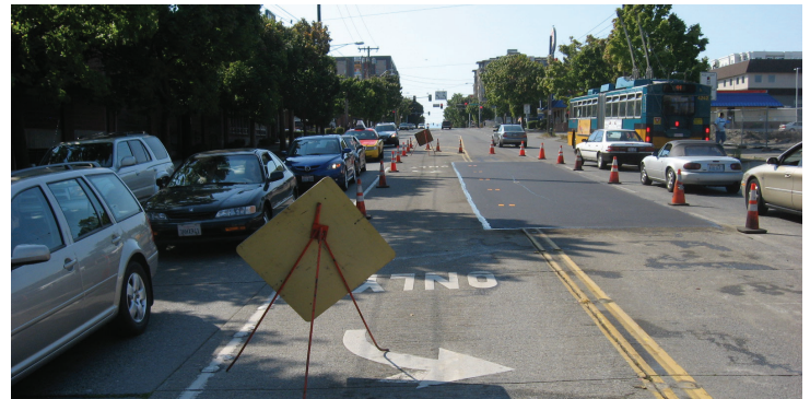
Spot repair on NW Market St.
