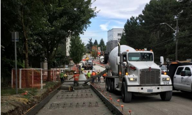
Construction on Delridge RapidRide H Line project
