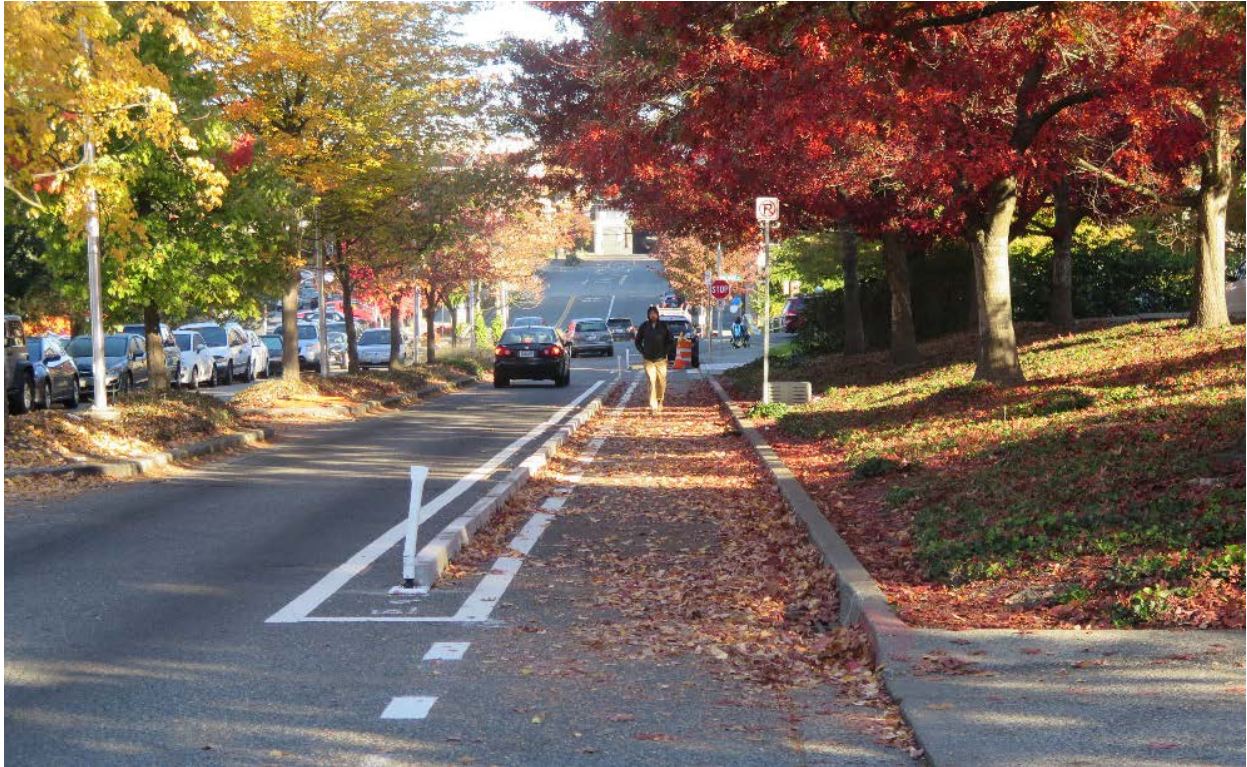
Low-cost sidewalk on 3rd Ave NE
