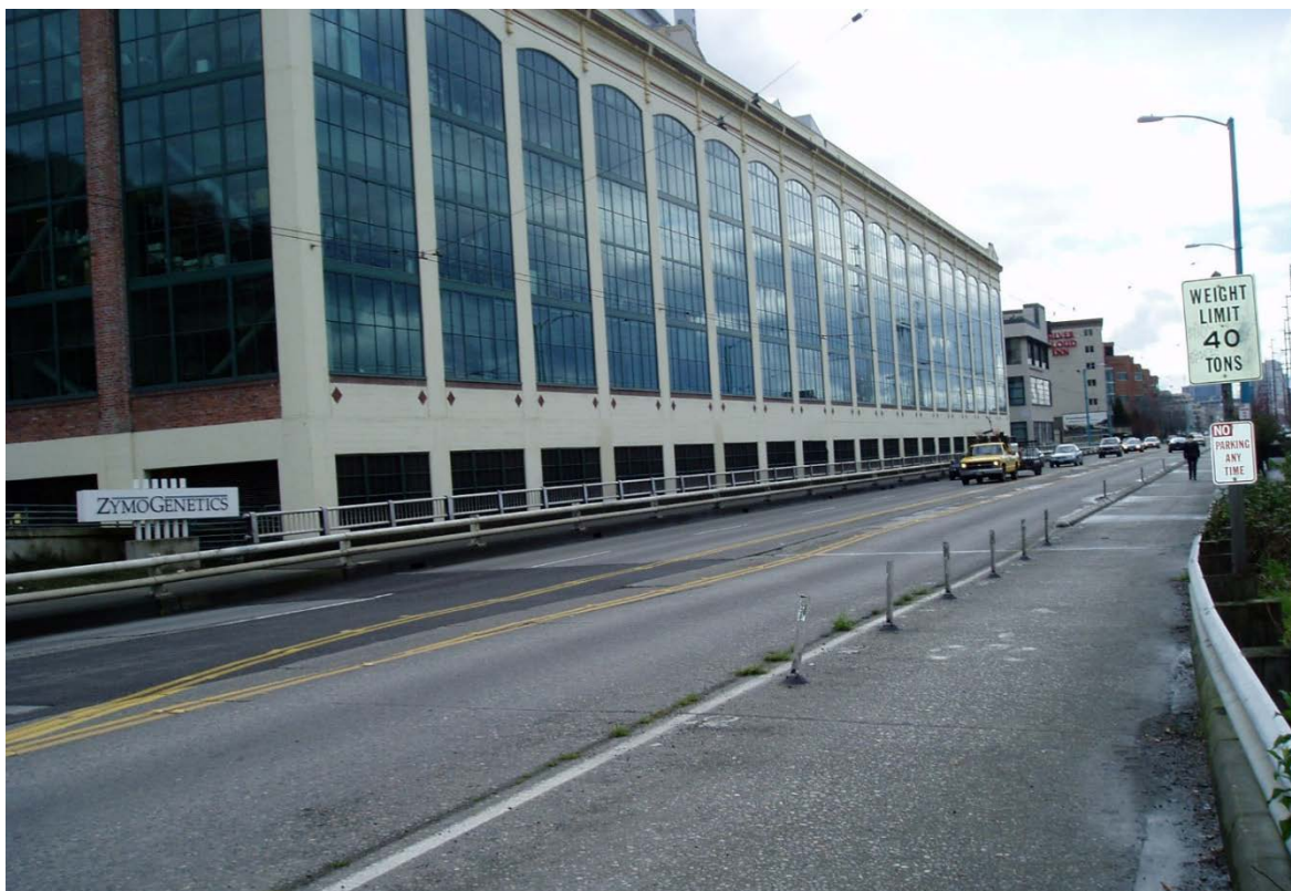
Existing conditions on Fairview Ave N
