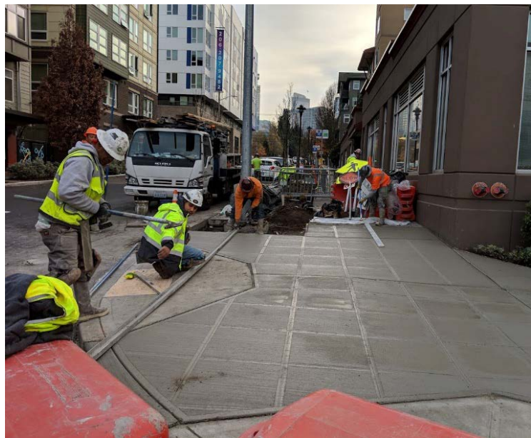
Finishing new curb ramp
