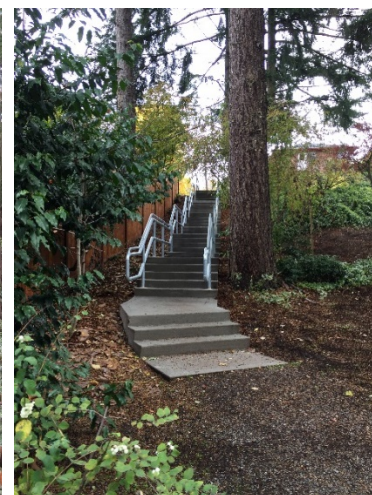
N 88th St stairway, after
