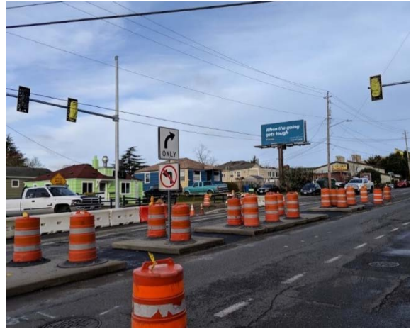
Work underway for greenway crossing at Greenwood Ave N/N 100th St
