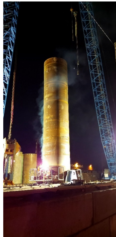
Crews weld shaft casing for Lander Bridge
