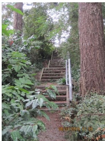
N 88th St stairway, before
