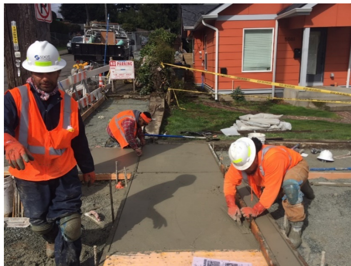
Crews building sidewalk
