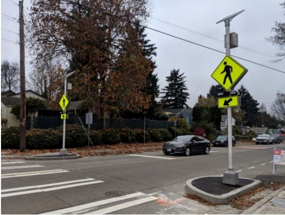
New sidewalk corner and bike ramp on Rainier Greenway
