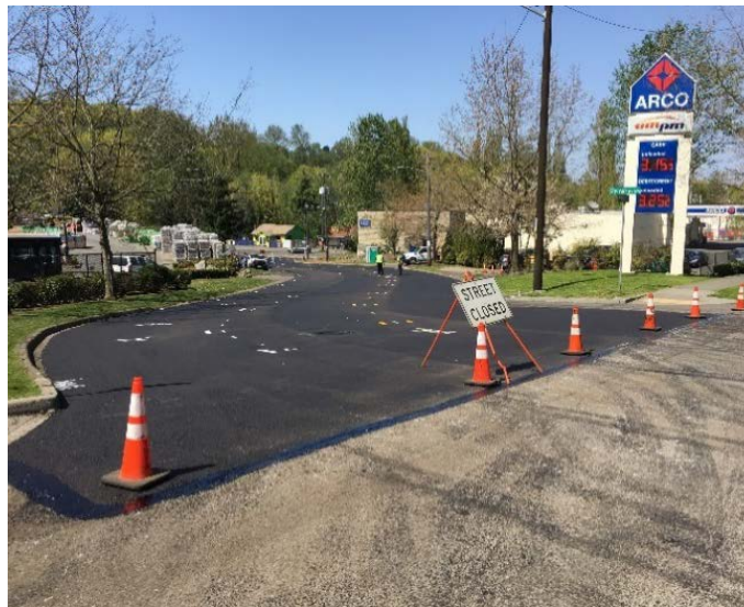
Pavement after repair
