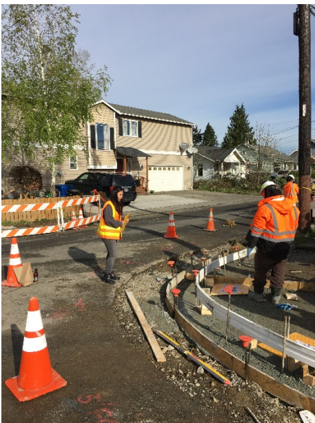
Forming new curb ramps and sidewalk corner
