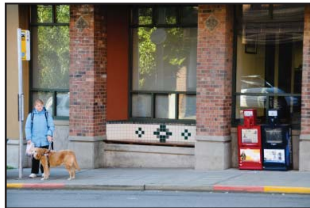
The integration of bus waiting facilities into building frontages avoids the need for free-standing transit shelters
