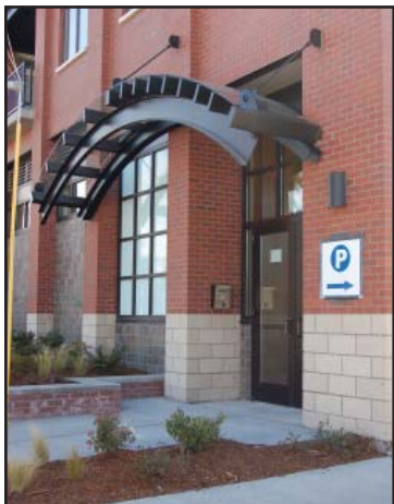
Residential entries should be visible from the sidewalk and landscaping is encouraged
