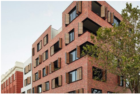
Operable windows at upper-levels add human scale with an ever-changing facade. The notched parapet and corners breakdown bulk of the form.
