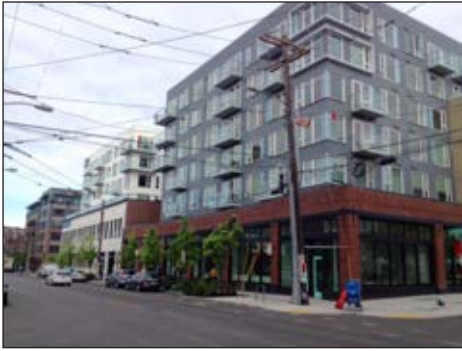
Large development site with massing that creates the appearance of a grouping of smaller structures.
