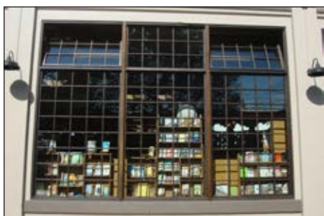
Window trim detailing.
