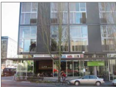
Use of modern materials
