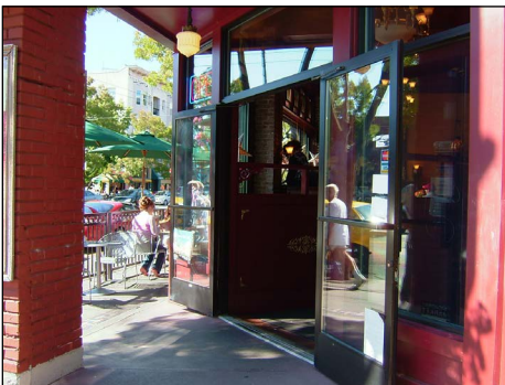
An example of a well-marked, articulated building entrance that is oriented to the sidewalk and provides overhead cover.
