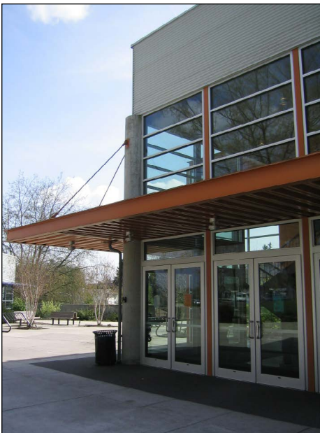
An example of well-designed overhead weather protection in New Holly.
