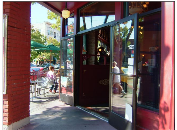
An example of a well-marked, articulated building entrance that is oriented to the sidewalk and provides overhead cover.
