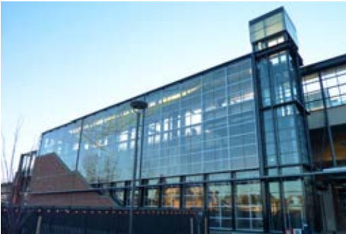
Mount Baker Light Rail station.
