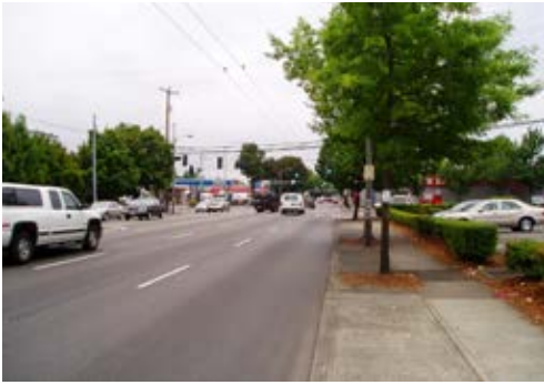
Most of the existing sidewalks along Rainier Ave. are narrow and provide no buffer from the passing car traffic for pedestrians.
