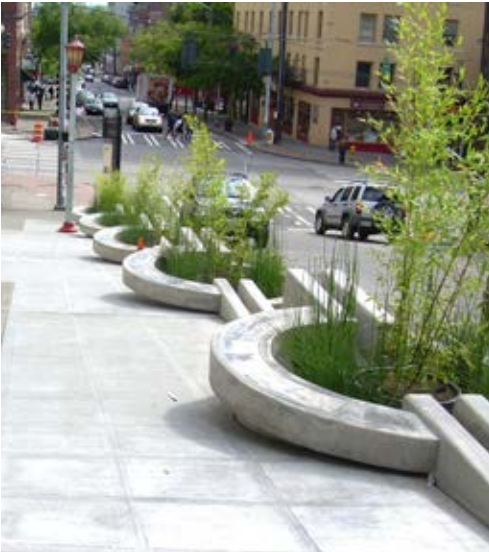
Cascading stormwater feature: These cascading concrete pools and landscaping along Maynard in the International District are a good example of capturing and controlling the flow of stormwater on a sloping site in an artistic and engaging design.
