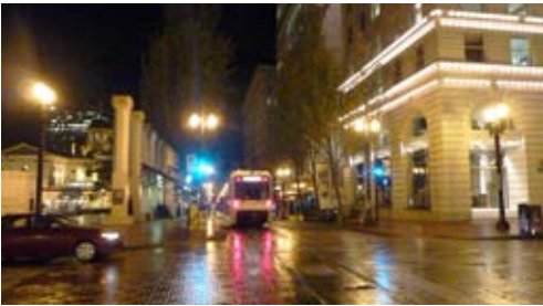
Effective street lighting.
