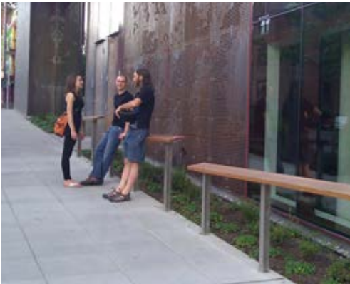
Example of lean rails.
