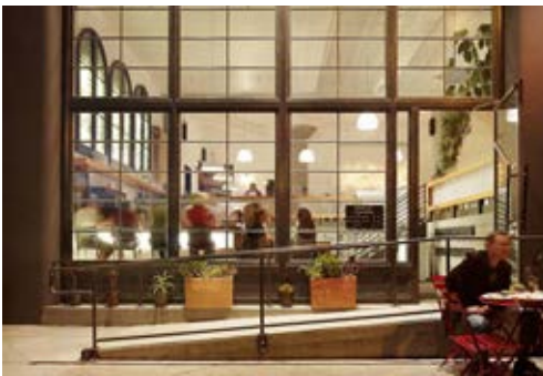
Access, visibility, & character: Barrier-free access accommodates all users, railings and plants add texture to the building edge, low sills and a high level of transparency increase visibility, and high quality materials and rhythm create a pleasing facade. (Mathew Millman Photography, Architizer)
