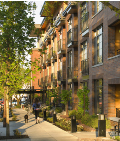
Finely scaled building features & rhythm: This building increases the level of detail below 30 feet in height, using operable windows with divided panes, natural and durable materials, and pedestrian lighting. Window headers are expressed with brick soldier courses. (Ankrom Moisan Architects)
