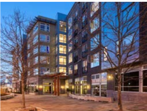
Well-illuminated public space.
