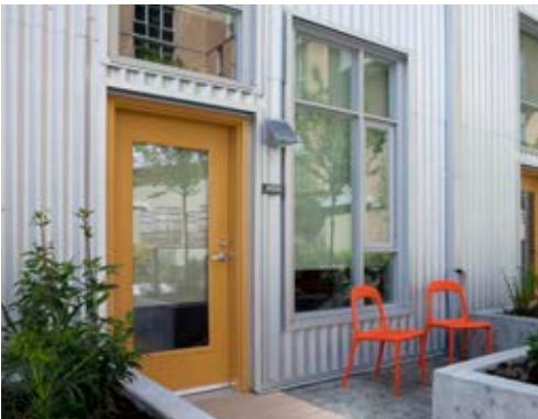
High quality windows: Aluminum windows integrate nicely with the metal facade on this residential building. (Gregg Galbraith Photography)
