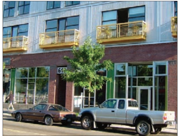
Brick, large storefront windows and masonry kick boards exhibit a sense of permanence at the street.
