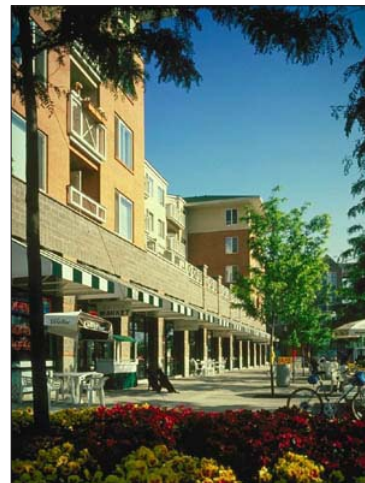
The horizontal dimension of this large, mixed-use building is emphasized through massing and a change of materials to relate well in scale to the pedestrian on the street.
