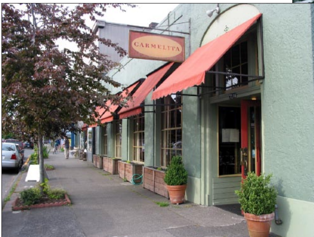
Figure A-8: Carmelita's (Greenwood Avenue North between North 70 th and North 75 th Streets). Streetfront windows highlighted with awnings and planter boxes make this simple building attractive from the sidewalk and street.
