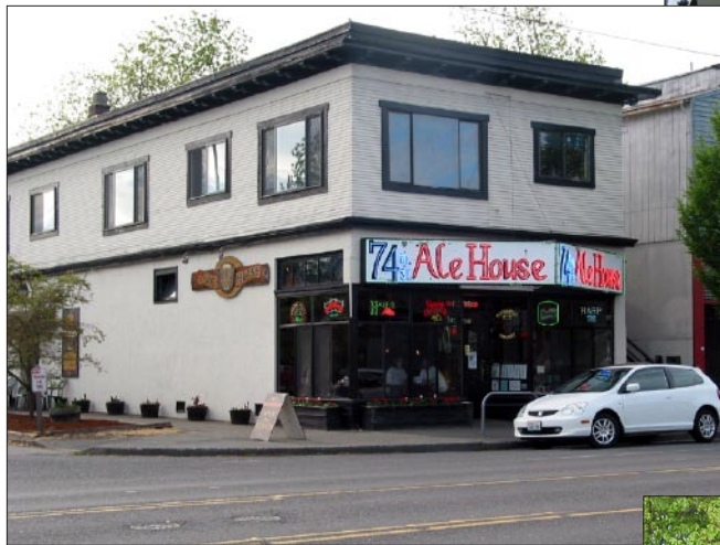
Figure A-3: 74 th Street Ale House (Greenwood Avenue North and North 74 th Street). This building's modest scale, traditional storefront features, and surrounding landscaping treatments make it a positive feature of the neighborhood.
