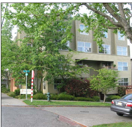
The small, heavily landscaped setback of this residential building on Greenwood Avenue North and North 76th Street enhances the residential environment.
