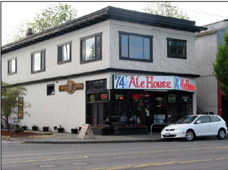
74 th Street Ale House (Greenwood Avenue North and North 74 th Street). This building's modest scale, traditional storefront features, and surrounding landscaping treatments make it a positive feature of the neighborhood.
