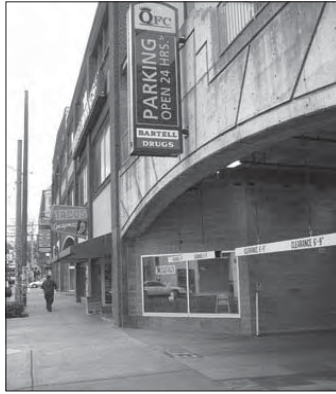
Retail spaces incorporated along street-front facade of a parking structure
