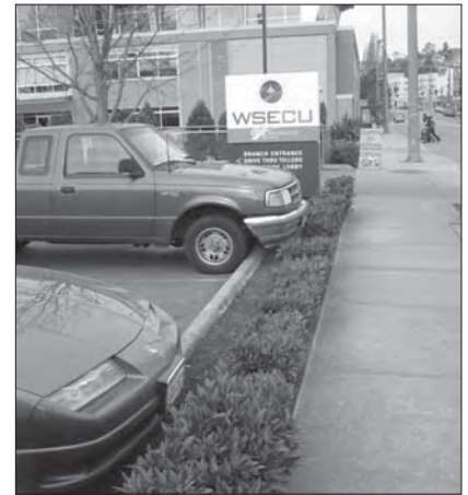
Provide a “wheel stop” at the perimeter of parking areas.
