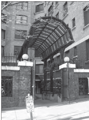
This distinctive weather canopy defines an entry and provides cover.
