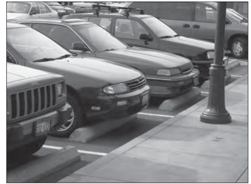
Tire bumpers keep cars from encroaching onto sidewalk.
