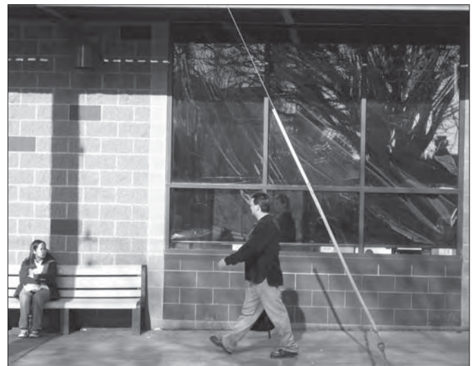
Impeding window transparency disconnects building use from the street, deadening the pedestrian environment and may be a code violation.
