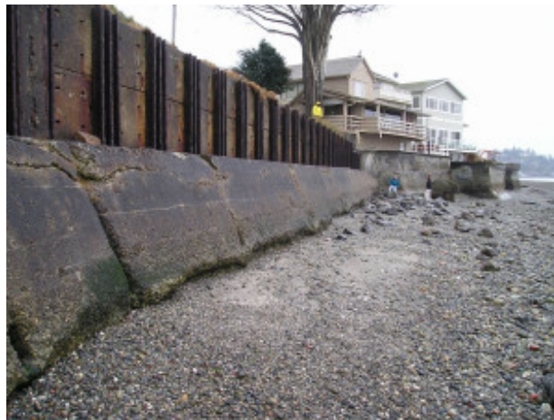
Existing Alki Seawall, Seattle, Washington
