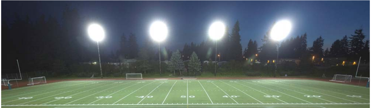
Shielded, Aimable Metal Halide Floodlight System 2015
