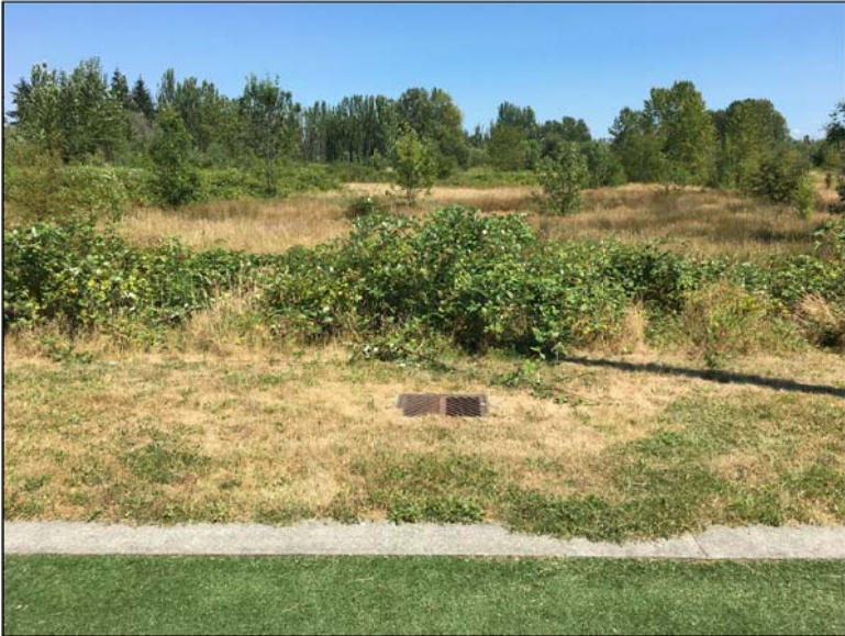
Typical drainage infrastructure associated with Fields 6 and 7, this catch basin is actually a cleanout / control structure, from which the piped storm water is discharged to a created wetland.
