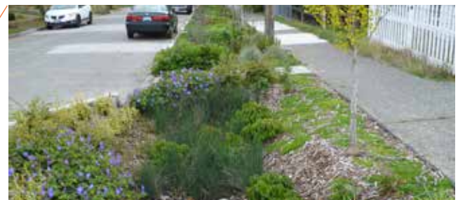
Ninety-one roadside bioretention cells capture runoff from the road in the Sunrise Heights and Westwood neighborhoods
