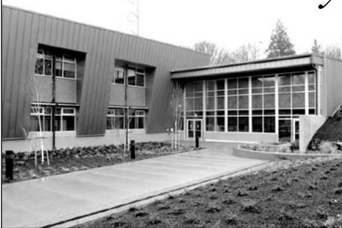
The south-facing facade of the Seattle Police Department's Southwest Precinct features a canted wall and overhang to provide sun protection at the second floor, and exterior sunscreens above the first floor windows.
