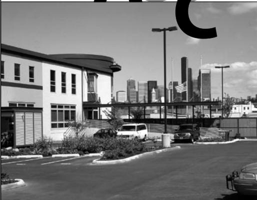
*The asphalt parking lot at Park 90-5, a multifunction police support facility, was at the end of its life and required replacement. It was pulverized on site and reused as base material under the new asphalt surface.*
