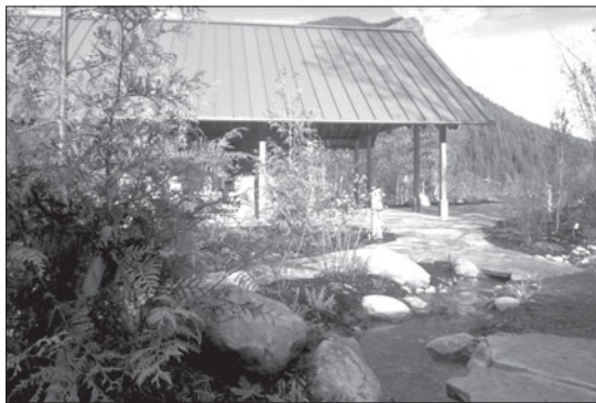
A constructed stream collects the surface drainage and roof water. Drainage from the parking areas is channeled into bioswales planted with wetland shrubs that slow and purify the water.
