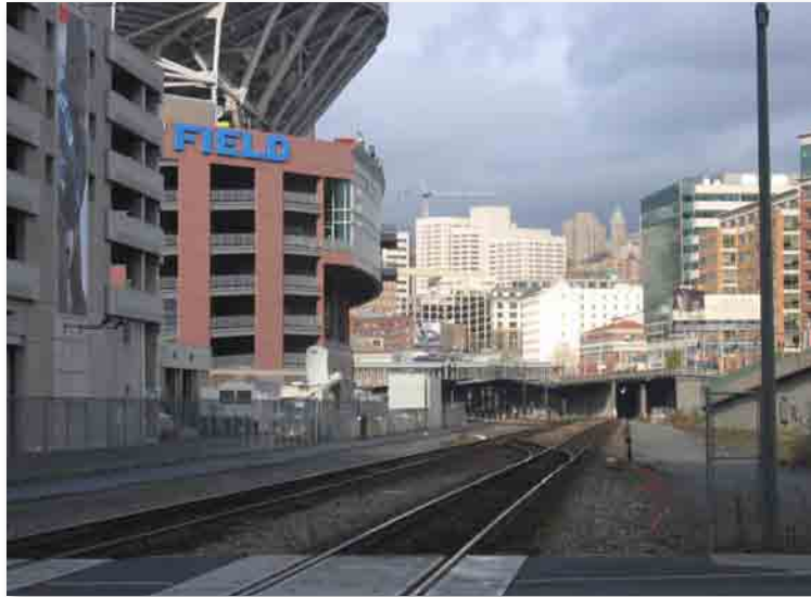
Rail crossing at S. Royal Brougham Way
