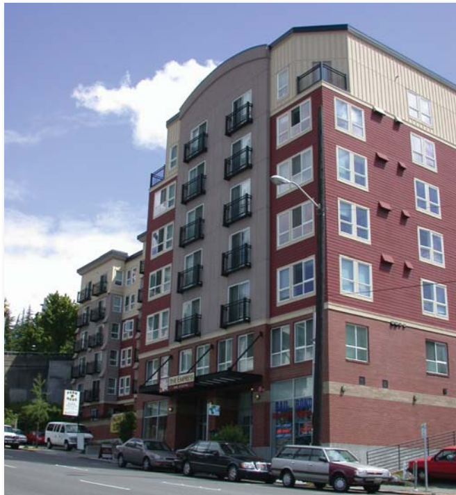
Careful infill: Empress Apartments on Fifth Avenue S.
