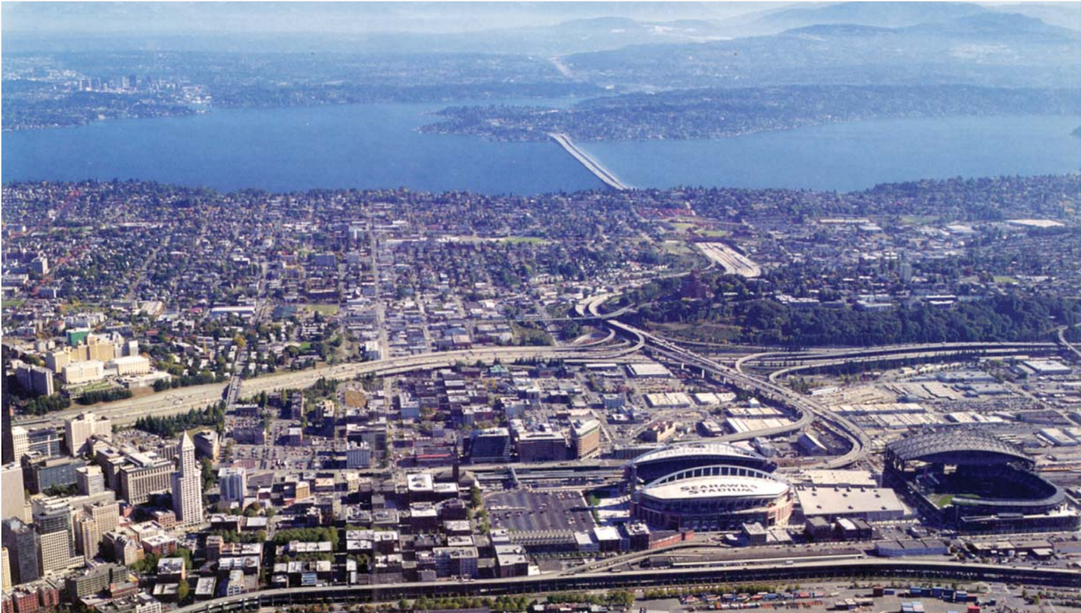
South Downtown, view from the west
