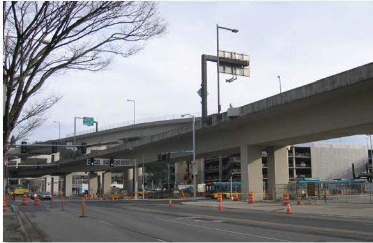
View of I-90 ramps from South-of-Dearborn Area
