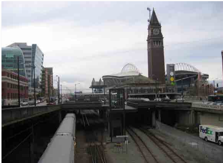
Railyard below street grade near S. Jackson Street
