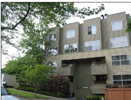
Apartment building (Greenwood Avenue North and North 76 th Street). Streetfront setbacks, landscaping, and building modulation make this one of the better multifamily building examples in the neighborhood.
