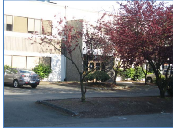
Figure 27: West side of Alpha Cine building
