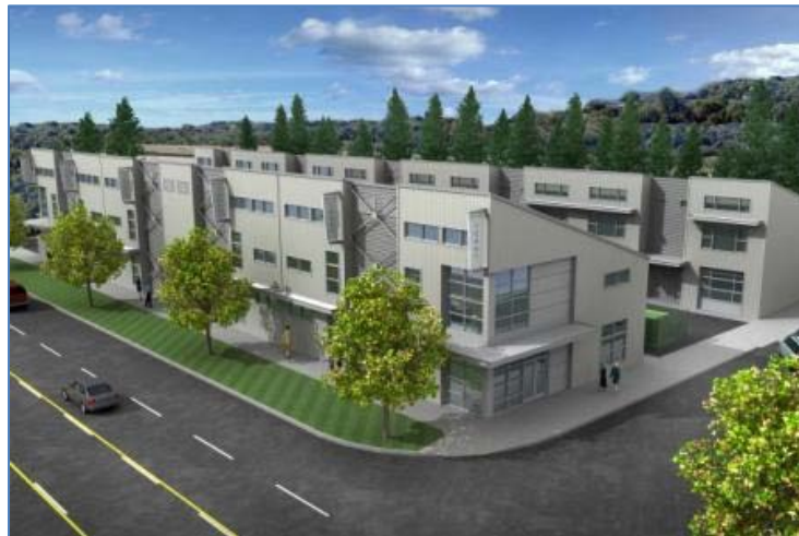
Figure 28: Holgate Square, proposed SoDo flex space development. Note the 20' clear height, small unit division, and loading interior to the site. 155
