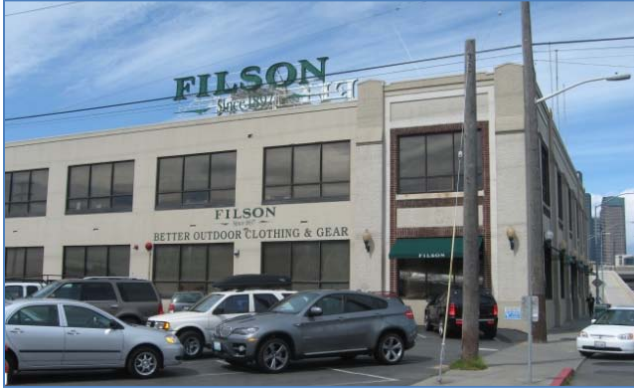
Figure 99: The 38,000-square-foot Filson factory and retail store, 1555 4th Avenue South 388
