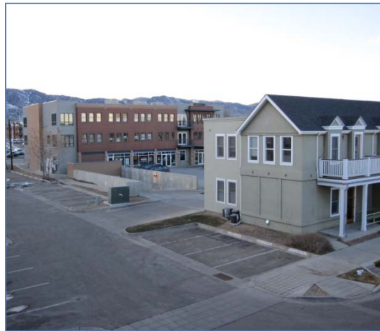
Figure 67: View from 2nd story industrial unit of housing (right foreground) and retail/office (left rear). Note that the retail building separates the housing from arterial traffic.
