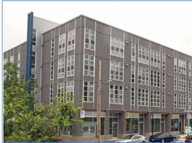
Figure 36: Artspace Hiawatha Lofts. 178 Spaces are available for live/work studios and retail.
