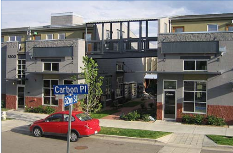
Figure 73: Industrial units at the Steel Yards 283
