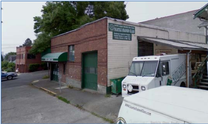
Figure 98: Seattle Stained Glass rear view. Note use of vans for delivery, high ceilings, covered loading, and multiple rollup doors. 379
