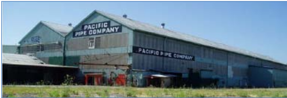
Figure 91: Existing Pacific Pipe Company building 325
