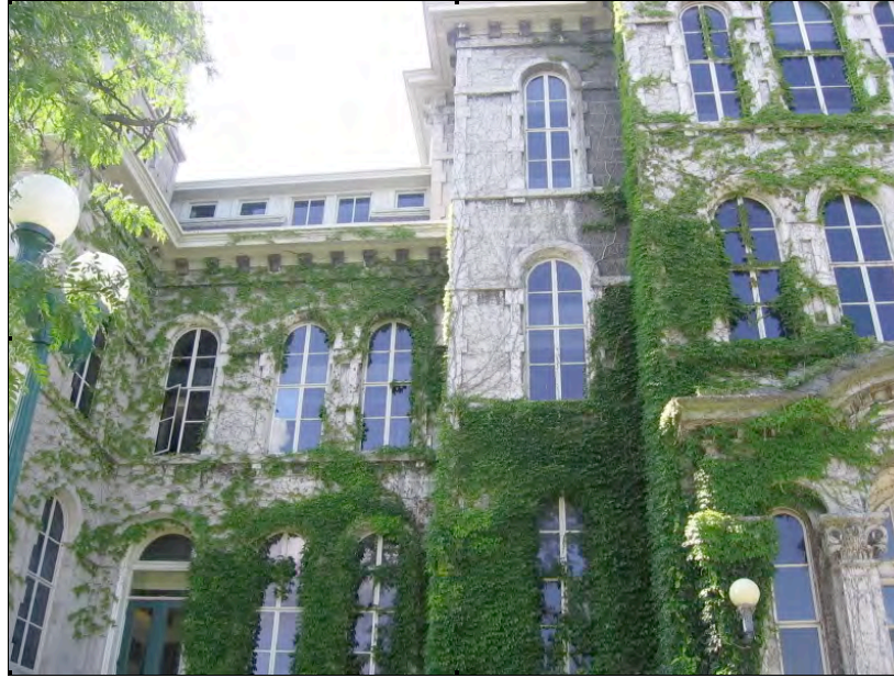
This late nineteenth century four-story building was renovated to insert an extra floor, visible as a wide band across the second story windows, above.
