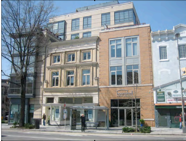
Buildings to the left, right, and above the center building are additions.
