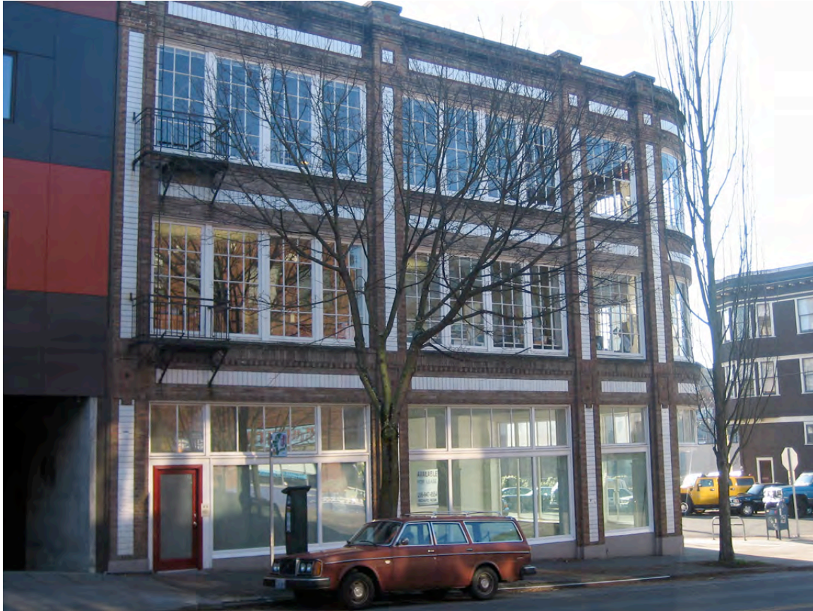
Solid frame construction and expansive windows give a solid, yet light and transparent appearance to neighborhood character buildings.
