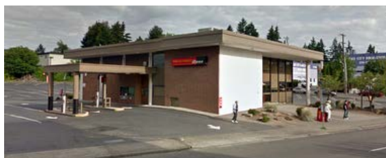
Small buildings surrounded by large parking lots are allowed in C1 but prohibited for new buildings in NC3 zones.
