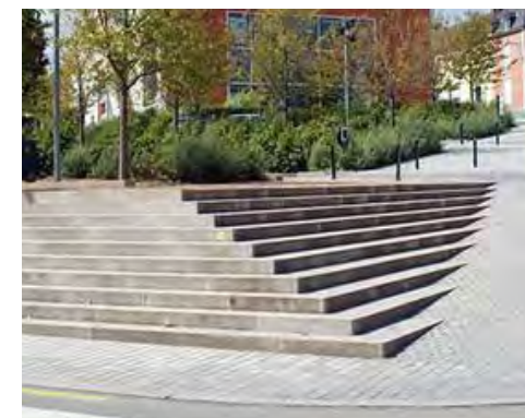
CIP Concrete Stair
