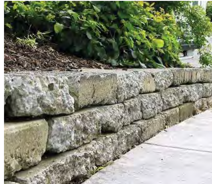
Salvaged Concrete Rubble Wall
