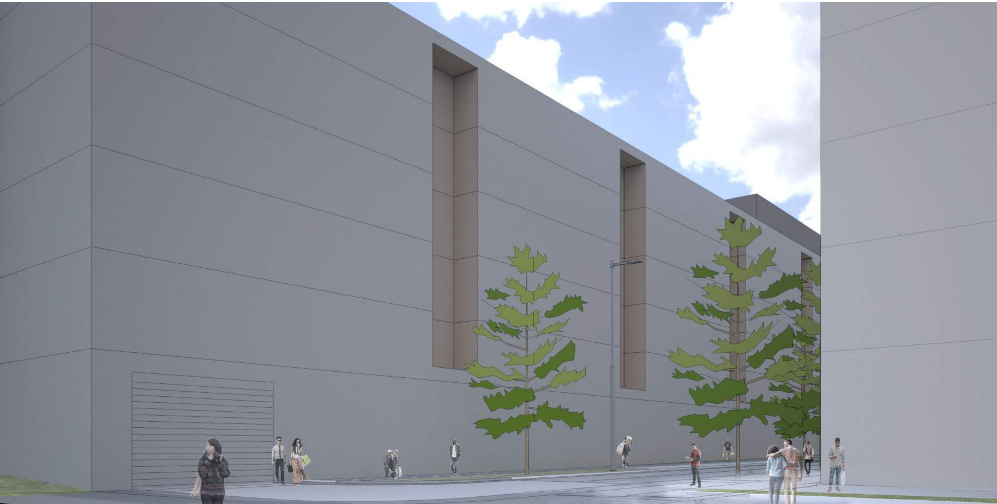
View looking North along 24th Ave
