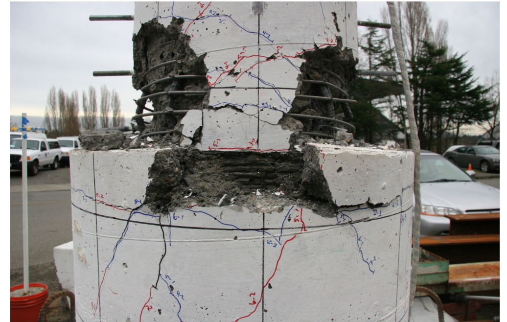
Figure 89. Photos. Specimen DS-1 column damage after cyclic testing.
