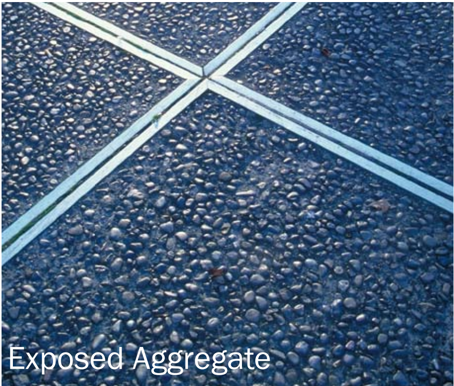
Entry Court and South Terraces: Texture and Functionality
