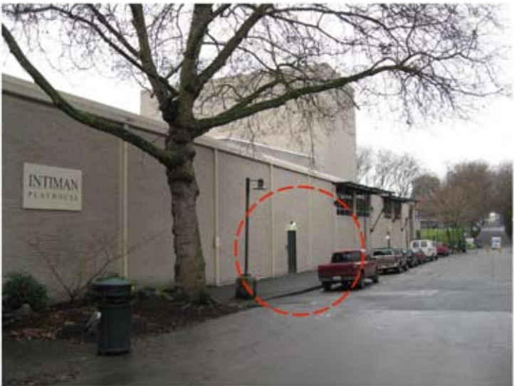
15 EXISTING CONDITION PHOTO - EXISTING ENTRY A103 SCALE: NTS
