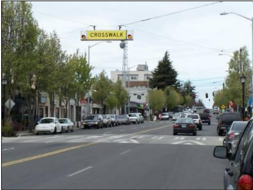
Arterial Traffic Calming in West Seattle
