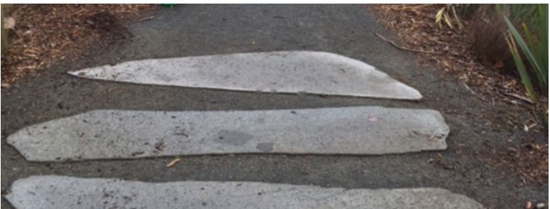
AGGREGATE PATH WITH STONE SLAB PAVERS
