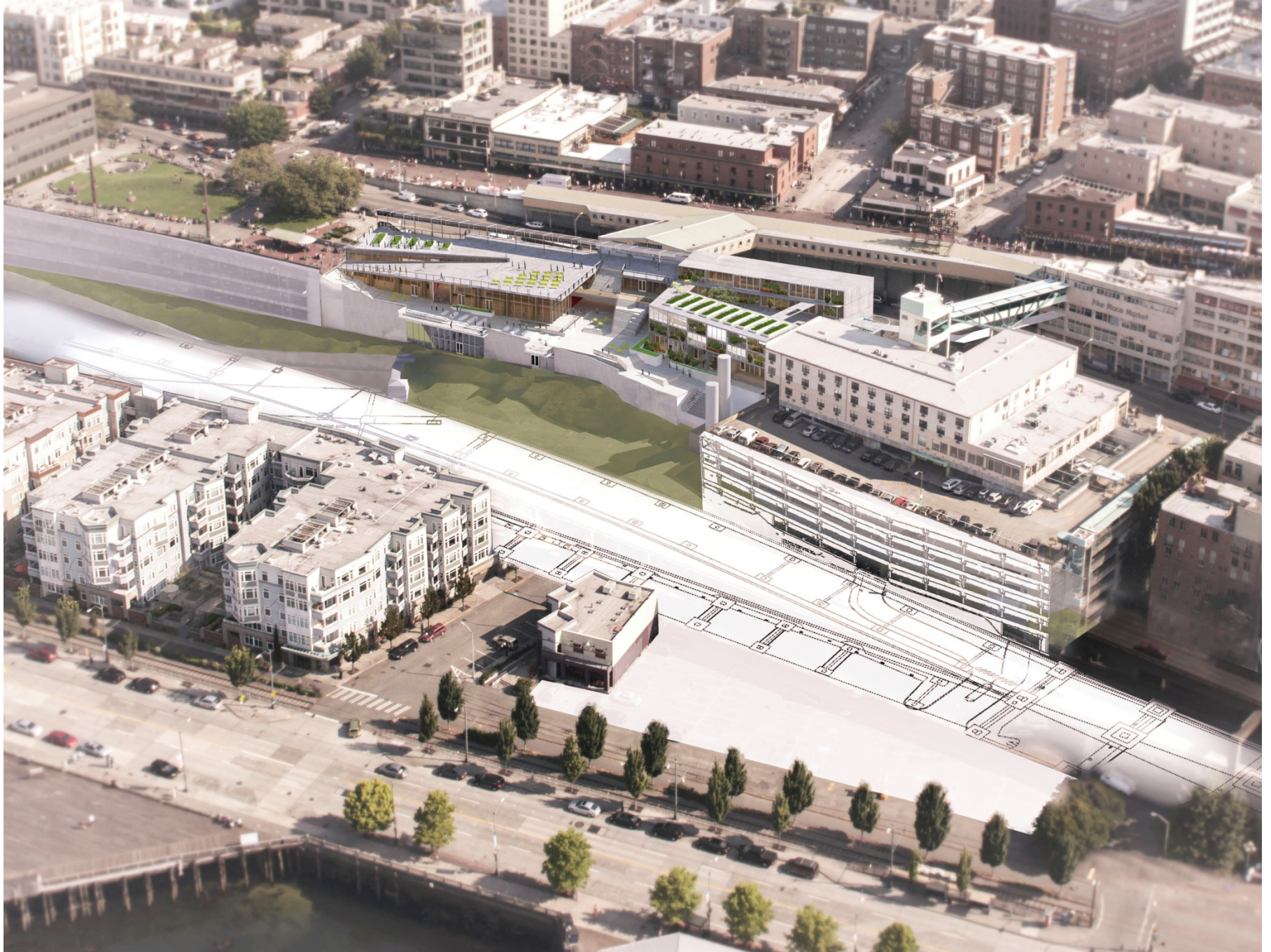
January 2016 – Demolition of Viaduct begins
