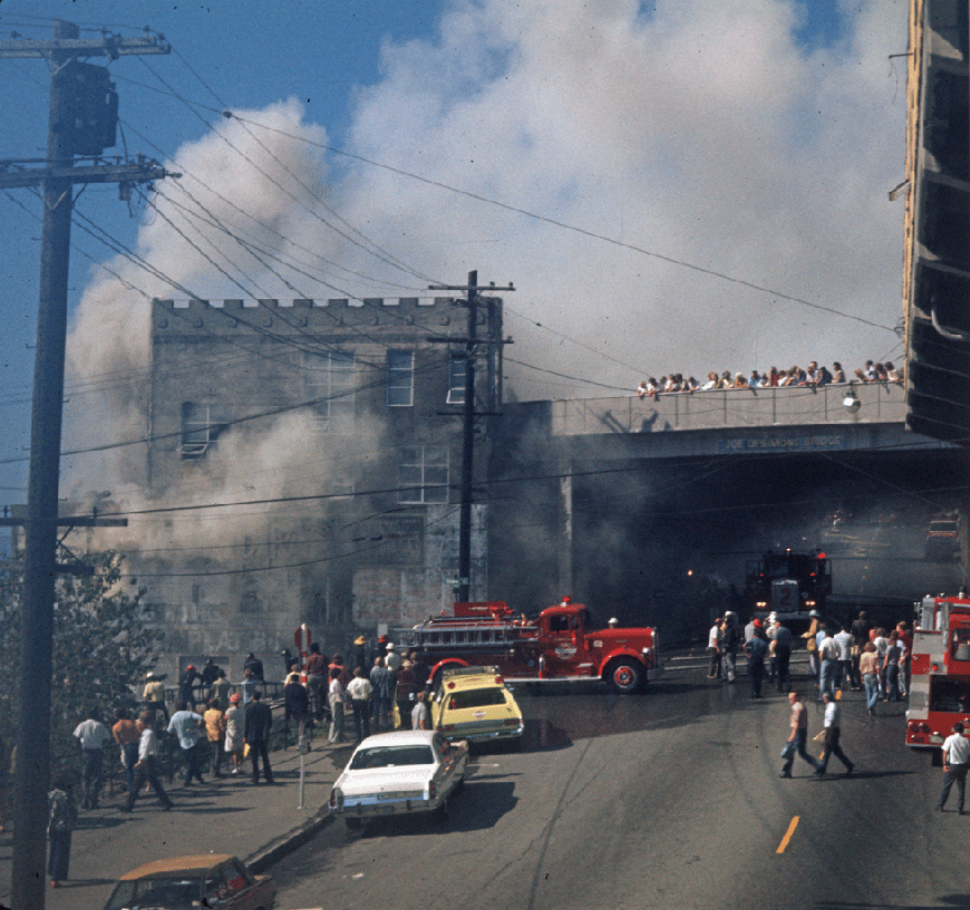
1974 – Fire in Municipal Market Building
