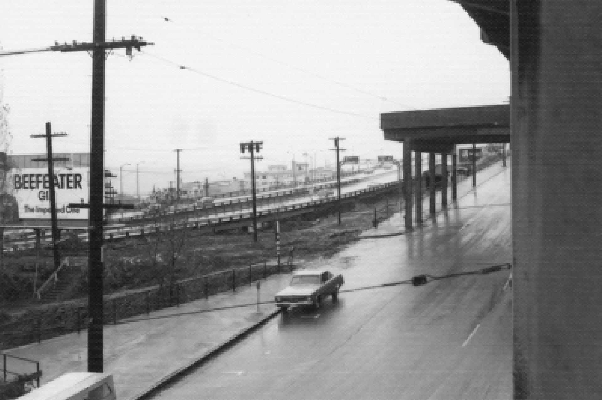
1974 – Cleared and Graded site
