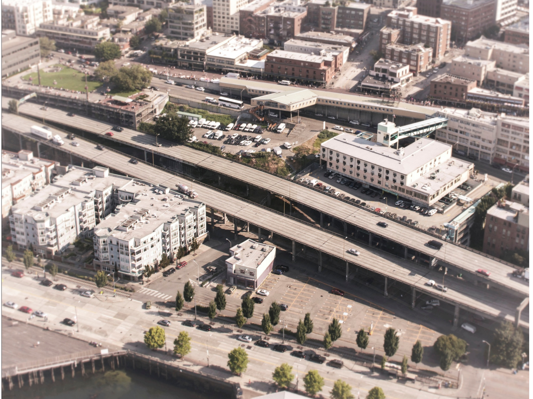
Summer 2014 – Construction Begins
