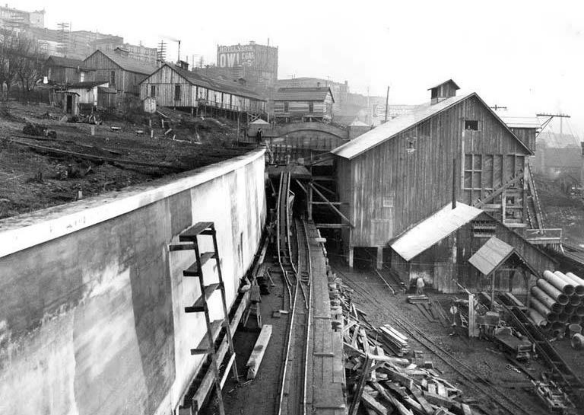
1904 (est) – Tunnel Construction (UW)
