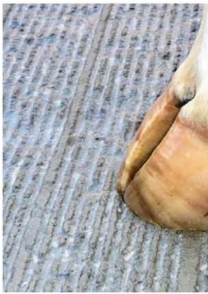
MACHINE GROUND GROOVES
