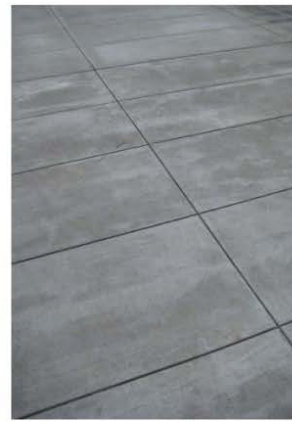
CAST IN PLACE CONCRETE
