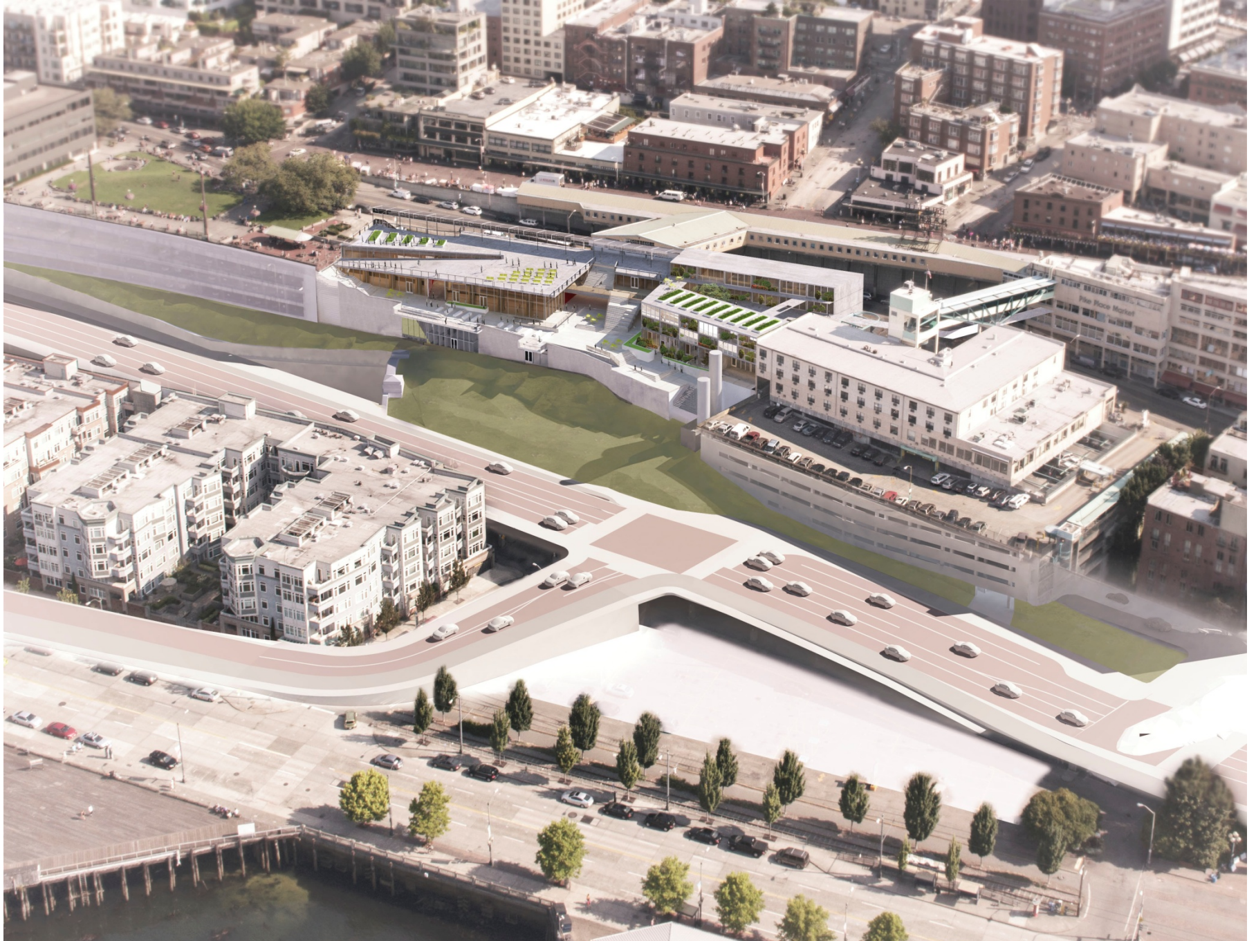
2017 – Construction of Elliott Way Connector Road
