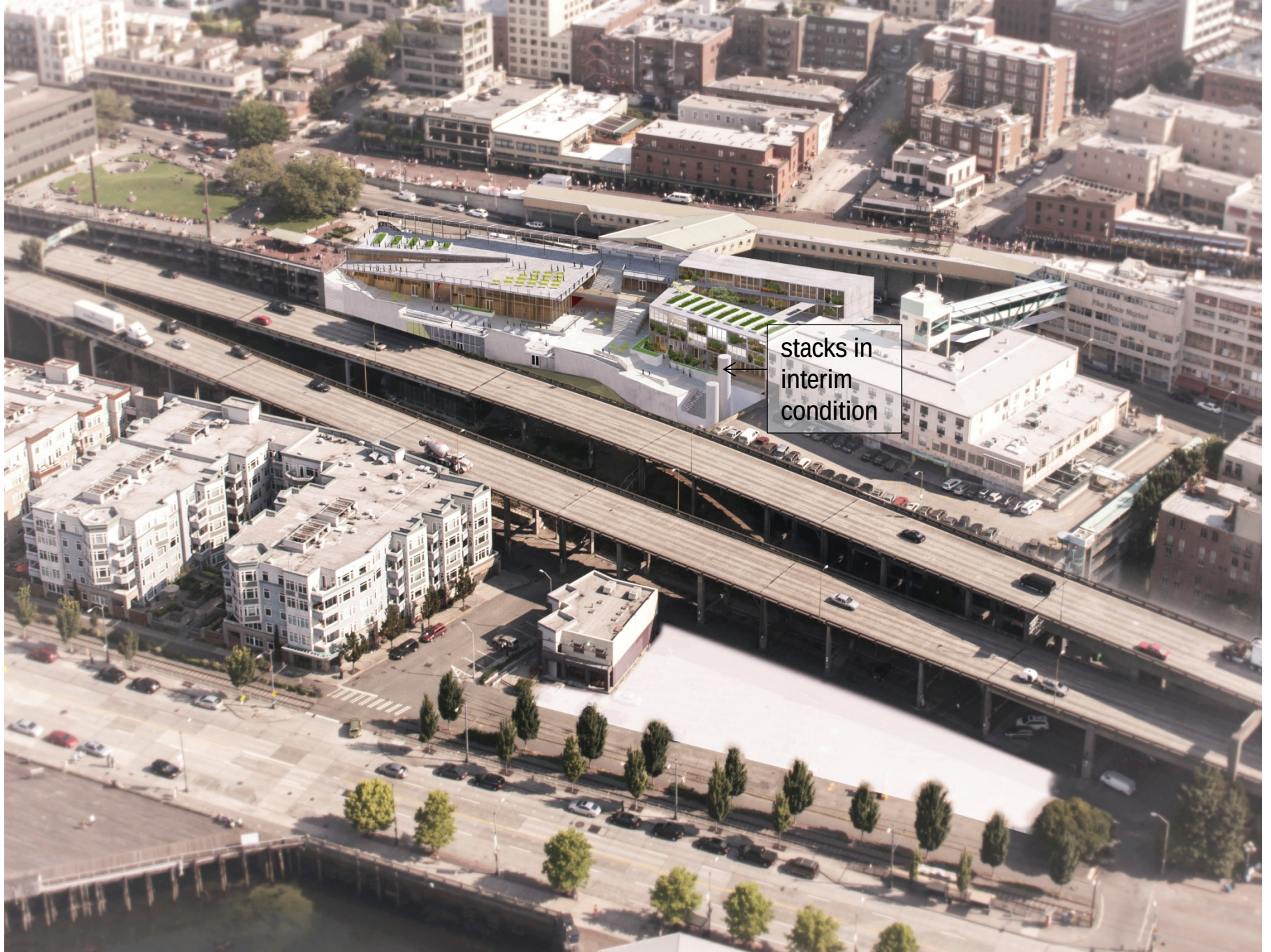
December 2015 – Construction Complete
