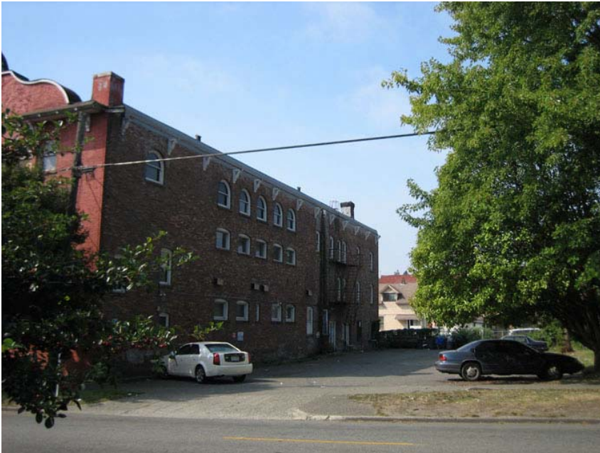
Washington Hall, 2007, view of north wall. (Photo by applicant)
