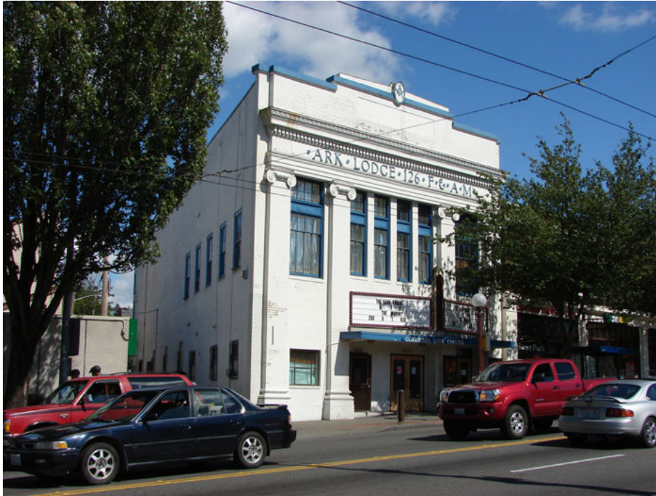
Ark Masonic Temple Lodge, 2008, view of northwest corner looking southeast. (Photo by applicant)
