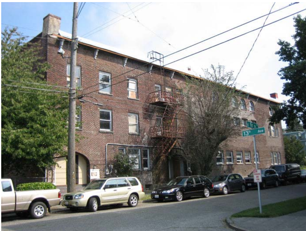
Washington Hall, 2007, view of Fir Street wall. (Photo by applicant)
