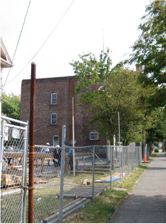
Washington Hall, 2007, view of west wall. (Photo by applicant)
