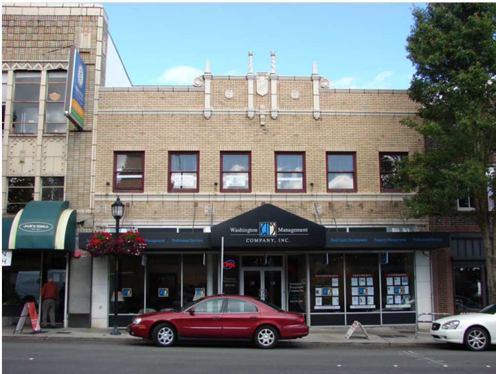
1929 Bartell Drugs Store (now Washington Management Co. building), 2008, view of west façade looking east. (Photo by applicant)
