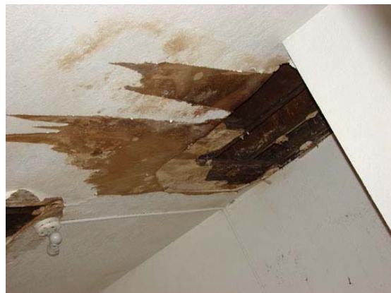
Washington Hall, 2007, view of damaged ceiling in 3 rd floor boarding room. (Photo by applicant)
