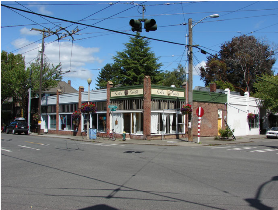
1924 Benjamin Franklin Thrift Market (now Café Soleil), 2008, view of southwest corner looking northeast. (Photo by applicant)
