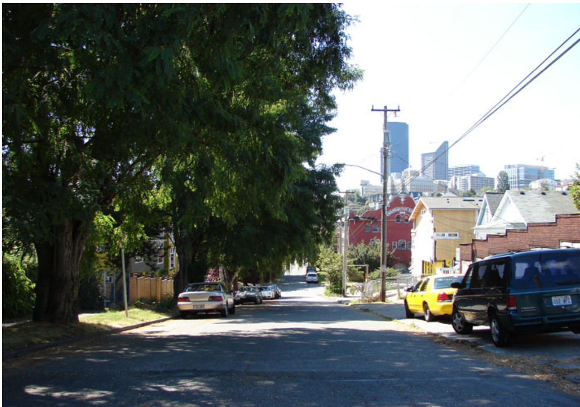
View of Washington Hall from intersection of 15 th Avenue and E Fir Street. Looking west. (Photo by applicant.)
