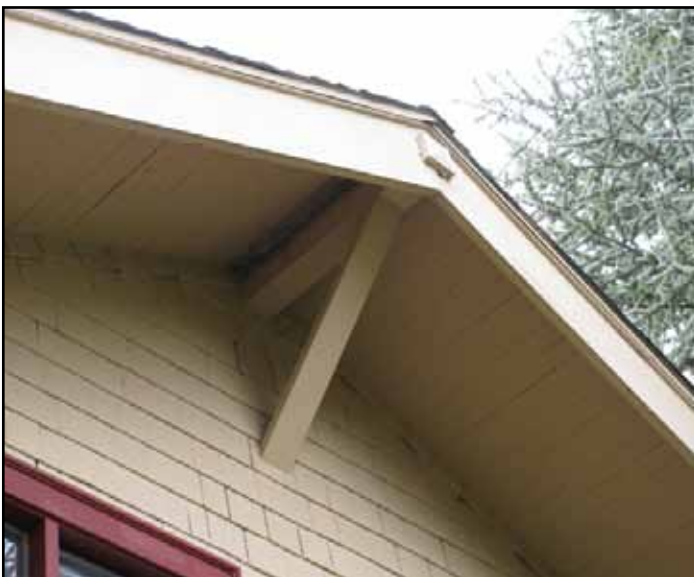
Left: 2010. Detail view of of triangular knee brace under eave. Right: 2010. View of notched ends of vergeboards at northeast corner of house. Note original pointed square block detail at end of triangular knee brace in both photos. Source: Historic Seattle
