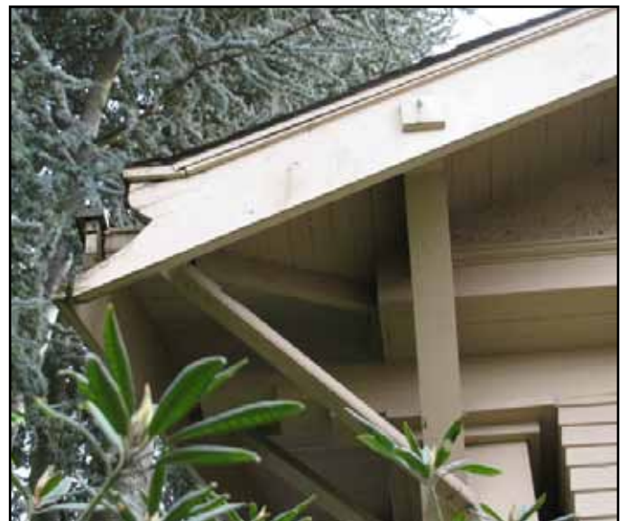
Left: 2010. Detail view of of triangular knee brace under eave. Right: 2010. View of notched ends of vergeboards at northeast corner of house. Note original pointed square block detail at end of triangular knee brace in both photos. Source: Historic Seattle
