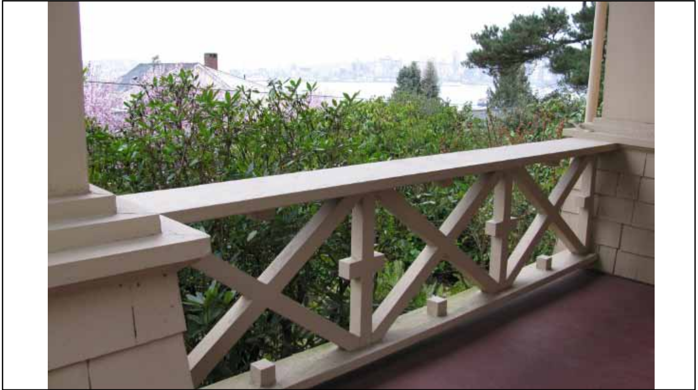
2010. Historic wood railing on front porch, facing northeast. Source: Historic Seattle
