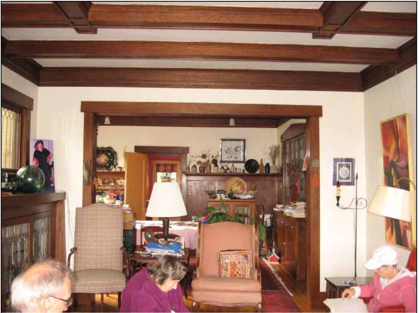
2009. View from living room looking west into dining room. Original features intact include: box beams, built-in bookcase, buffet, wainscot, molding, oak floor, picture rail, baseboards, plaster walls and ceiling, and ceiling lights in dining room. Woodwork is mahogany. Bloss House owner Ruth Ward in center sitting with friends Jim and Sharon Price. Source: Historic Seattle
