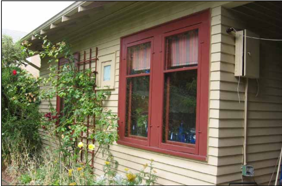
2009. View of rear (south) facade, facing northwest. Note rafter ends under eave and original one-over-one, double-hung, wood sash windows (with wood storm windows). Source: Historic Seattle
