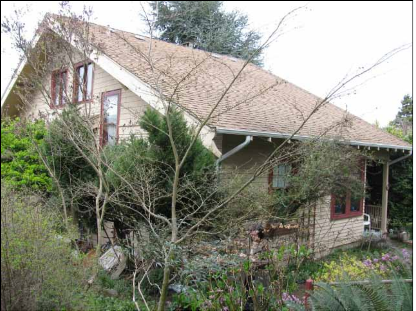
2010. View of west (side) and south (rear) facades, facing northeast. Note rafter ends on south facade and rear porch at southeast corner. Source: Historic Seattle
