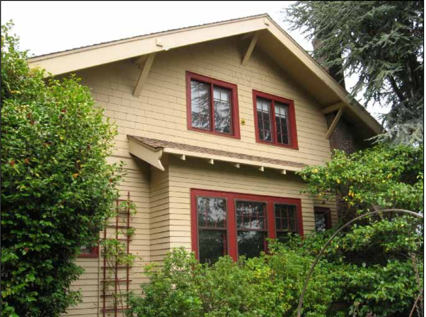
2009. View of east facade, facing northwest. Square window bay features a cluster of three, original, double-hung-wood sash windows (with contemporary storm windows). Bay has a shed roof with notched vergeboard end and rafter ends. Original casement windows provide light into the upper half-story. Source: Historic Seattle
