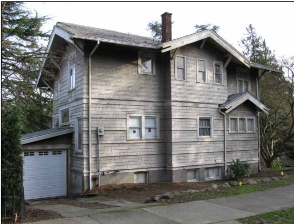
2010. Elmer E. Green-designed house at 2540 34th Ave S in Mount Baker. Garage added. Built in 1912, the property is included in DON's Historic Sites Inventory database. Source: Historic Seattle.
