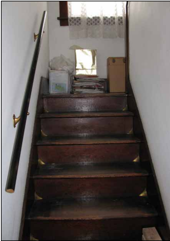
2010. Original wood stairs from hallway to upper-half story, facing west. Note metal, corner dust catchers. Source: Historic Seattle
