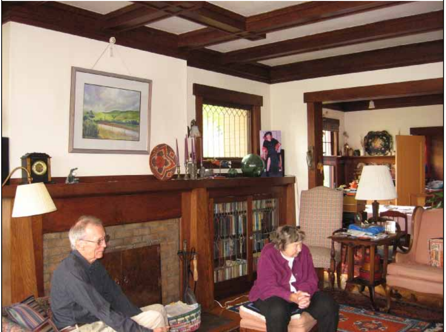
2009. View of living room east wall looking southeast. Dining room on right. Original fireplace and built-in bookcase with leaded glass doors share a wood mantelshelf. Leaded glass window is above the bookcase. Bloss House owner Ruth Ward on right sitting with friend Jim Price. Source: Historic Seattle
