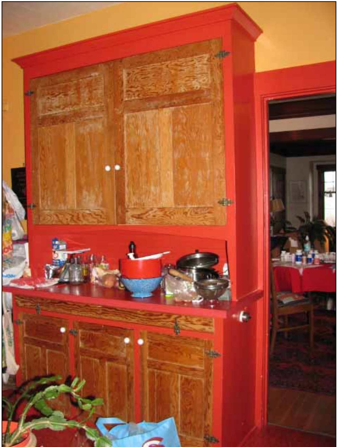
2010. View of original, wood kitchen cabinets, facing northwest. Original ironing board hidden between countertop and lower cabinets. Countertop and vinyl floor installed in the 1970s. Source: Historic Seattle
