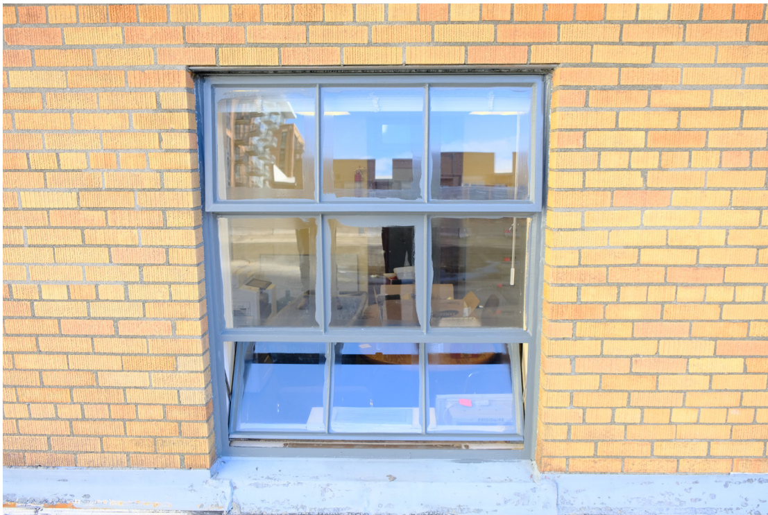
ORIGINAL WINDOW ON NORTH FACADE RESTORED
