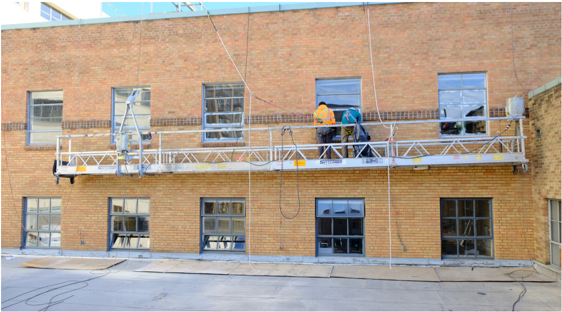
ORIGINAL WINDOW RESTORATION IN PROCESS ON NORTH FACADE
