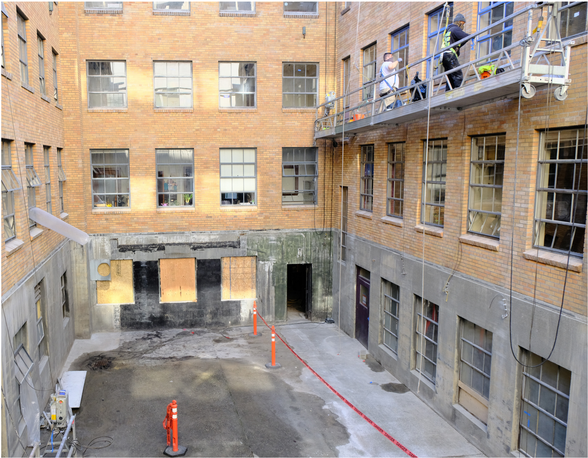
ORIGINAL WINDOW RESTORATION IN PROCESS AT THE COURTYARD FACADES
