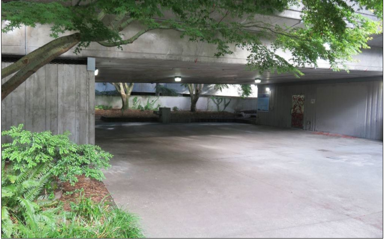
Photo 14. Freeway Park as it passes under the 8th Ave. overpass, with maintenance sheds on either side of the breezeway, view northeast.
