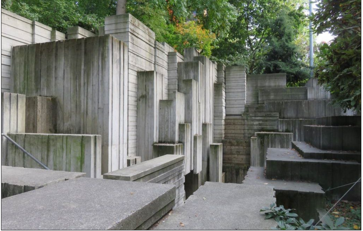
Photo 11. Interior of Freeway Park Canyon, view southeast (waterfall temporarily inactive).
