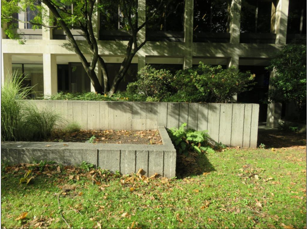
Photo 7. The Park Place Plaza (1971) where it connects to Freeway Park (1976). Seams in the concrete are minimally visible.
