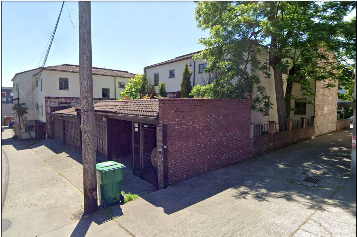
Fig. 11 – East and north elevations from alley. (Google Streetview, 2019)
