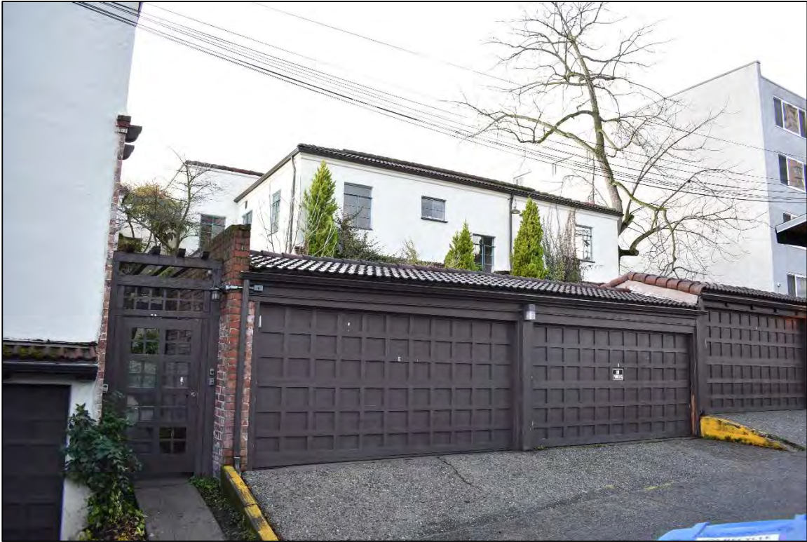
Fig. 10 – East elevation of garage from alley.
