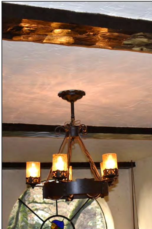
Fig. 35 - (Four photos) Interior, typical unit details. All include wall niches, built-in cabinets, hand-adzed ceiling beams, period light fixtures and door hardware.
