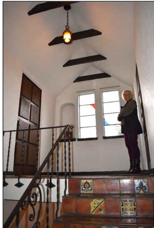
Fig. 22 - (Four photos) Interior, main stairwells (typical), showing variety of decorative glazed tile. Photo at lower right shows third floor landing at southwest building mass; visible are exposed beams, wall niche, leaded stained glass. There are two unit doors at each landing.
