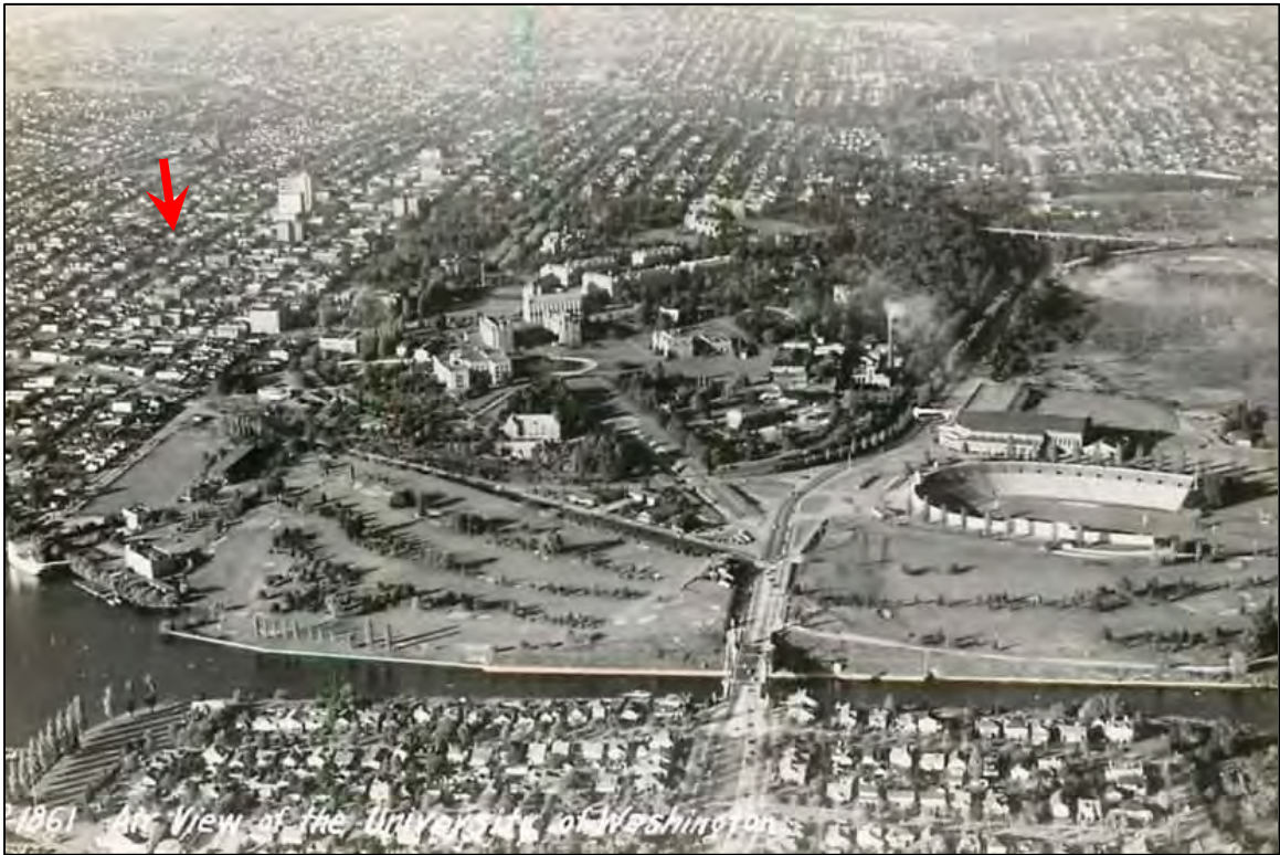
Fig. 47 - Circa 1940 northward view of the University of Washington. University District visible at left. Arrow indicates approximate location of subject building. (Paul Dorpat)
