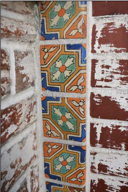
Fig. 15 - (Two photos) South elevation, detail showing decorative glazed tiles and metal window screens.
