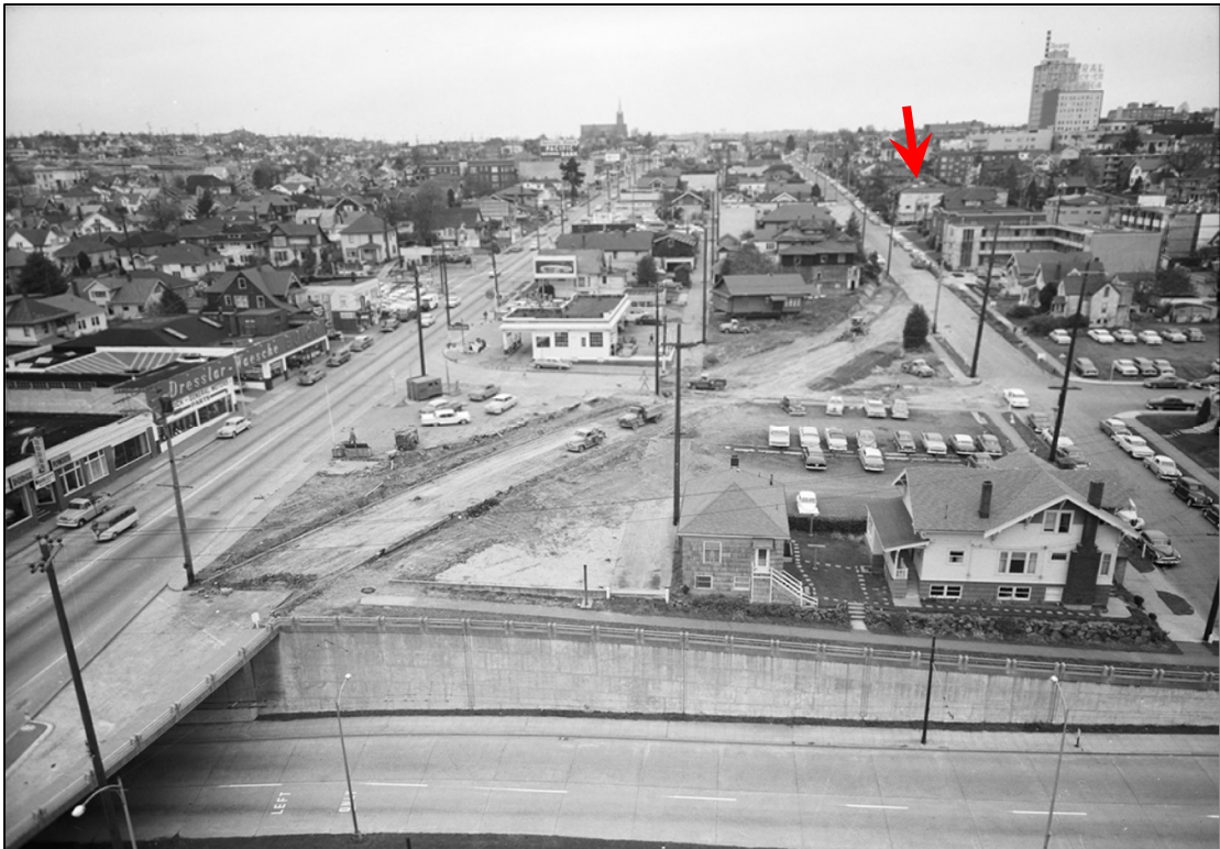
Fig. 46 - 1959 view northward of Roosevelt and 11 th Avenues, being converted to twinned one-way arterials. Campus Parkway in foreground, with retaining wall. Subject property indicated by arrow. (SMA #62966)
