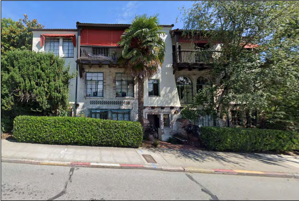
Fig. 12 – West elevation, south part, from 11 th Avenue NE. (Google Streetview, 2019)
