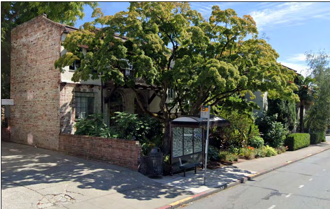
Fig. 13 – North and west elevations from 11 th Avenue NE. (Google Streetview, 2019)
