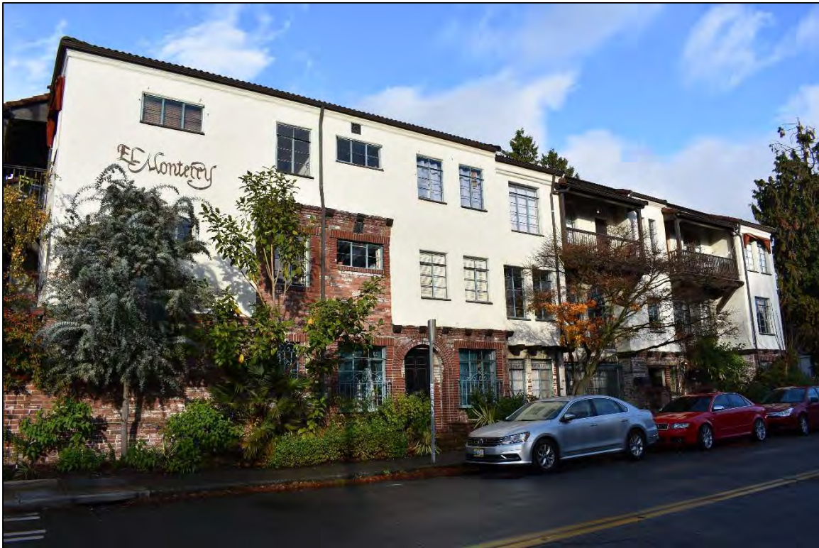
Fig. 8 – South elevation from NE 42 nd Street.
