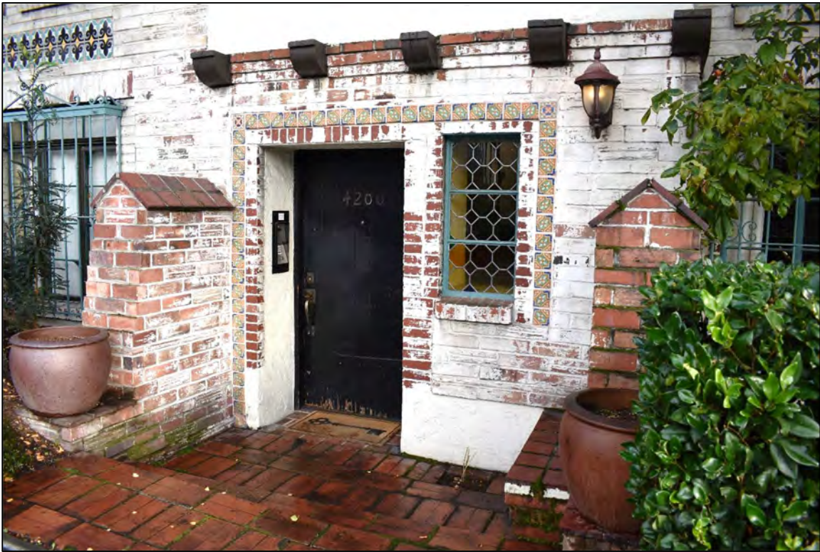
Fig. 16 – South elevation, main entry to southwest units; note glazed tile surround.
