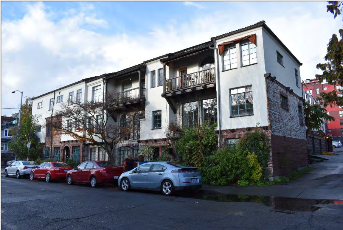
Fig. 7 – View northwest towards site from NE 42 nd Street, showing south and east elevations.
