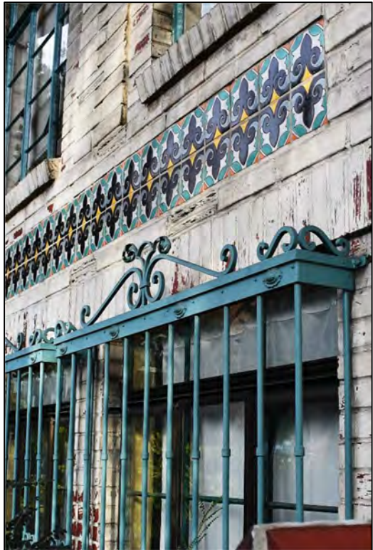
Fig. 15 - (Two photos) South elevation, detail showing decorative glazed tiles and metal window screens.
