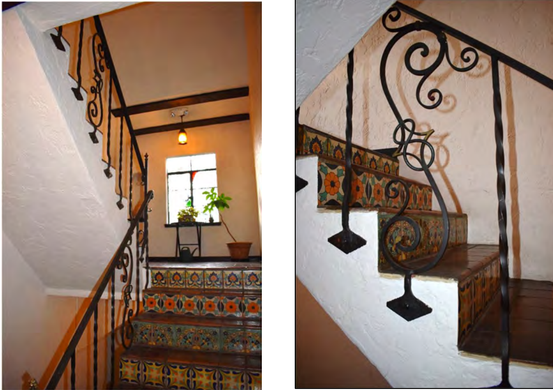
Fig. 23 - (Two photos) Interior, typical conditions at main stairwells; detail of wrought iron balustrade.
