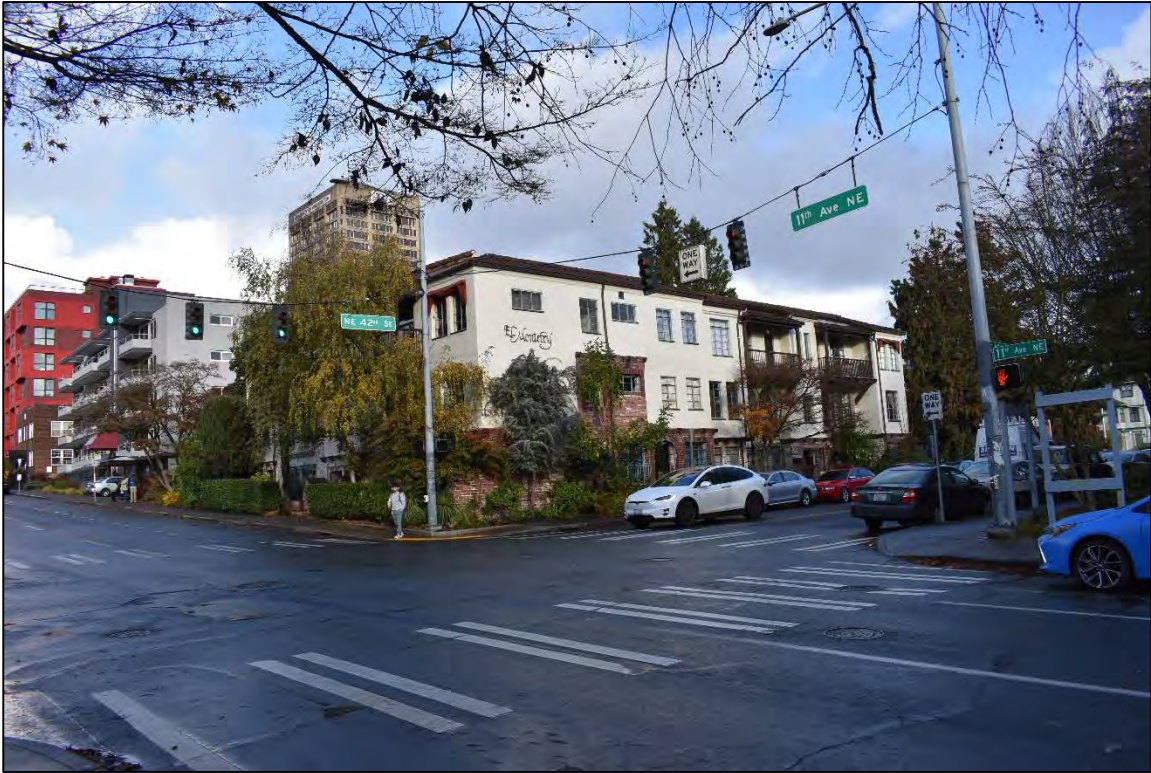
Fig. 6 – Context: View northeast towards site.
