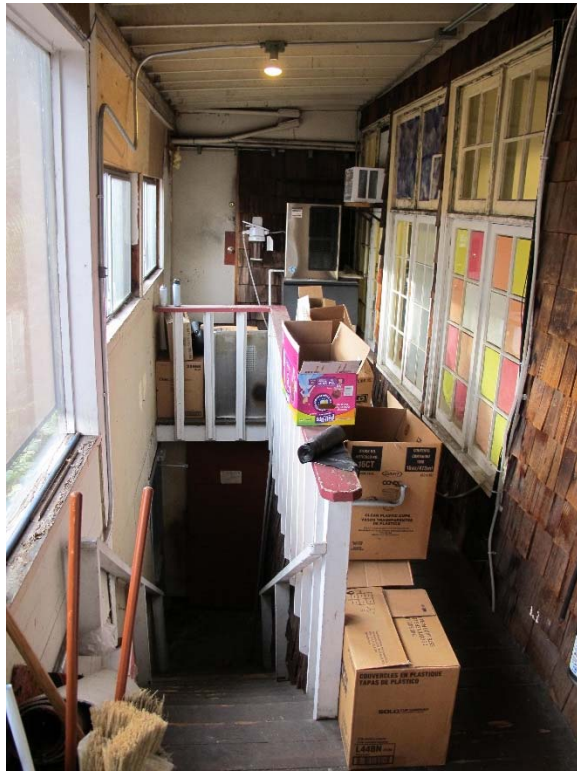
Fig. 77 – Interior main level, enclosed rear exterior stair behind concessions room storage area.
