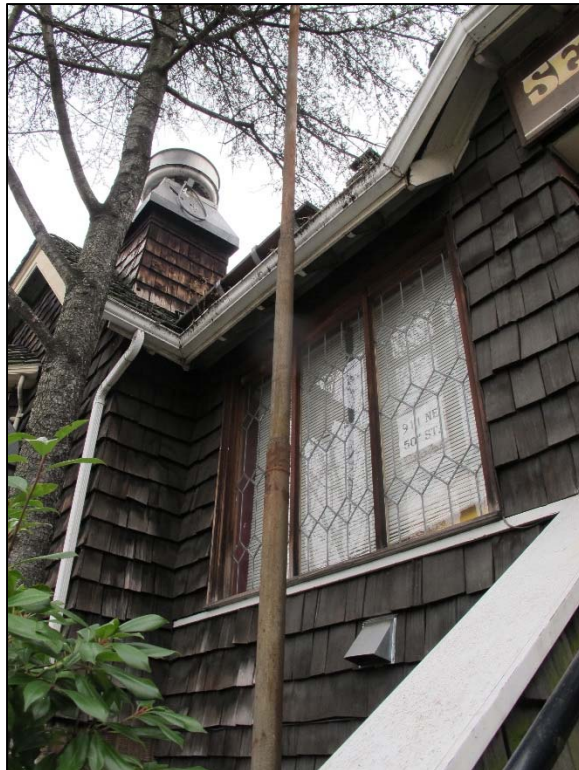
Fig. 35 – North elevation, detail of leaded window on left side of entry porch
