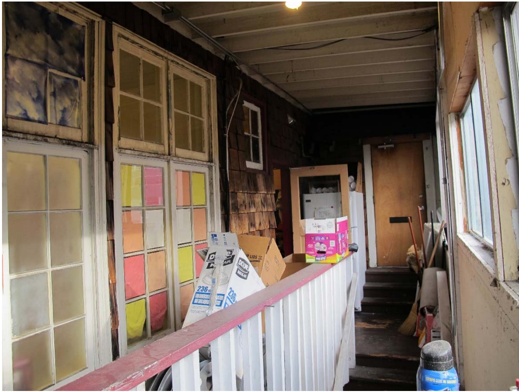
Fig. 78 – Interior main level, enclosed rear exterior stair behind concessions room storage area.
