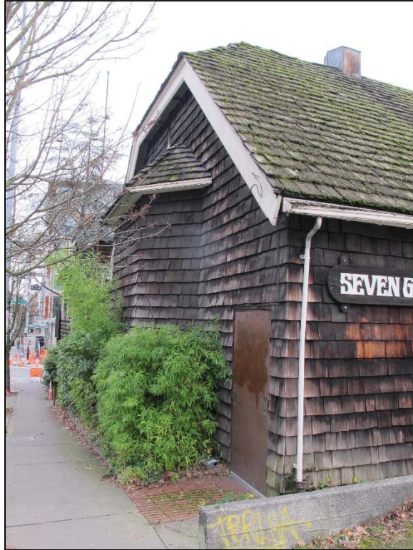
Fig. 31 – Detail, northwest building corner
