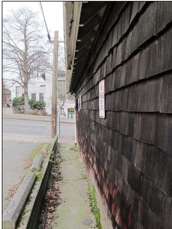
Fig. 55 – West elevation, view northwards
