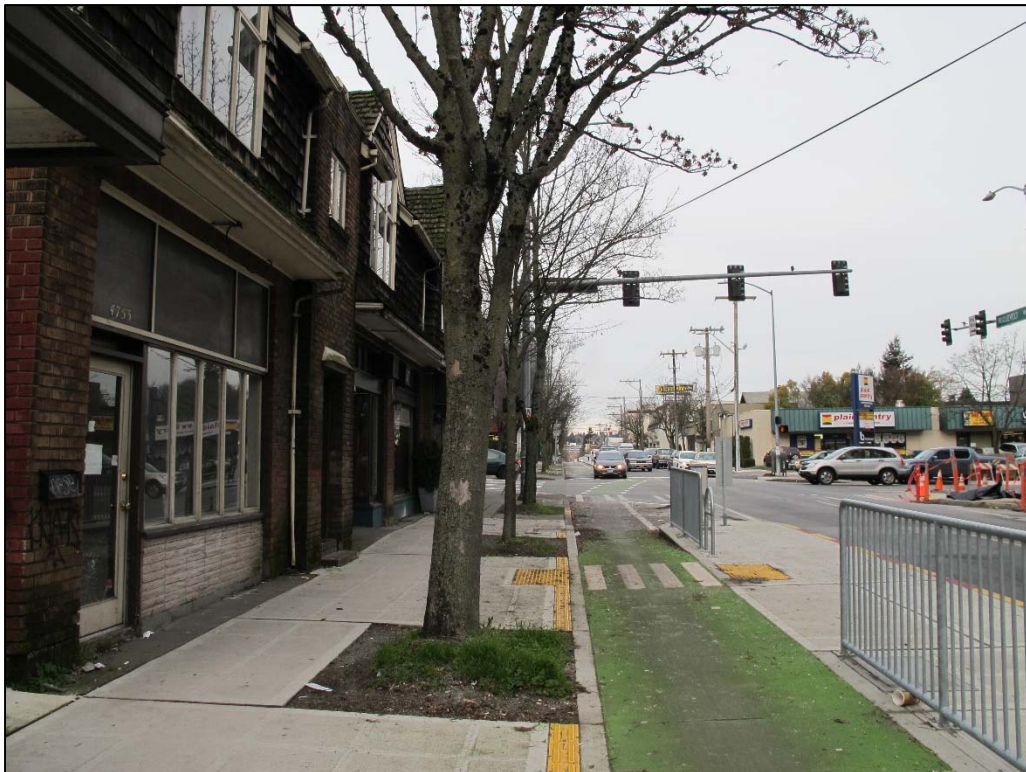
Fig. 44 – East elevation, at sidewalk
