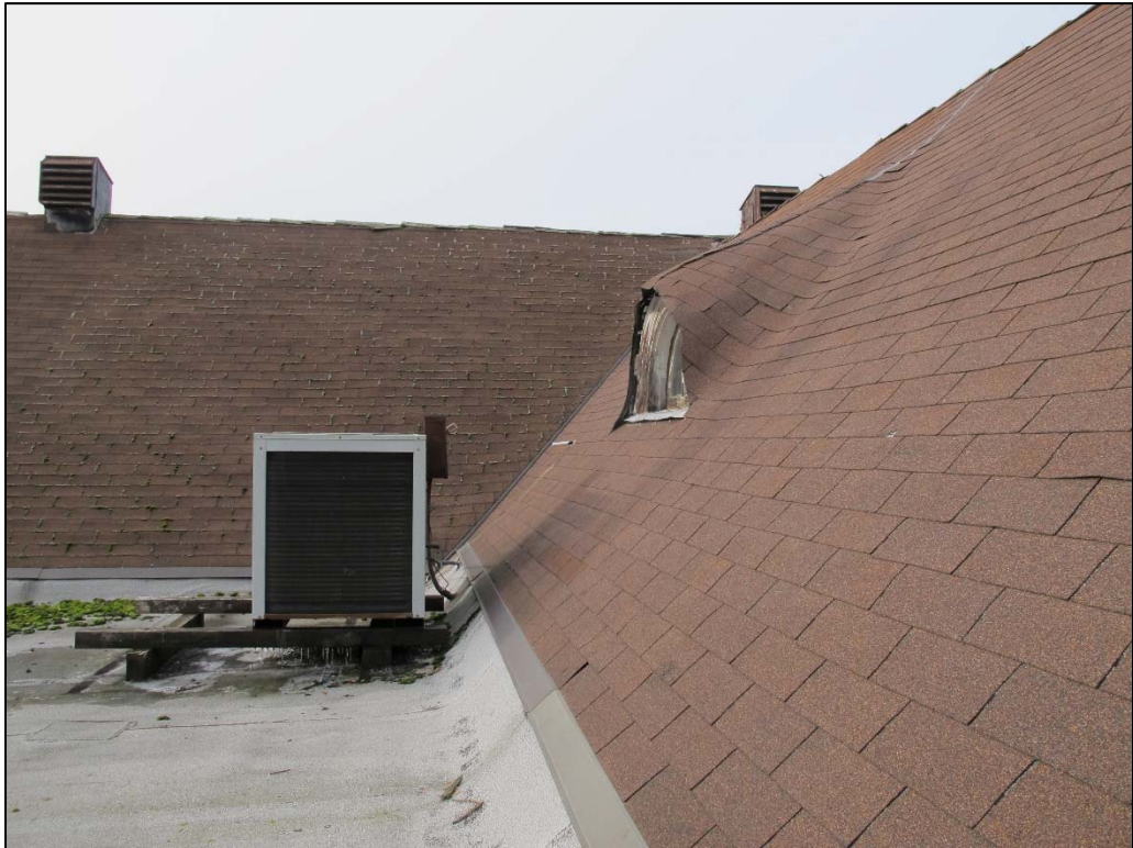
Fig. 58 – Flat roof at central south portion of building, showing eyebrow window.
