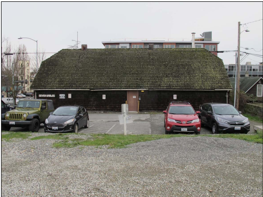
Fig. 54 – West elevation and adjacent parking lot
