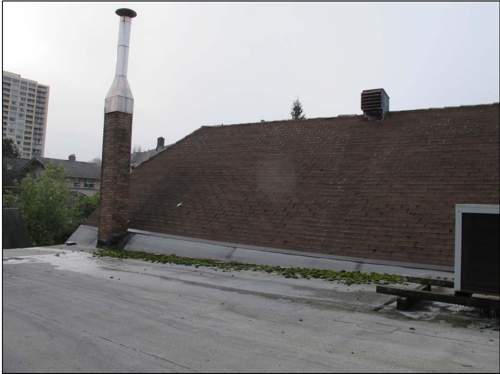
Fig. 57 – Flat roof at central south portion of building.
