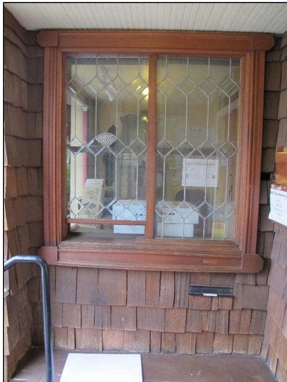
Fig. 40 – North elevation, window at east interior porch wall formerly used as ticket window
