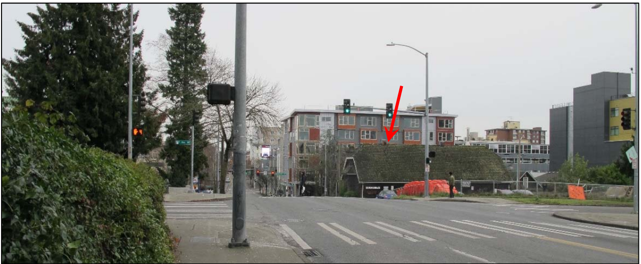
Fig. 27 – Context: View eastward on NE 50 th Street. Subject building indicated by arrow.
