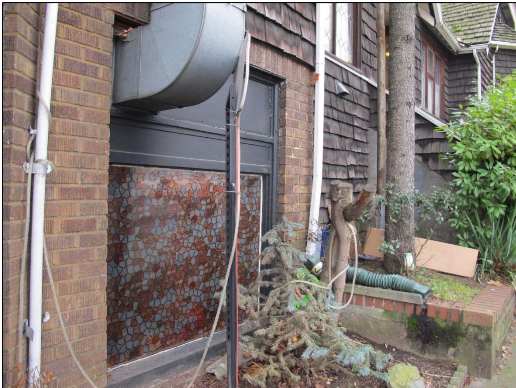
Fig. 38 – North elevation, bay window at first floor northeast corner
