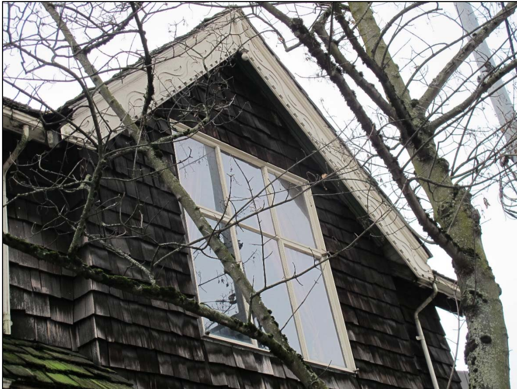
Fig. 46 – Detail, east elevation, second floor gable with decorative bargeboard
