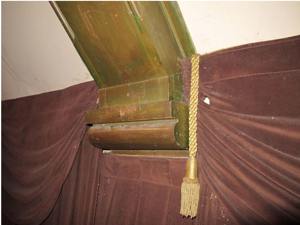
Fig. 86 – Interior main level, theater, detail of ceiling beams.
