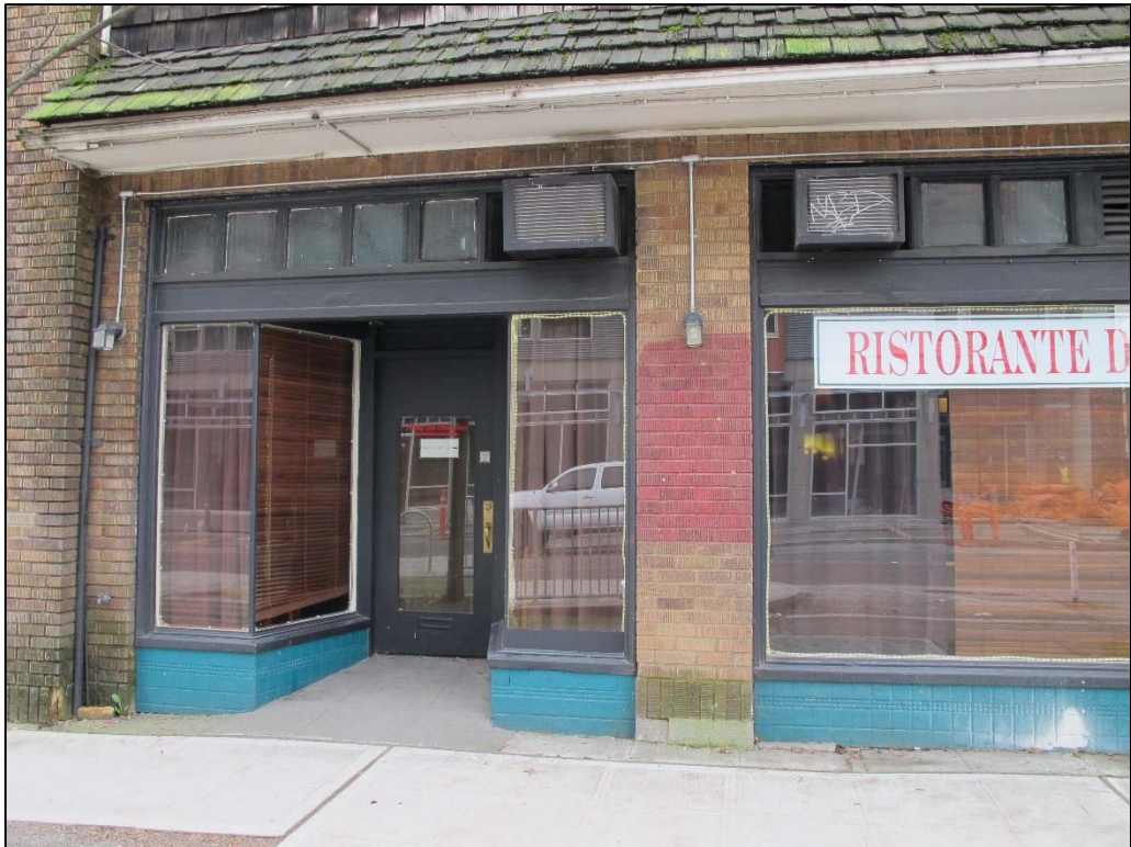
Fig. 49 – East elevation, north storefront
