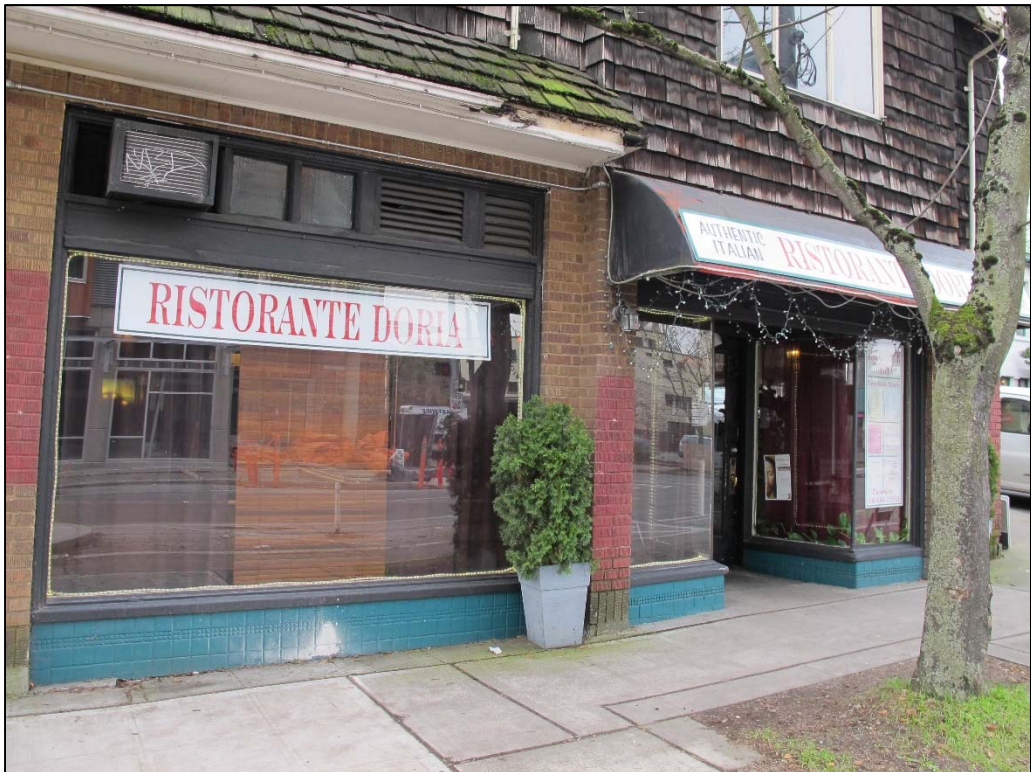
Fig. 50 – East elevation, north storefront
