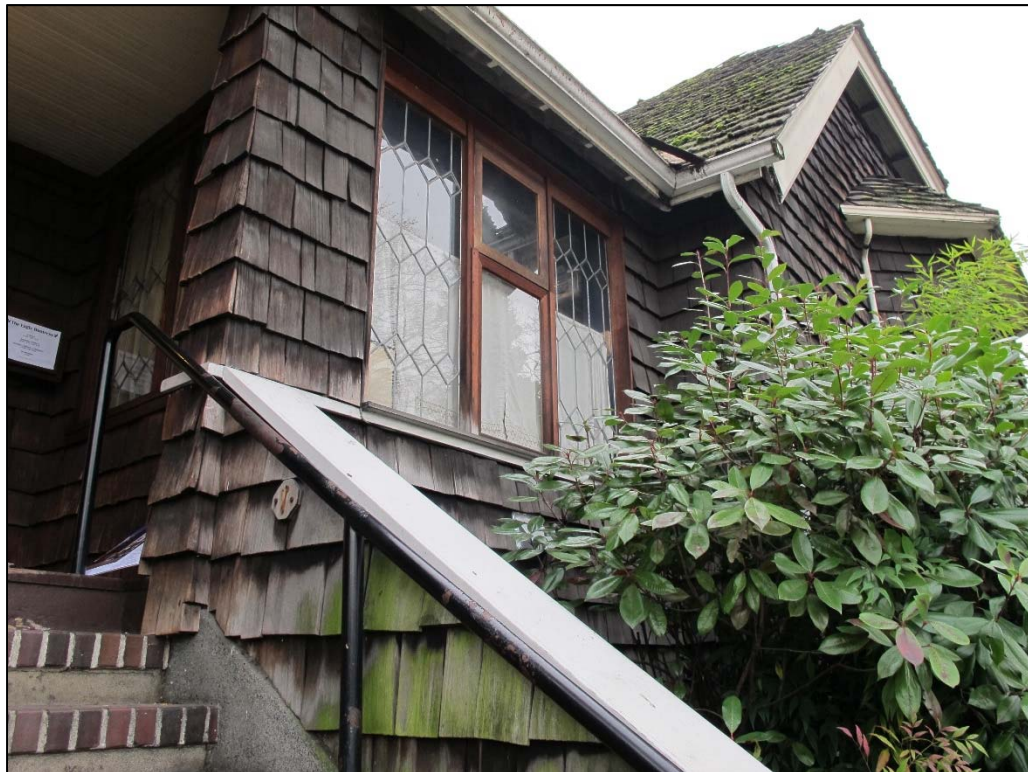
Fig. 36 – North elevation, detail of leaded window on right side of entry porch
