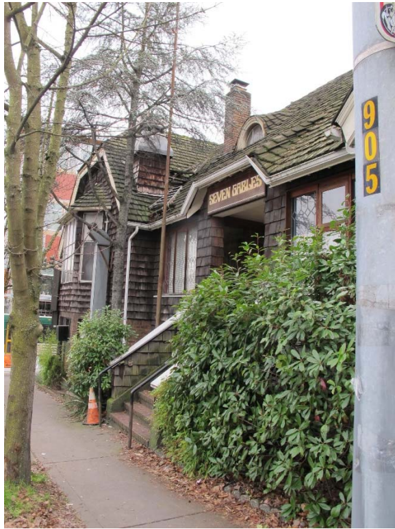
Fig. 33 – North elevation, viewing eastward
