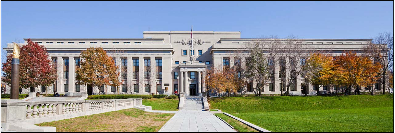
Fig. 13 – American Legion National Headquarters, Indianapolis, Indiana (Walker & Weeks, 1948-50)
