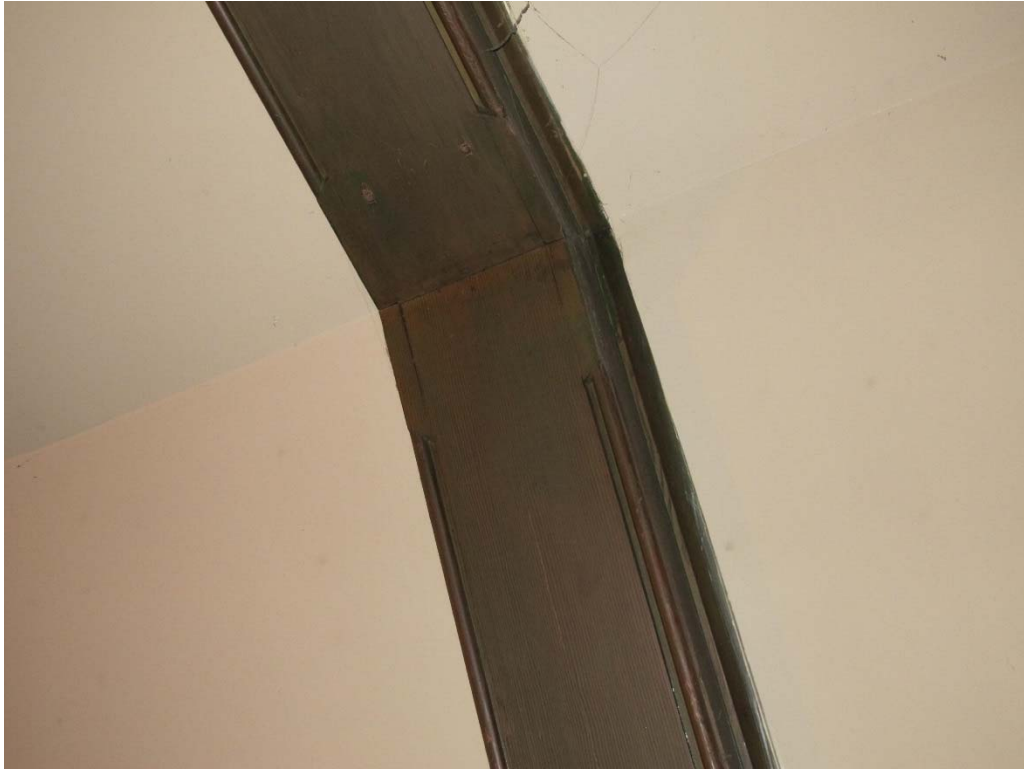
Fig. 87 – Interior main level, theater, detail of ceiling beams.
