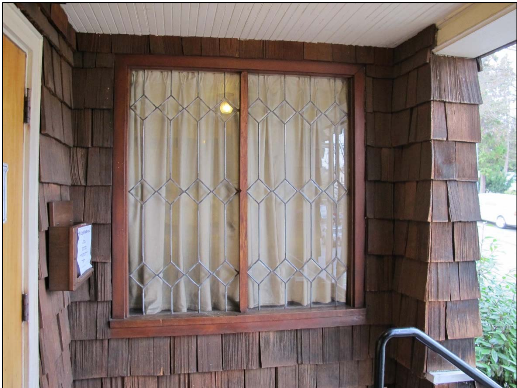
Fig. 42 – North elevation, window at west interior porch wall
