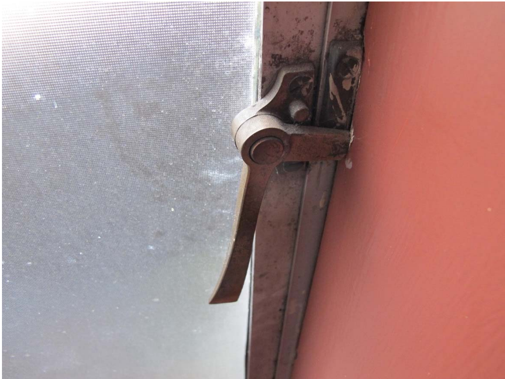
Fig. 72 – Interior main level, lounge, detail of window.
