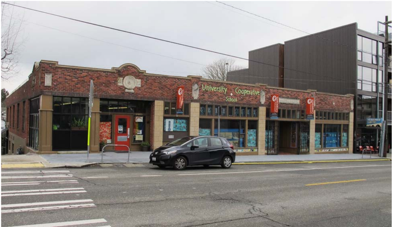
Fig. 22 – Cowen Park Garage/Maxwell Building (1925, Eric Rising, altered)
