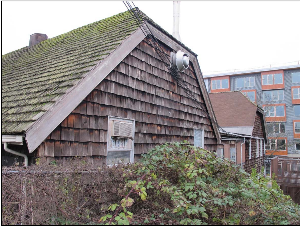
Fig. 52 – South elevation, upper part, view from the west
