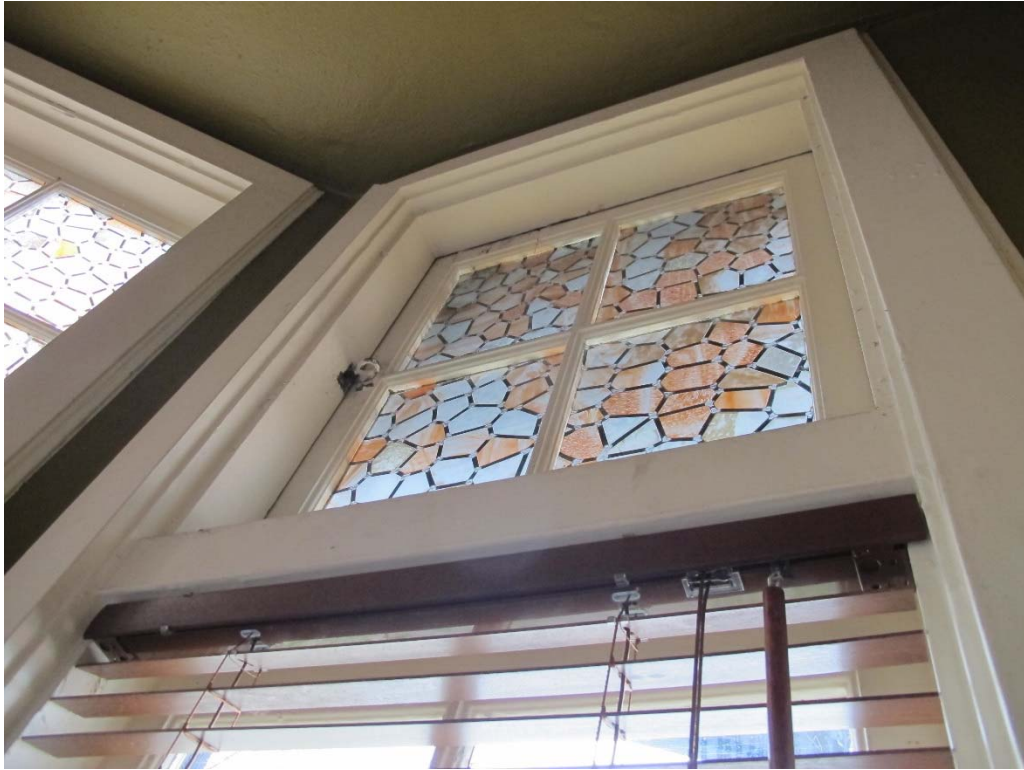
Fig. 101 – Interior lower level, restaurant dining room detail of bay window on north elevation.
