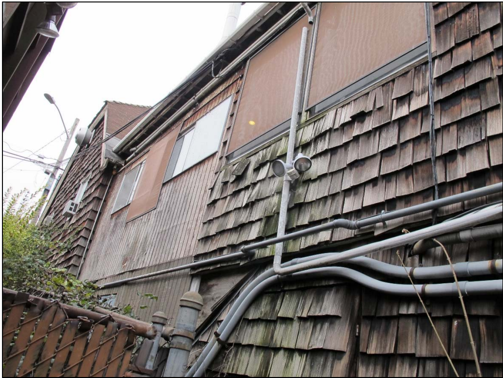
Fig. 53 – South elevation, upper part, view from the east (sidewalk). Infilled rear stair (see interior photos) visible at left of center.
