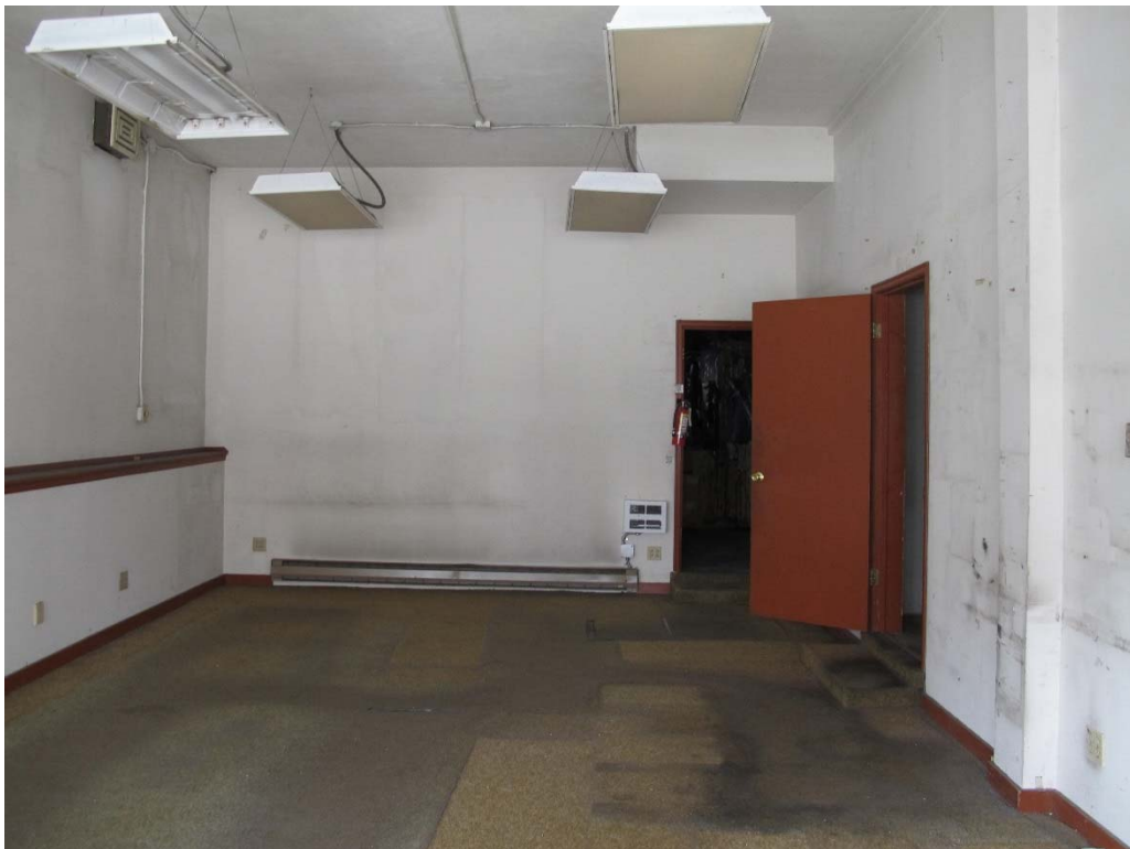
Fig. 108 – Interior lower level, tenant commercial space at southeast building corner.
