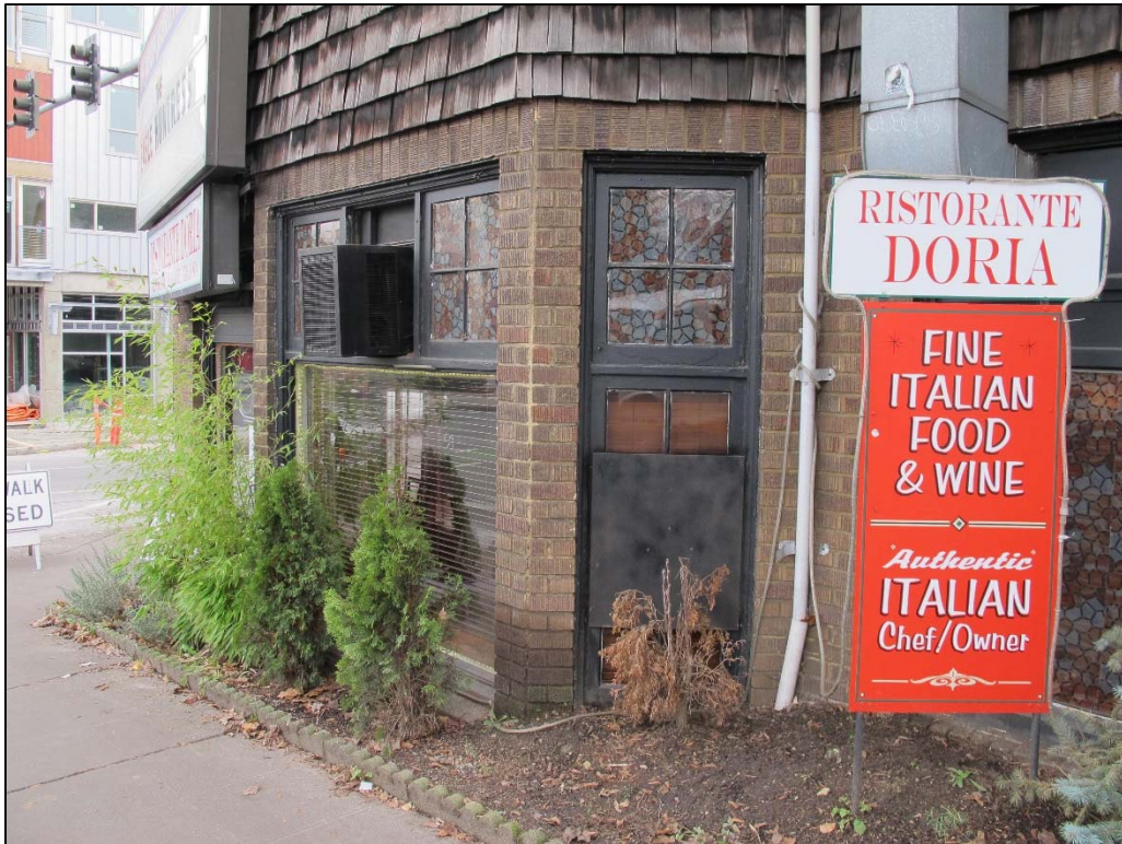
Fig. 37 – North elevation, bay window at first floor northeast corner
