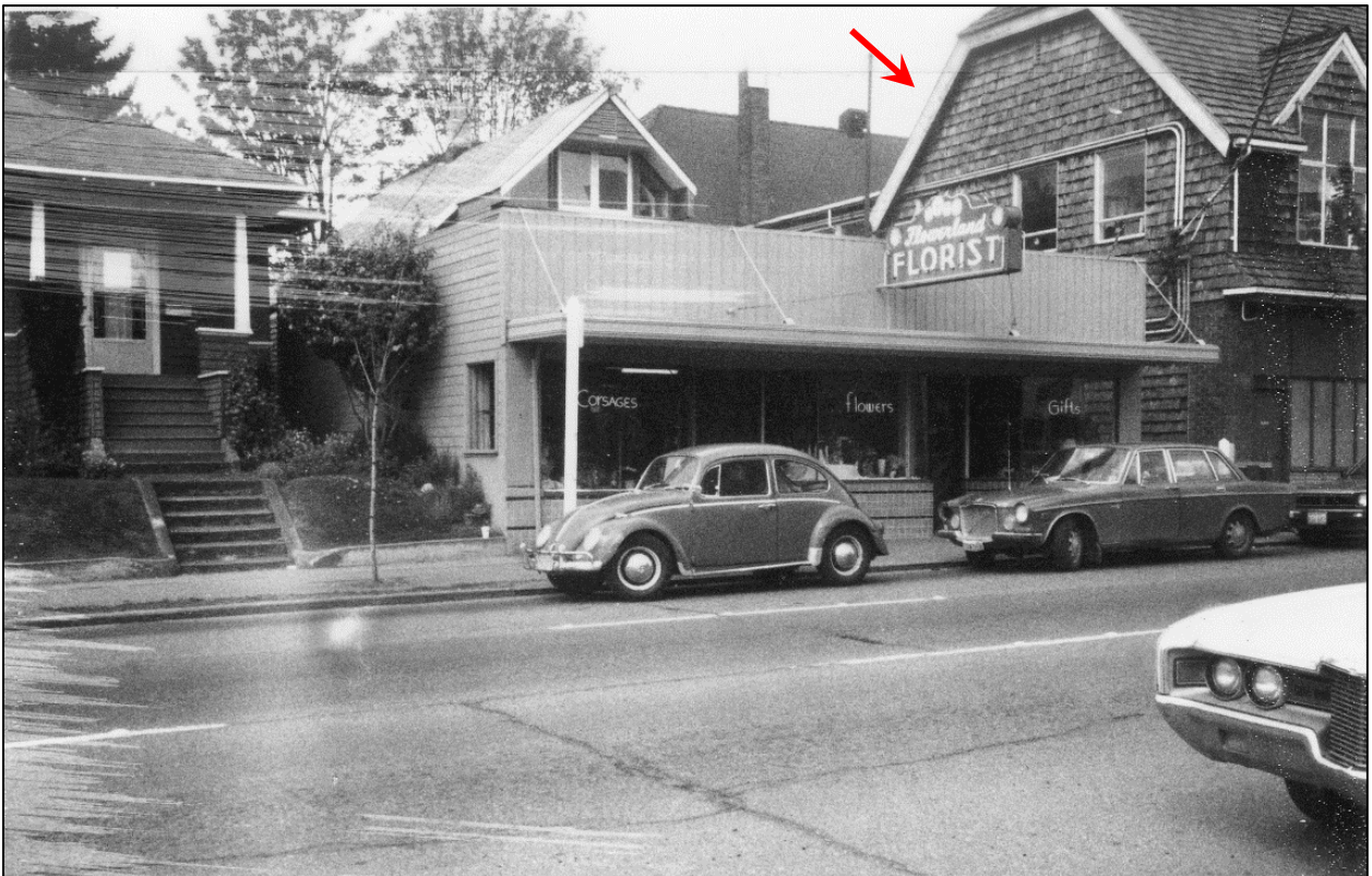
Fig. 9 – Detail, 1982 tax assessor photo of adjacent building, showing west elevation of the subject building.
