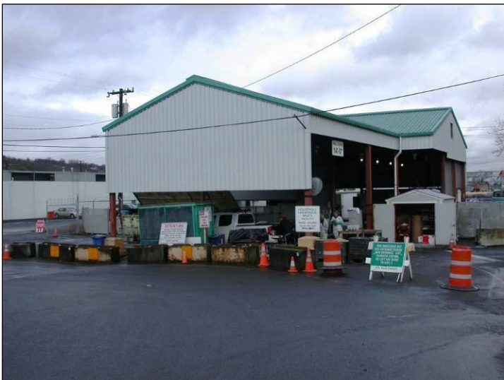
Fig. 39: Household Hazardous Waste Collection Shed, south and east facades. (March, 2008)
