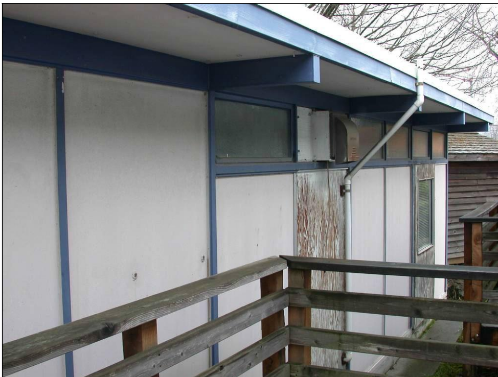
Fig. 35: Detail of the rear, west façade of the original Operations Building. (March, 2008)
