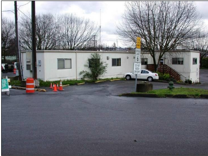
Fig. 38: Current Administrative Operations building, south and west facades. (March, 2008)
