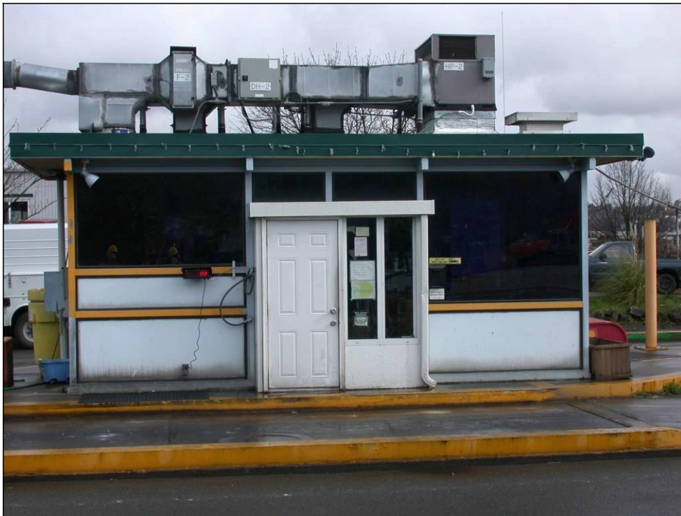
Fig. 28: The current south elevation of the Scale House. The building was re-located and re-oriented in 1989. (March, 2008)
