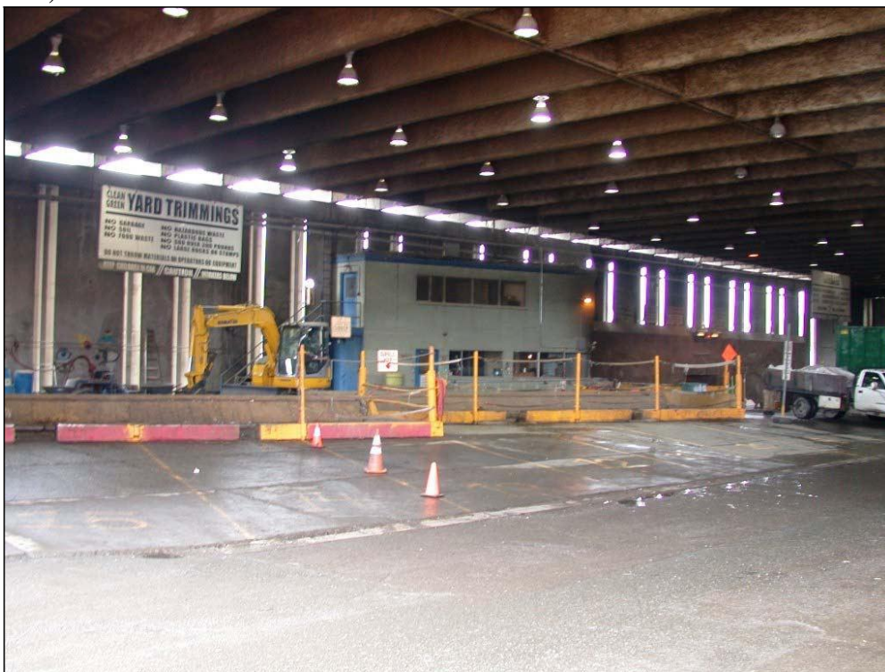
Fig. 24: Viewing east towards the interior west elevation of the east wall and the tipping stalls that receive yard waste/compostable materials. The office/storage building is beyond. (March, 2008)
