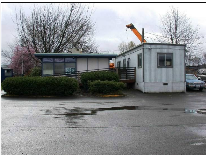
Fig. 33: The original Operations Building, north elevation. The modular trailer unit was added on the west side in 1985. (March, 2008)
