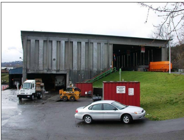
Fig. 18: View of the north façade. The tipping floor exit is at the upper level on the right. Truck entry to the loading level is on the lower left side. (March, 2008)
