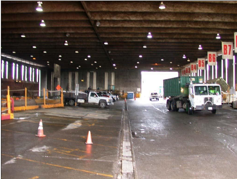
Fig. 25: Viewing south towards the entry. Tipping bays are on the left (east) and the driving lane is on the right (west). (March, 2008)
