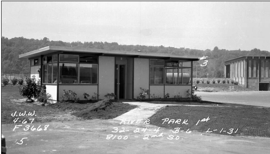
Fig. 31: Historic Tax Assessor file photo of the Operations Building, 1967, south and east facades.
