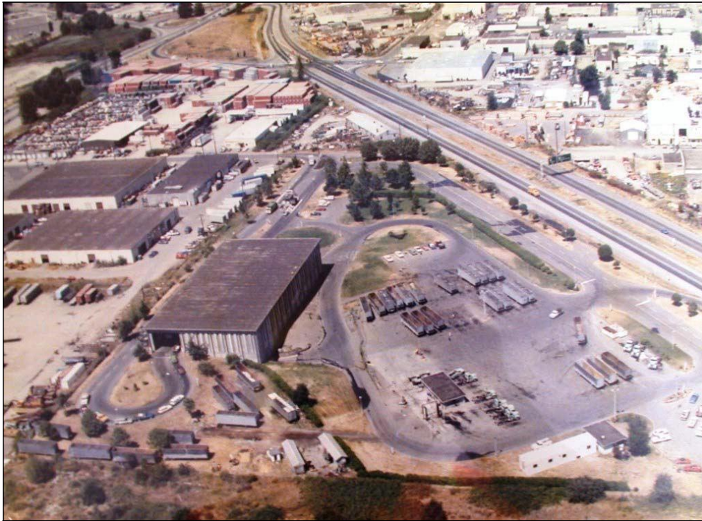
Fig. 5: This 1985 aerial photo, viewing north, shows the original configuration of the circulation and facilities on the site. The original public entrance was on the north end at South Kenyon St. (Seattle Public Utilities)
