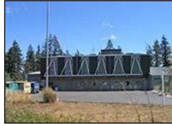
Fig. 49: King County Transfer Station-Vashon, constructed in 2001. (King County Solid Waste Division)
