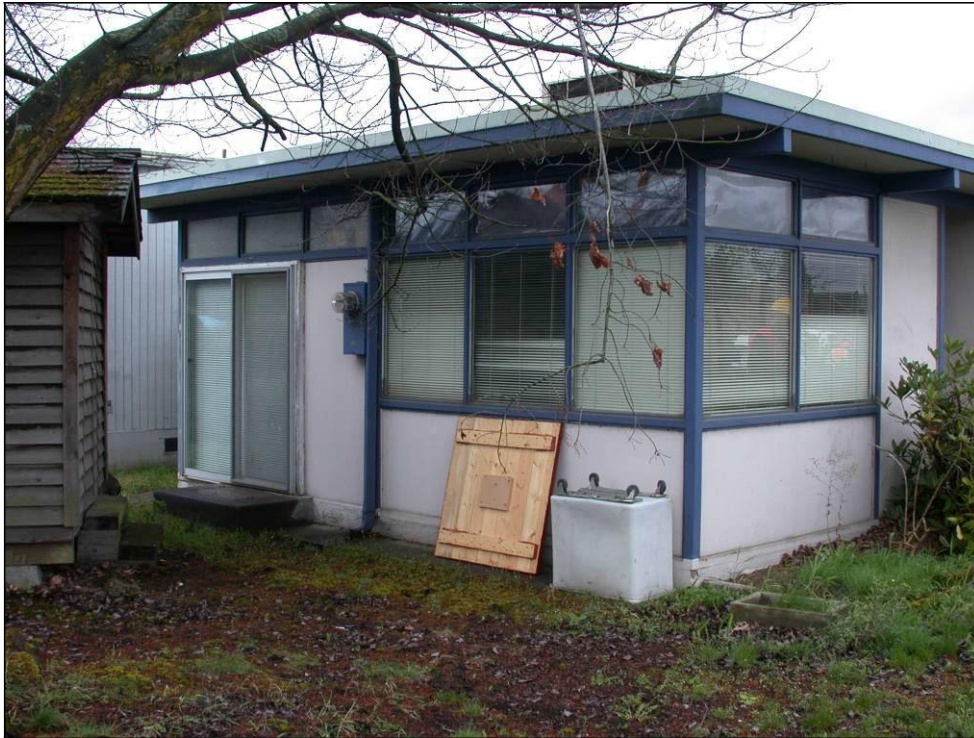
Fig. 34: South and partial east facades of the original Operations Building. The sliding glass doors are not original. (March, 2008)
