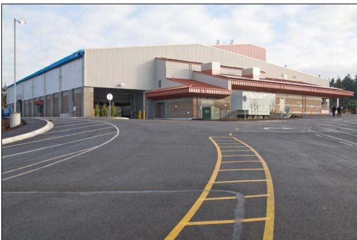
Fig. 52: Shoreline Recycling and Transfer Station Facility (2008) (King County Solid Waste Division)
