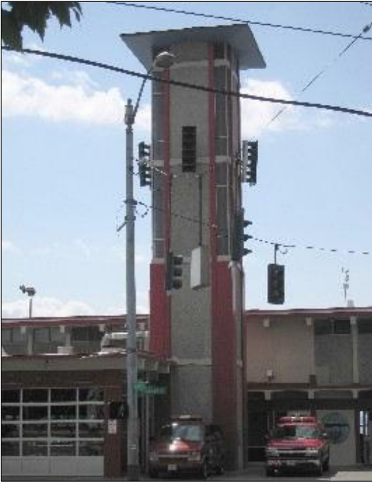
Fig. 43: Fire Station#5 (1963), Durham, Anderson & Freed. This building was awarded a citation from the Prestressed Concrete Institute and is a Seattle Landmark. Contemporary view. (DAHP/DoCoMoMo.WeWa)
