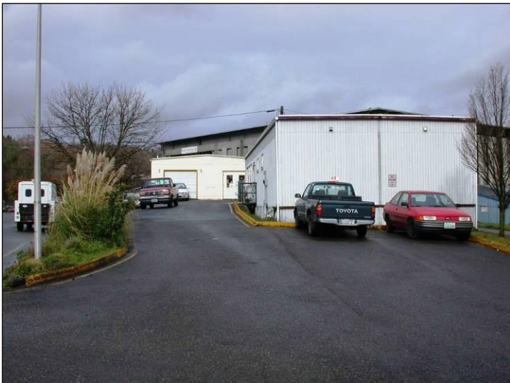
Fig. 40: Viewing northwest, showing south and west facades of Employee Locker Room/ Break Room building in the foreground. View of the partial south façade of the Warehouse/ storage building is beyond. Behind the storage building is the top of the Transfer Station's south façade. (March, 2008)
