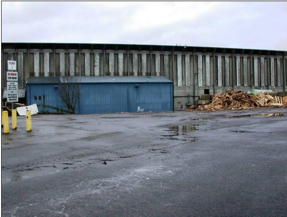
Fig. 21: East façade. The metal shed houses a compactor unit that was added in 1991. (March, 2008)
