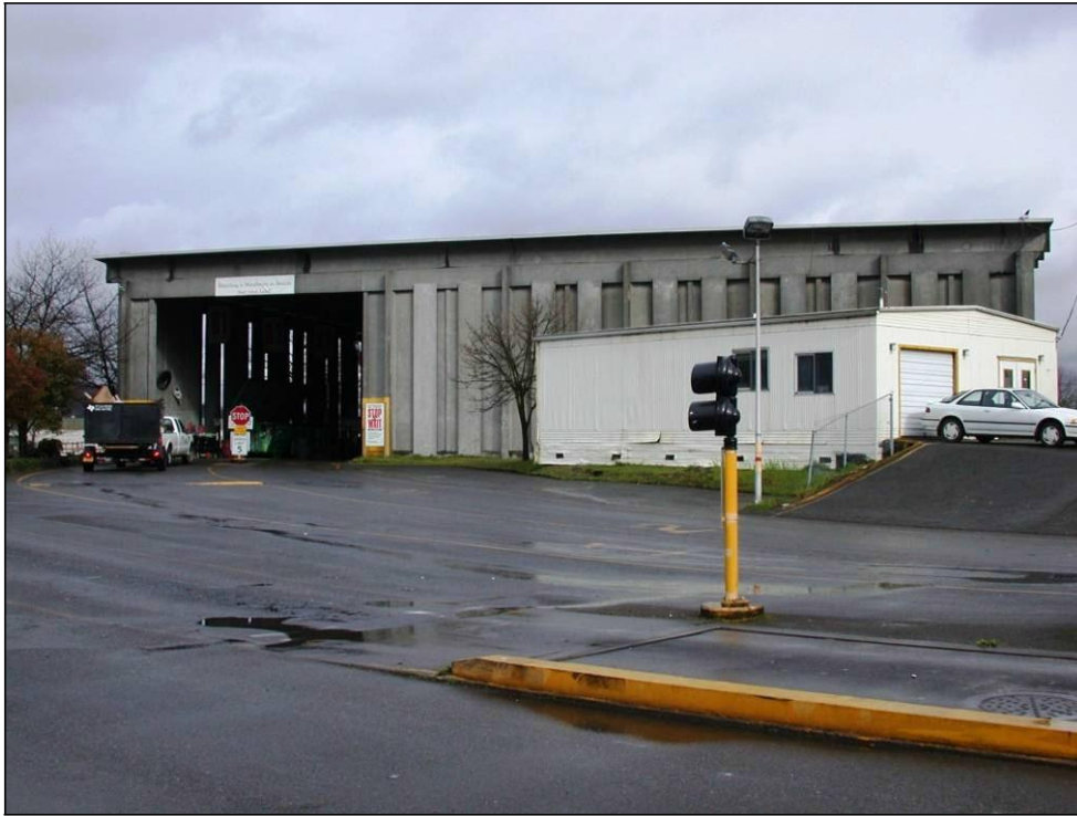
Fig. 19: The south facade, showing the entry of the tipping floor. The building to the right is a storage building. (March, 2008)
