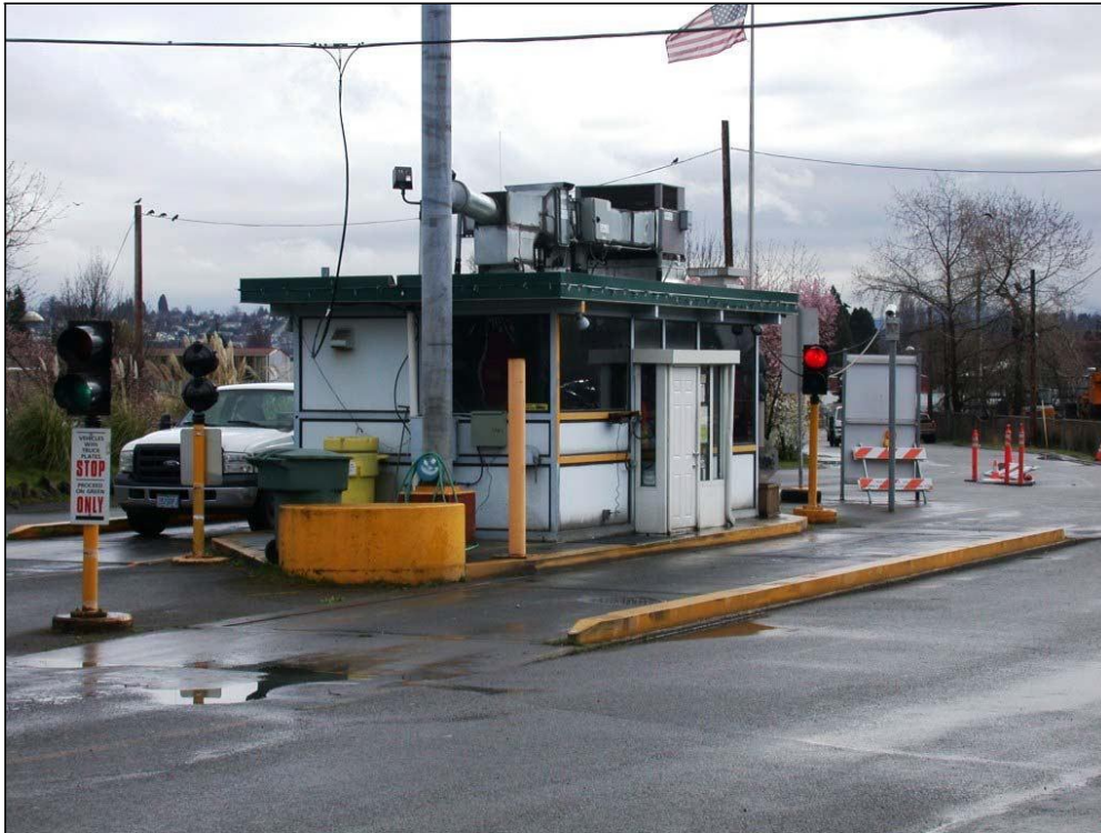
Fig. 29: The west and south facades of the Scale House. (March, 2008)
