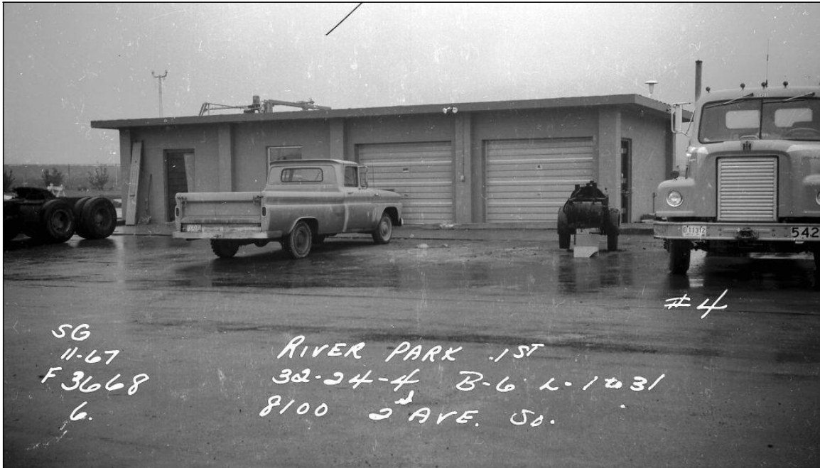
Fig. 36: Historic Tax Assessor File photo of the Service Garage, 1967, showing the east elevation. (Puget Sound Regional Archives)
