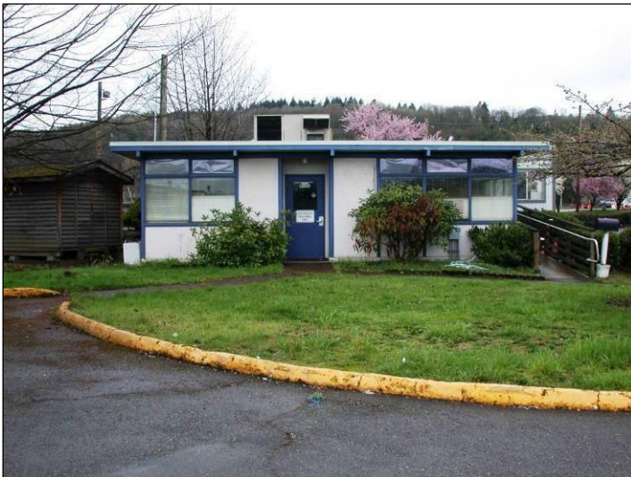
Fig. 32: East elevation of the original Operations Building. (March, 2008)
