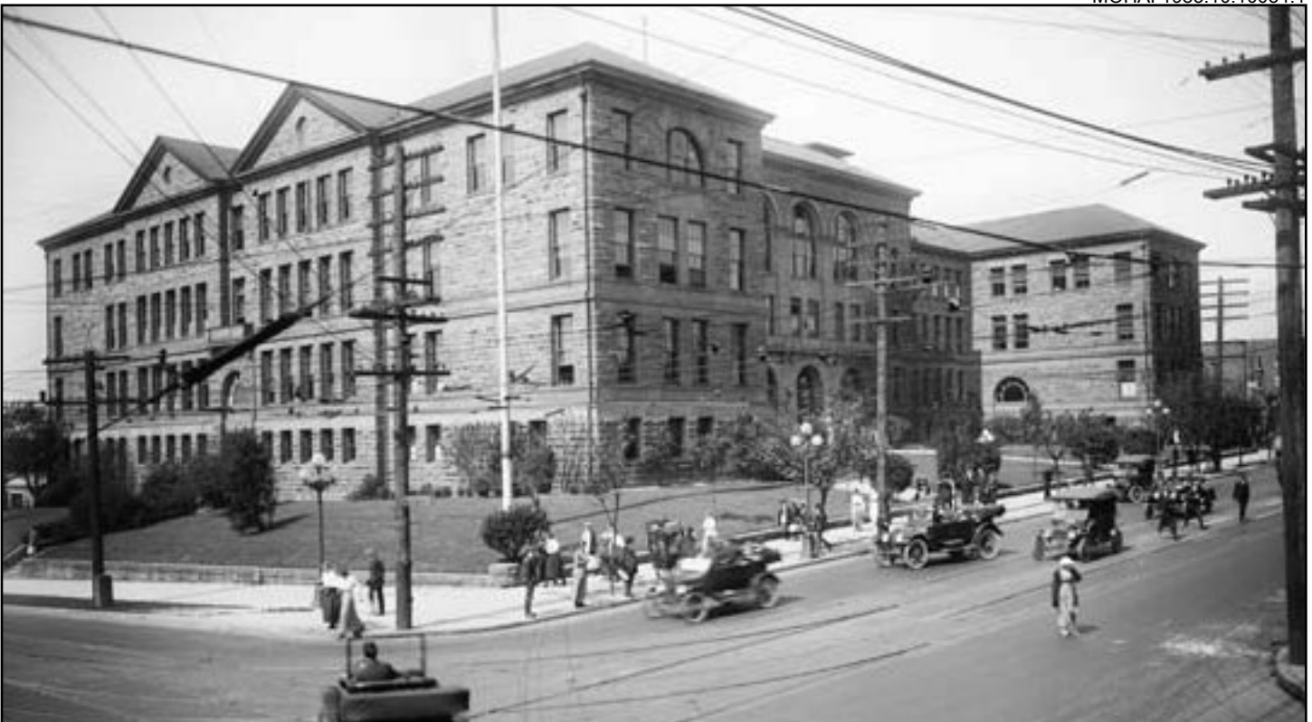
Figure 6. Central High School/Broadway High School (W.E. Boone & J.M. Corner, 1902)
