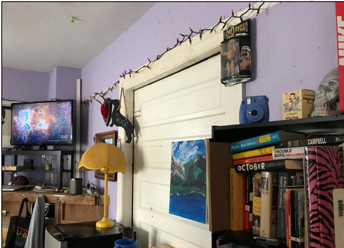
Figure 23 • Former parlor, pocket door detail
