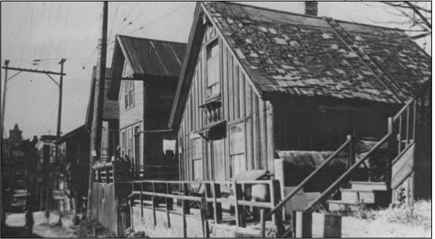
Figure 62 • Houses in the First Hill neighborhood, ca. 1940
