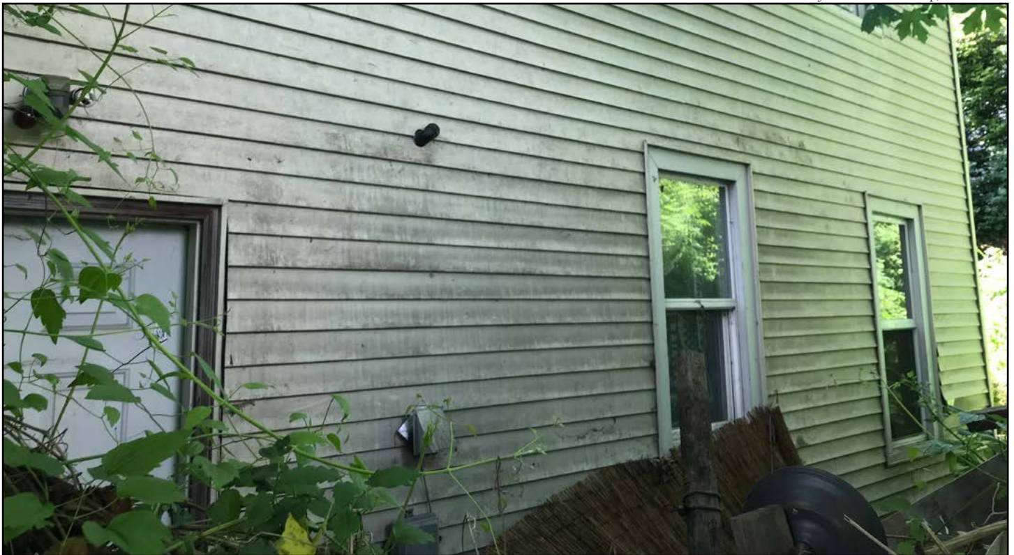
Figure 17 • 1010 East Spruce Street, northern façade, lower
