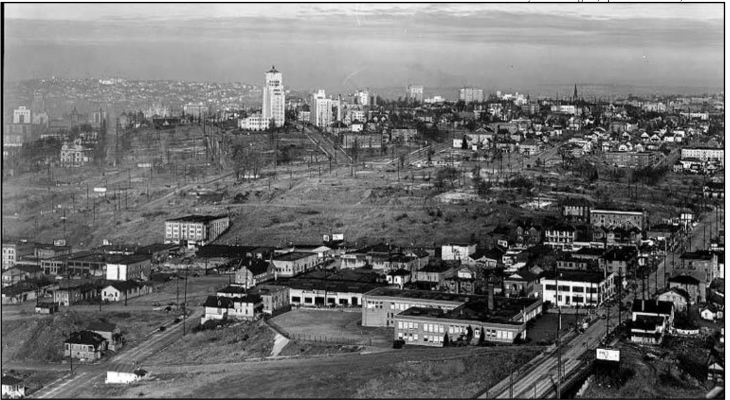
Figure 67 • First Hill during construction of Yesler Terrace, 1941
