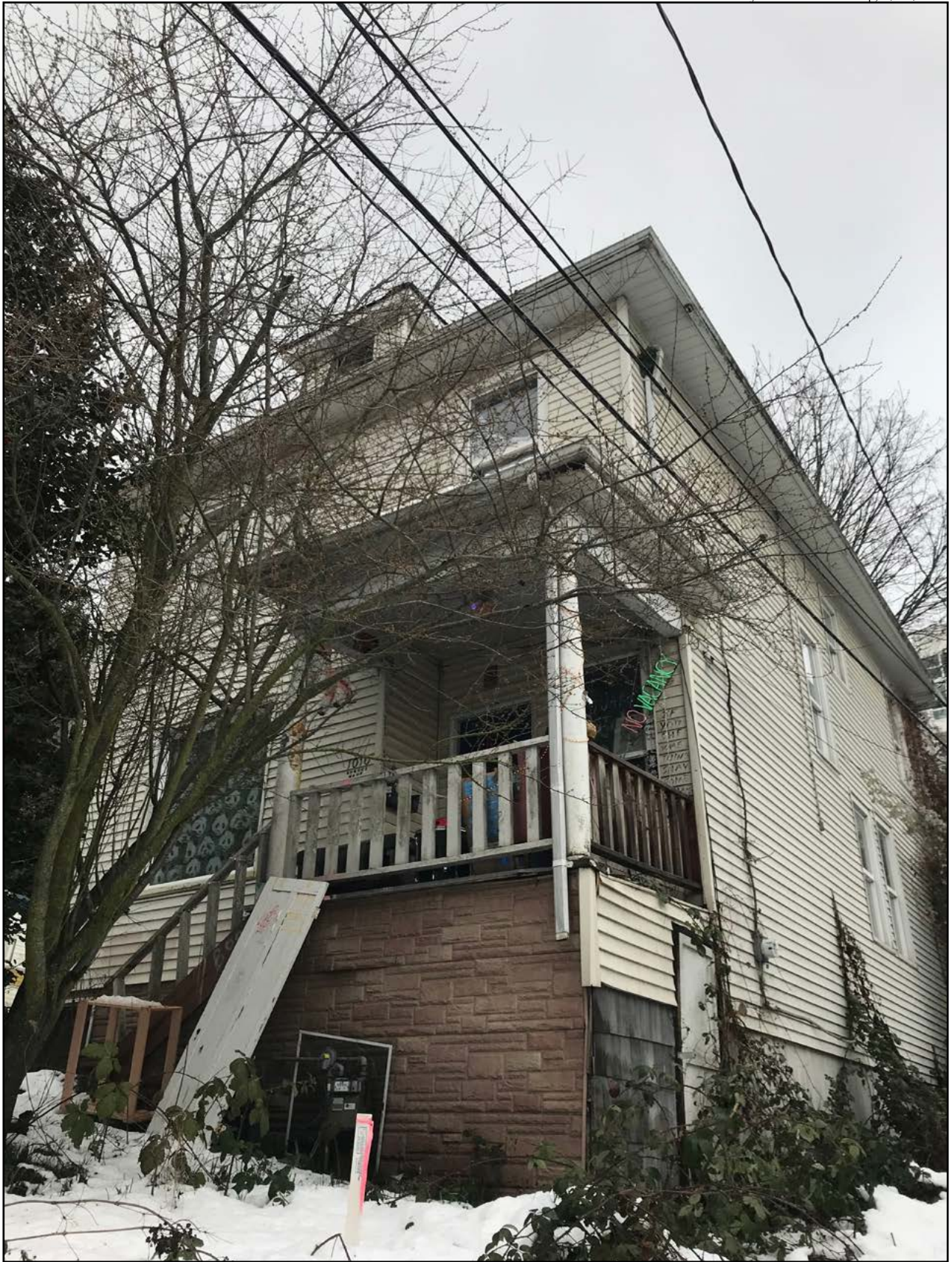
Figure 14 • 1010 East Spruce Street, southeastern corner, recessed porch
