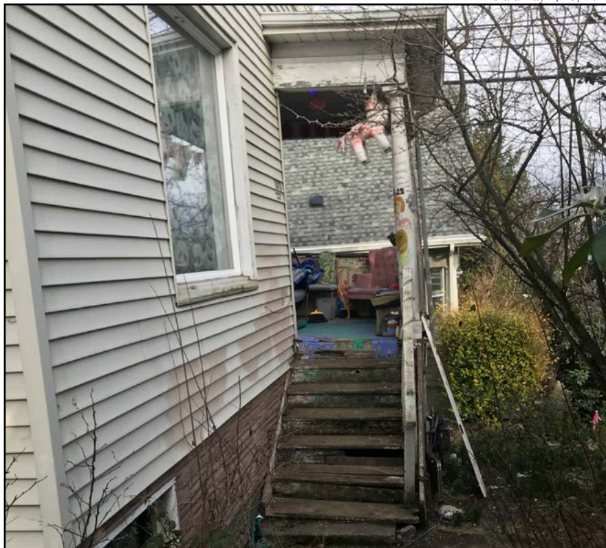
Figure 13 • 1010 East Spruce Street, southern façade, recessed porch front detail
