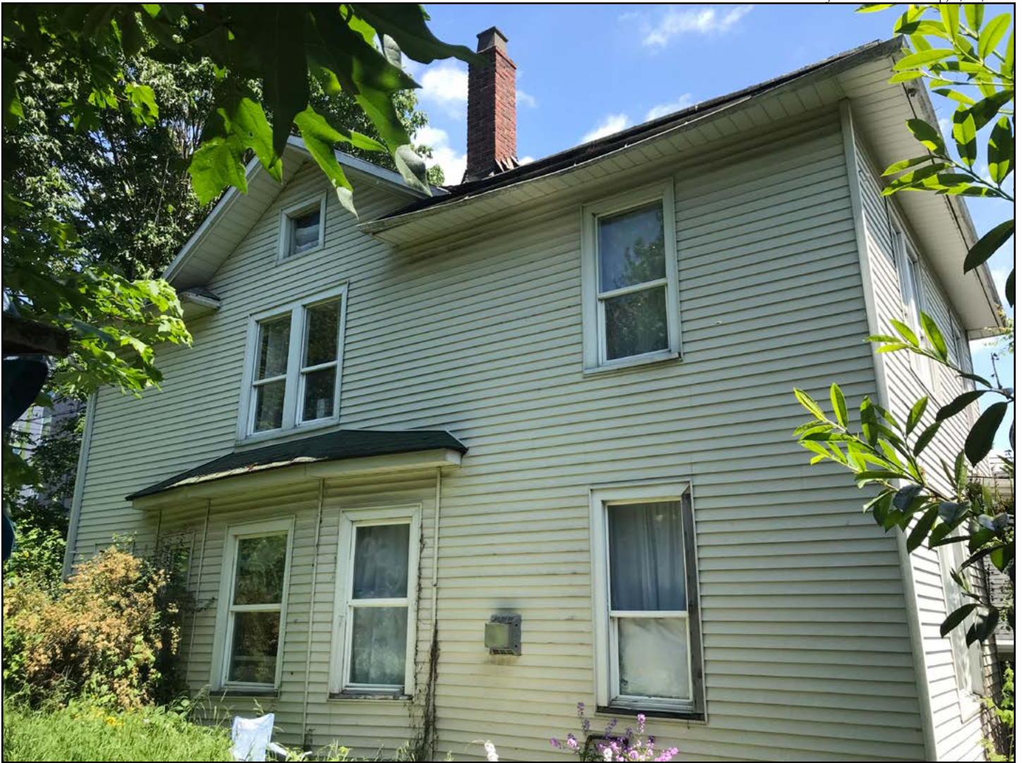
Figure 15 • 1010 East Spruce Street, western façade
