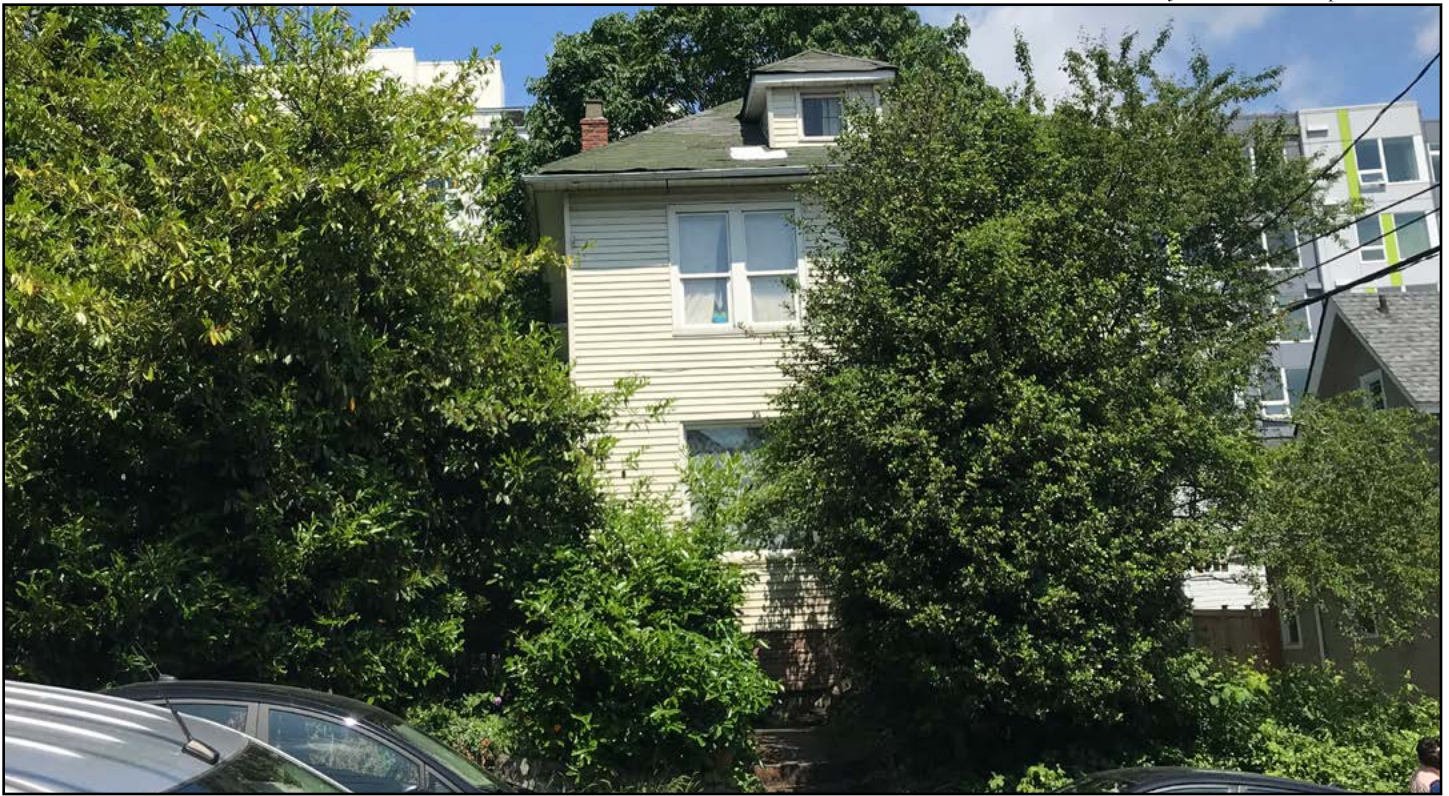
Figure 12 • 1010 East Spruce Street, southern façade
