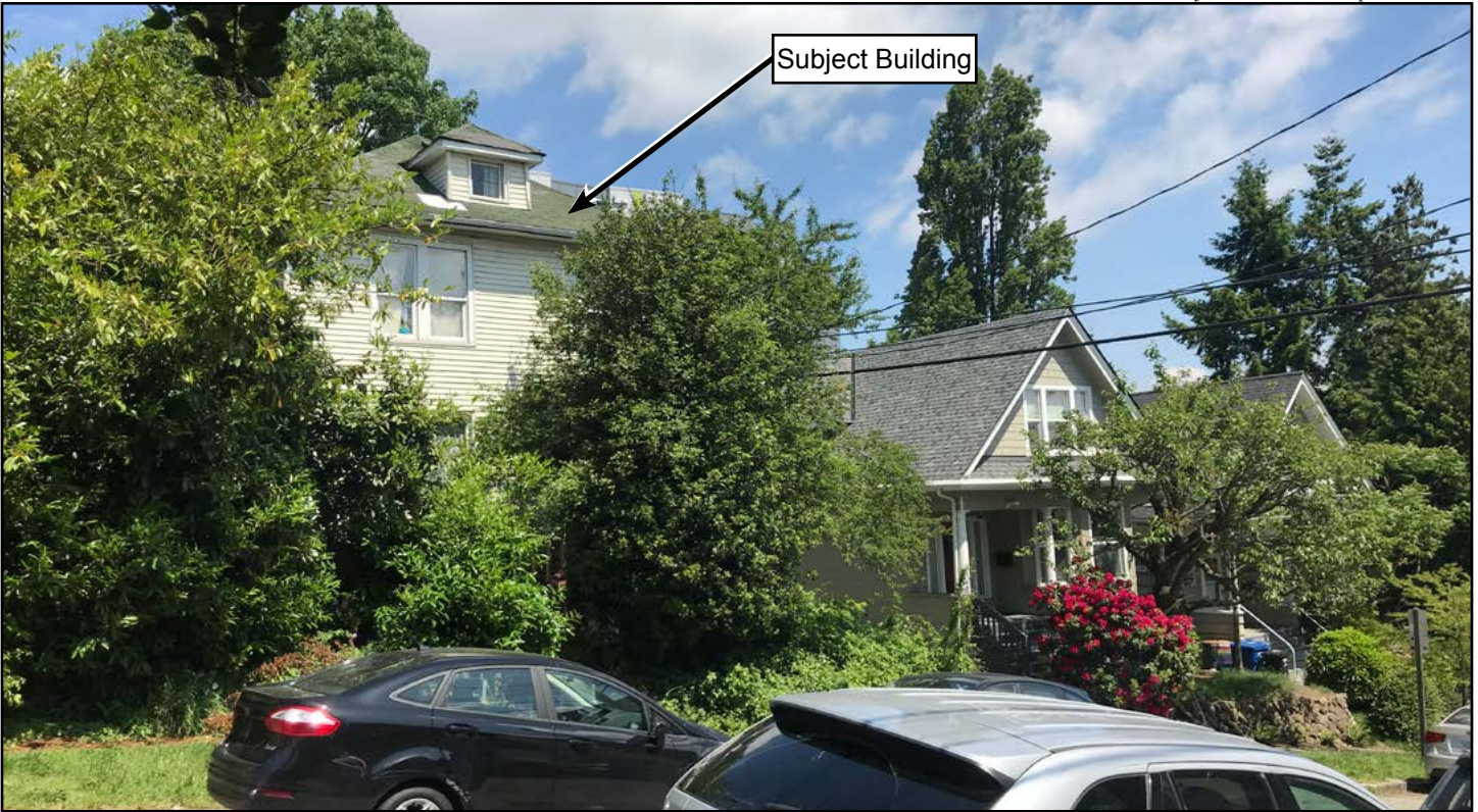
Figure 7 • View C - Viewing north on E Spruce Street
