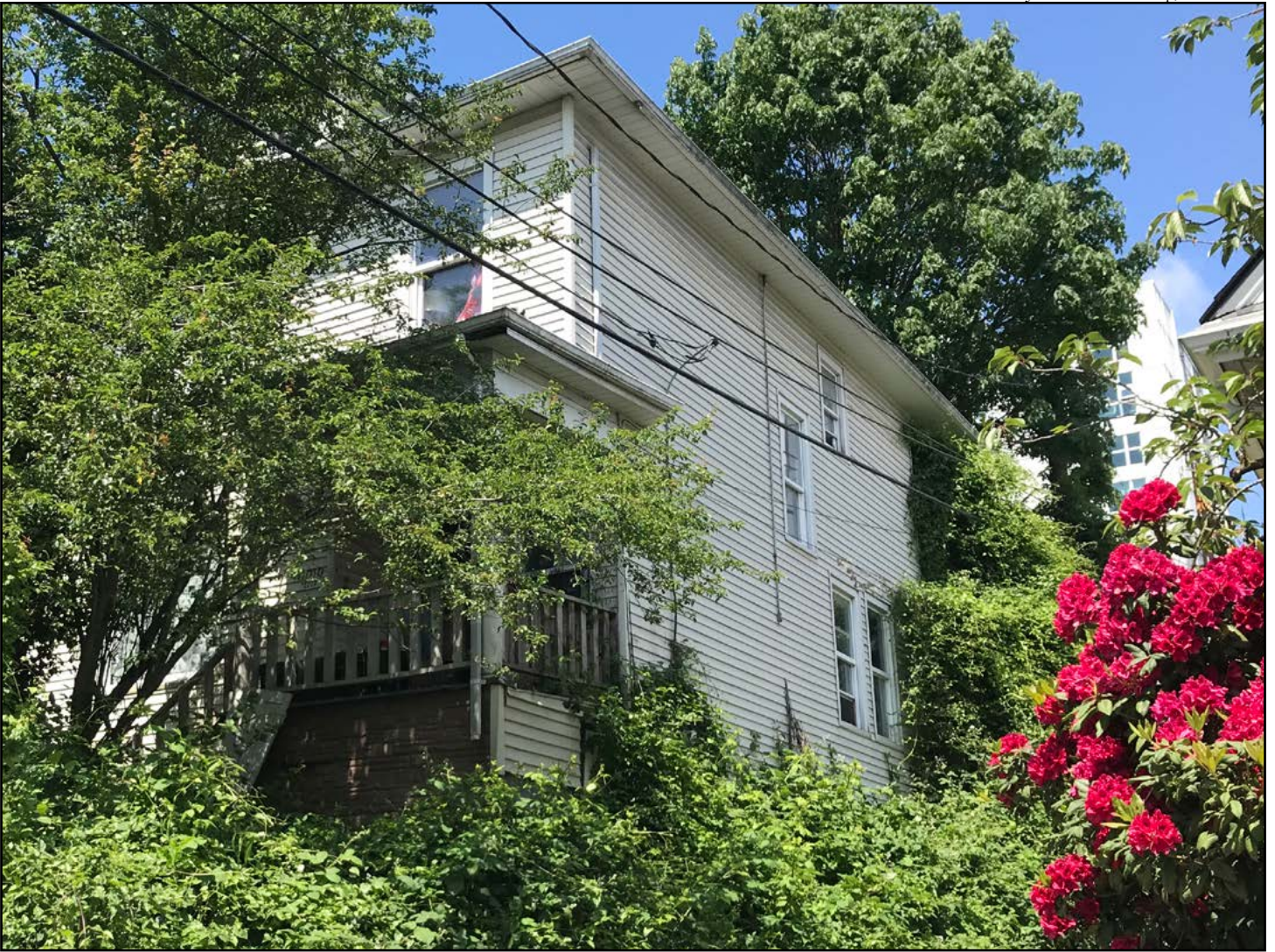
Figure 18 • 1010 East Spruce Street, eastern façade, lower
