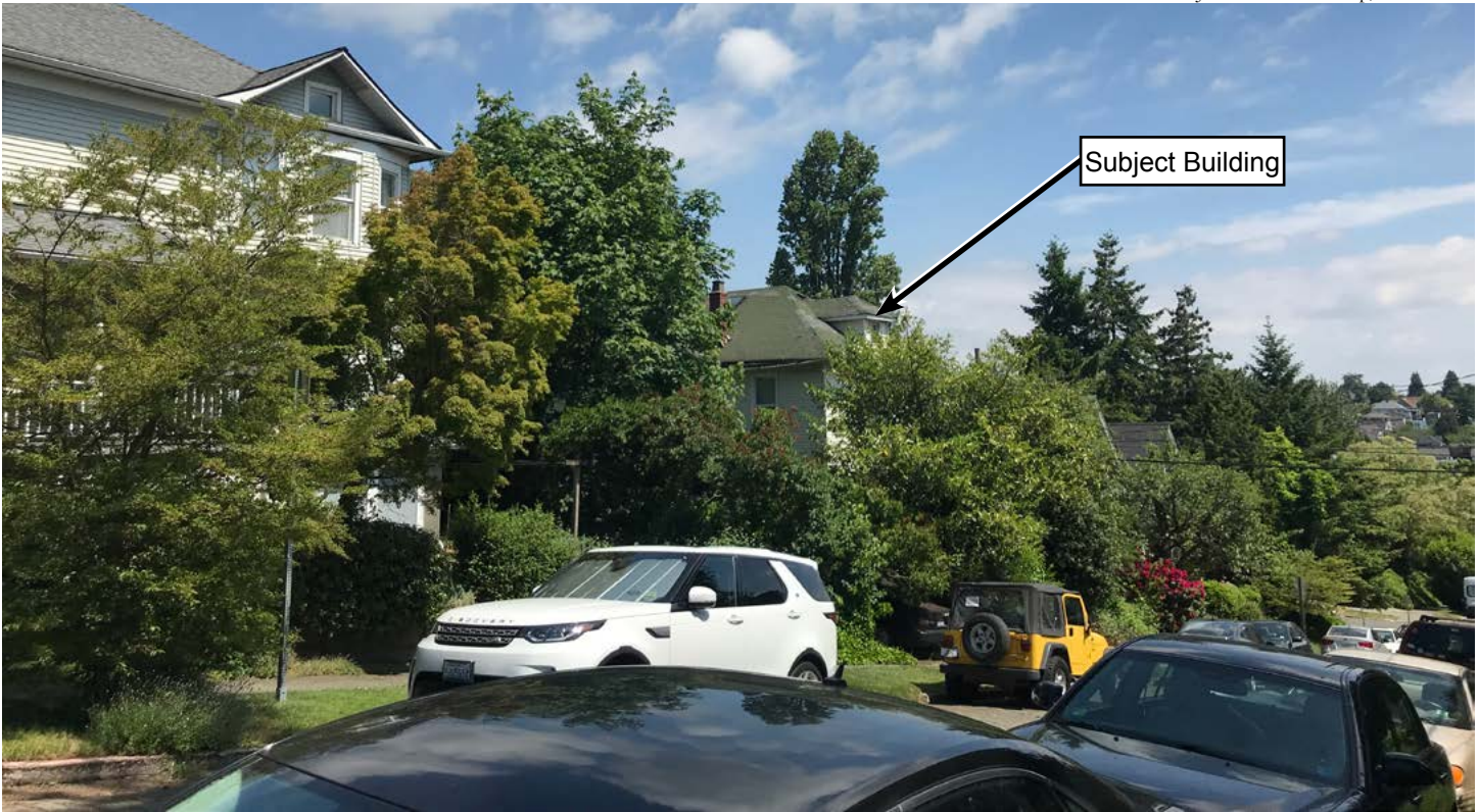
Figure 8 • View D - Viewing northeast on E Spruce Street
