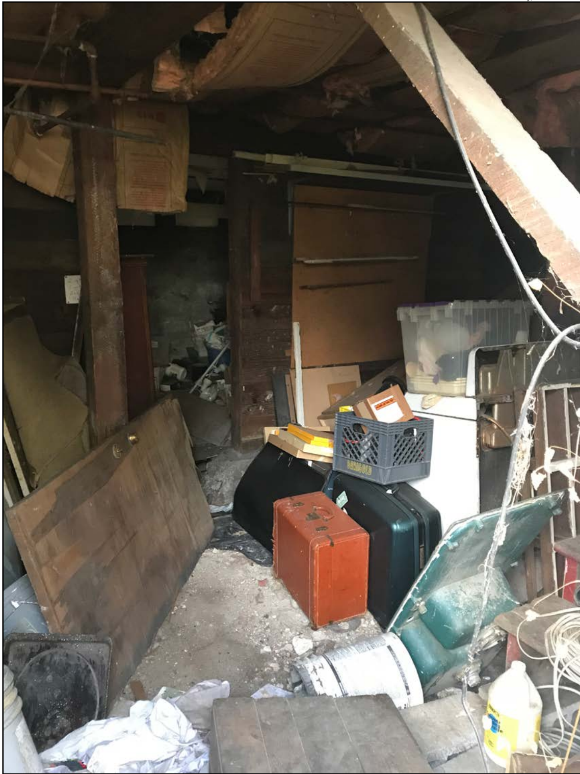
Figure 19 • View of basement
