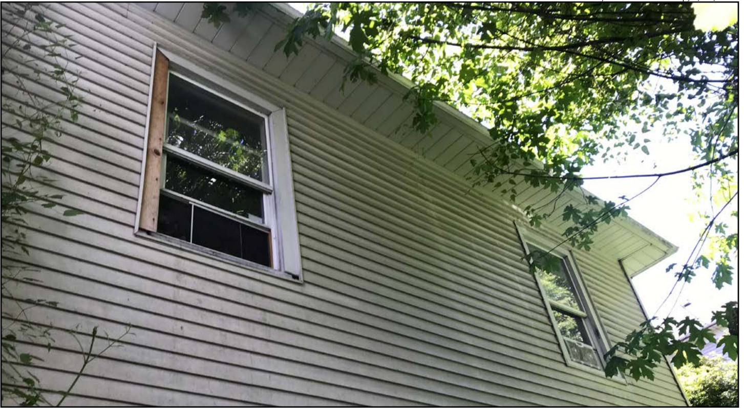
Figure 16 • 1010 East Spruce Street, northern façade, upper
