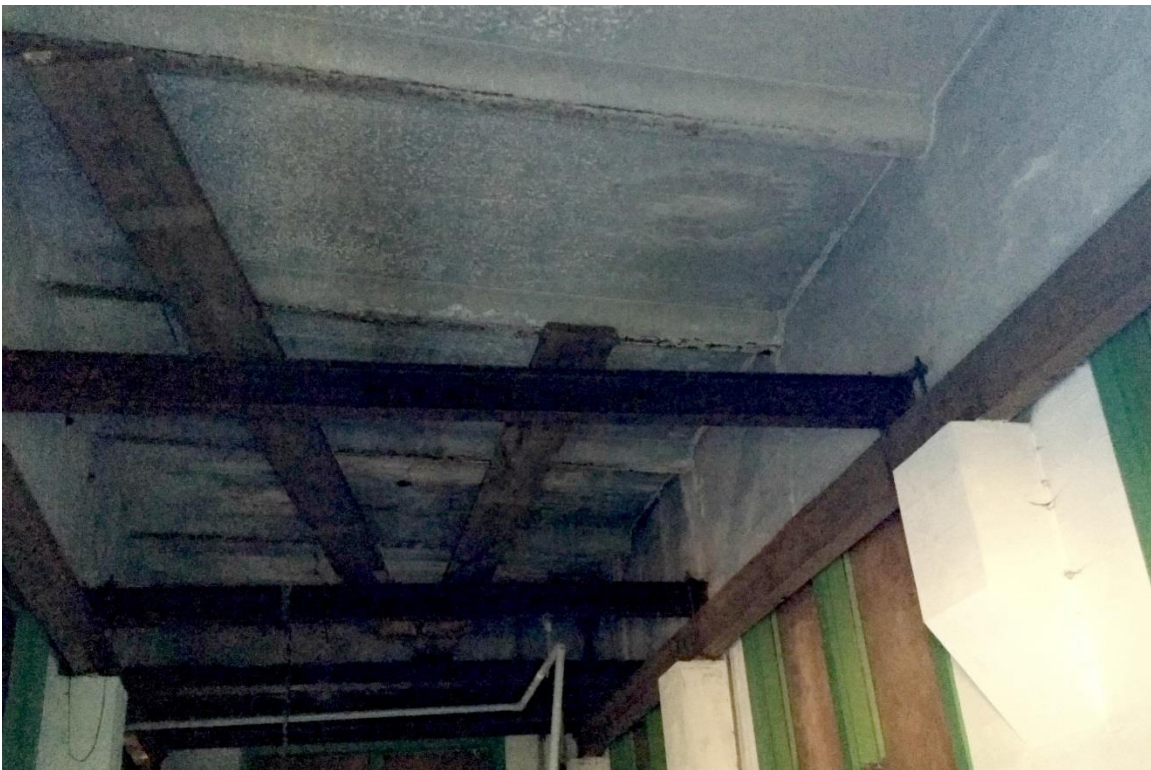
Photo 11 – Pump House Interior, View from North Window to Ceiling (Source: Seattle Parks and Recreation, 2019)
