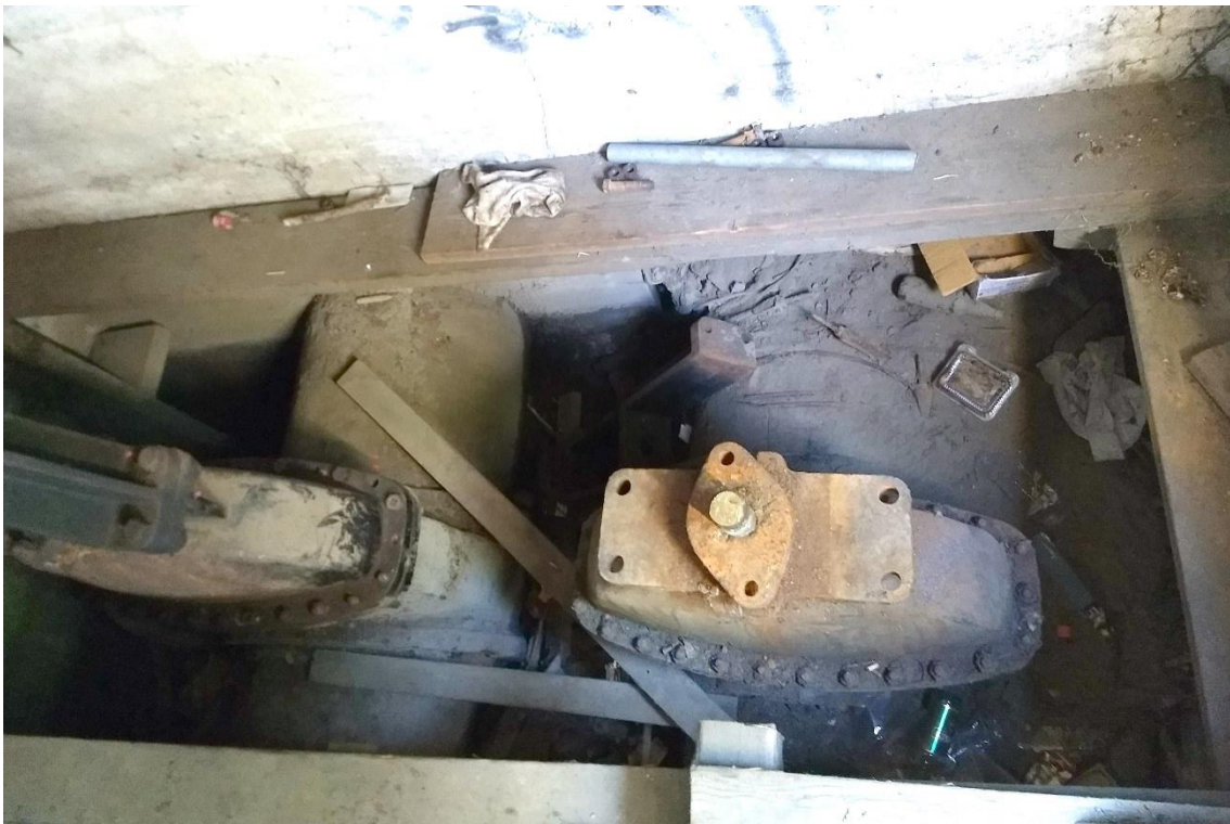
Photo 16 – Valve House Interior, View of Gate Valves and Cast Iron Pipelines Top Part of Right Gate Valve Stem Sawn Off (Source: Seattle Parks and Recreation, 2019)
