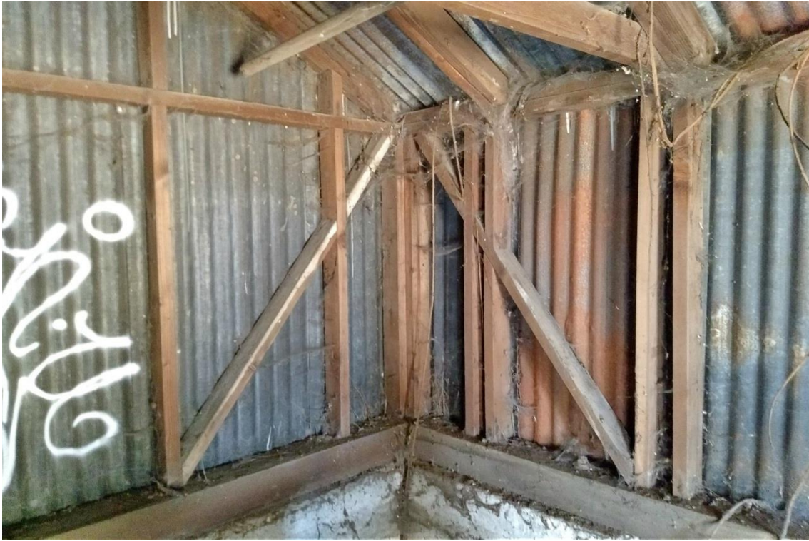
Photo 15 – Valve House Interior, View to Northeast Corner (Source: Seattle Parks and Recreation, 2019)
