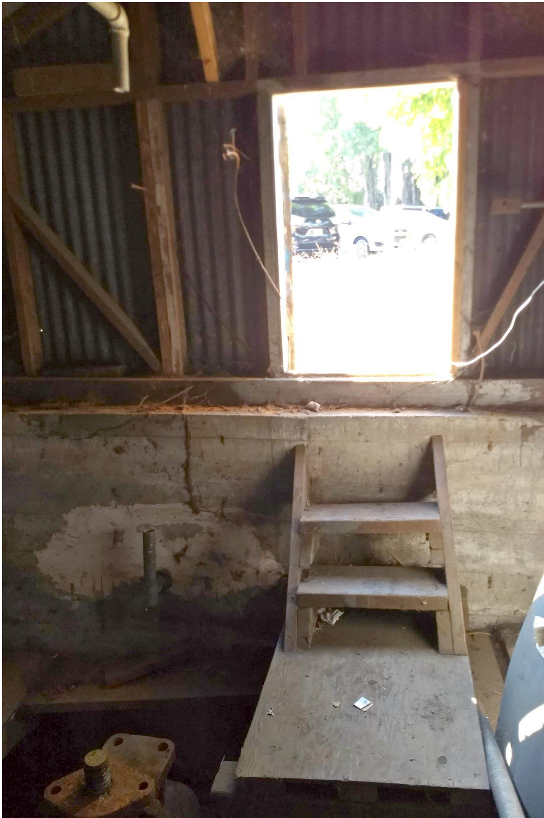
Photo 14 – Valve House Interior, View to Southeast Entrance
