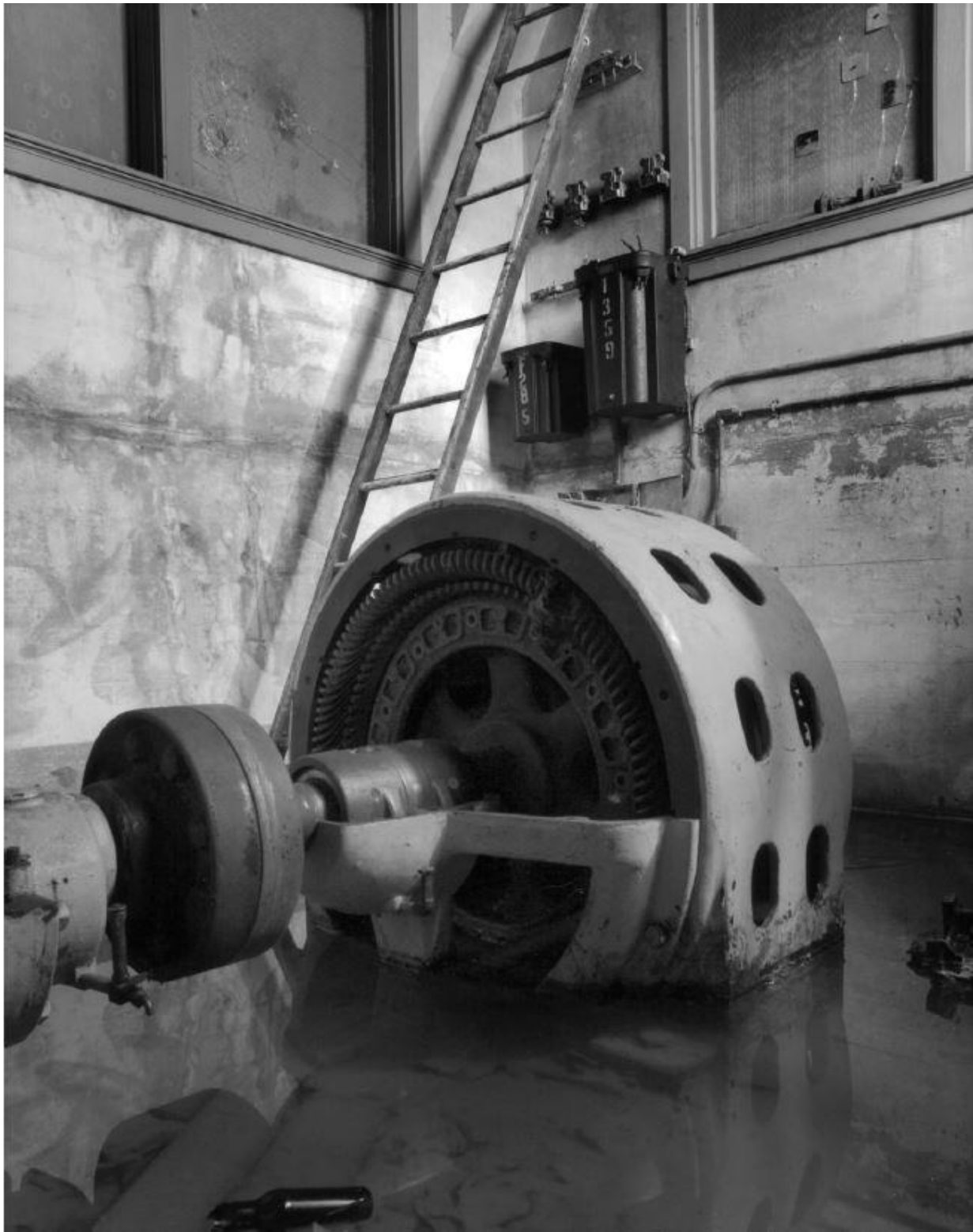
Photo 12 – Pump House Interior, View to Northwest Corner (Source: (Historic American Engineering Record (HAER), 2009), WA 1-69)
