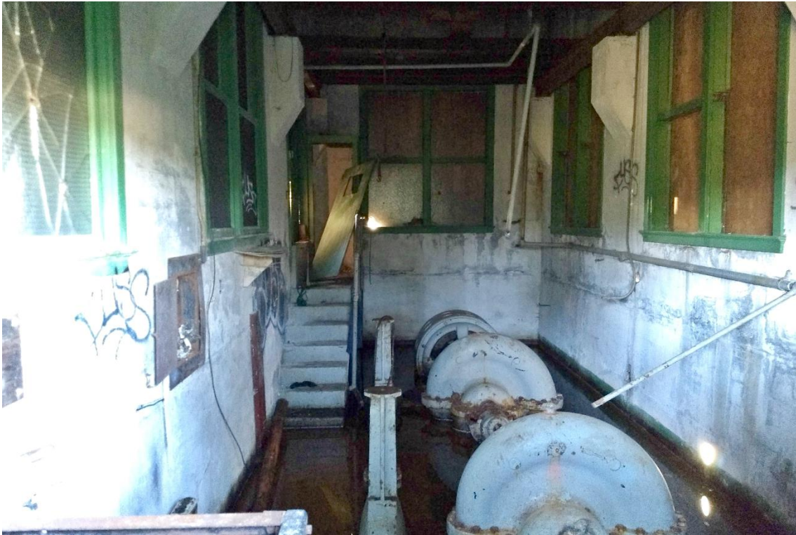
Photo 10 – Pump House Interior, View from North Window to Southwest Wall (Source: Seattle Parks and Recreation, 2019)
