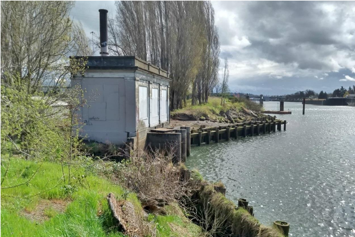
Photo 7 – Northwest and Southwest Elevations (Source: Seattle Parks and Recreation, 2019)
