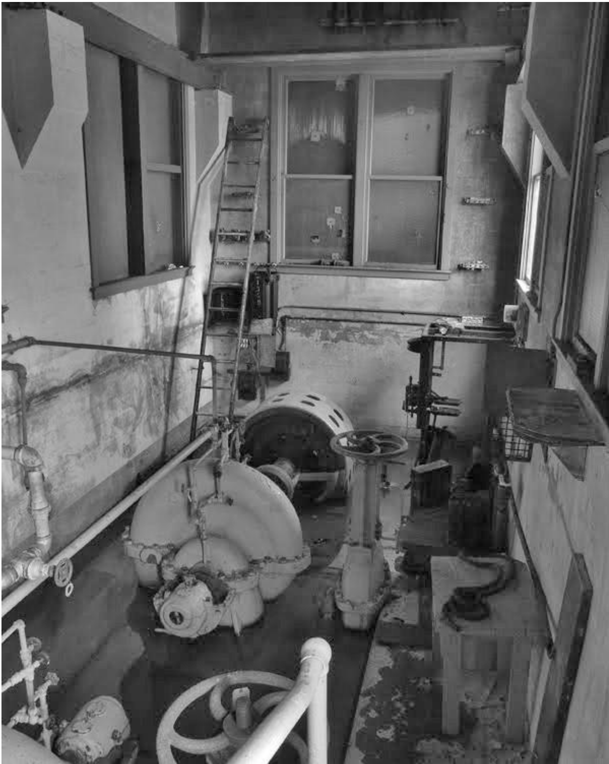
Photo 9 – Pump House Interior, View from Entry Platform to Northwest Wall (Source: (Historic American Engineering Record (HAER), 2009), WA 1-69)
