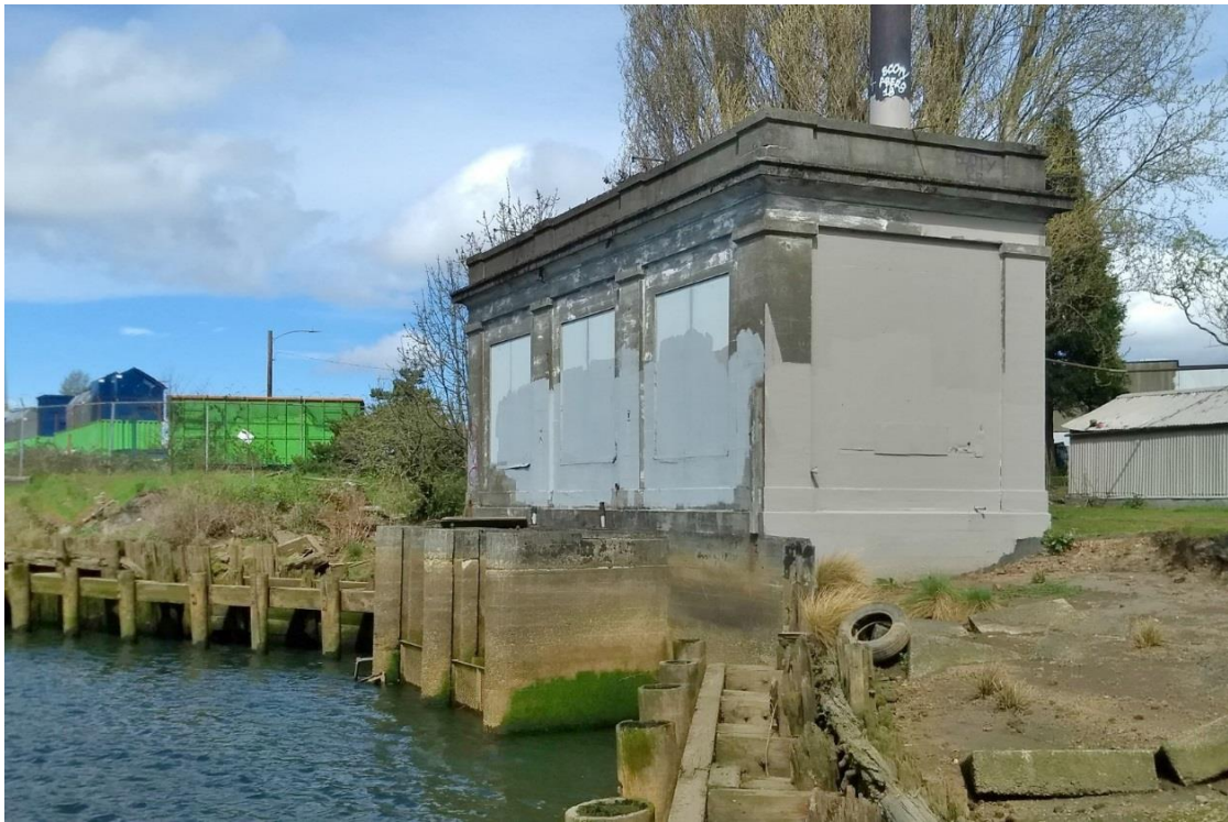
Photo 5 – Southwest and Southeast Elevations (Source: Seattle Parks and Recreation, 2019)
