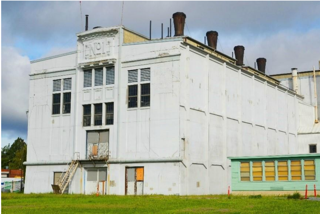
Photo 17 – GTSP Southeast Elevation (Source: Seattle City Light Collection, 2018)
