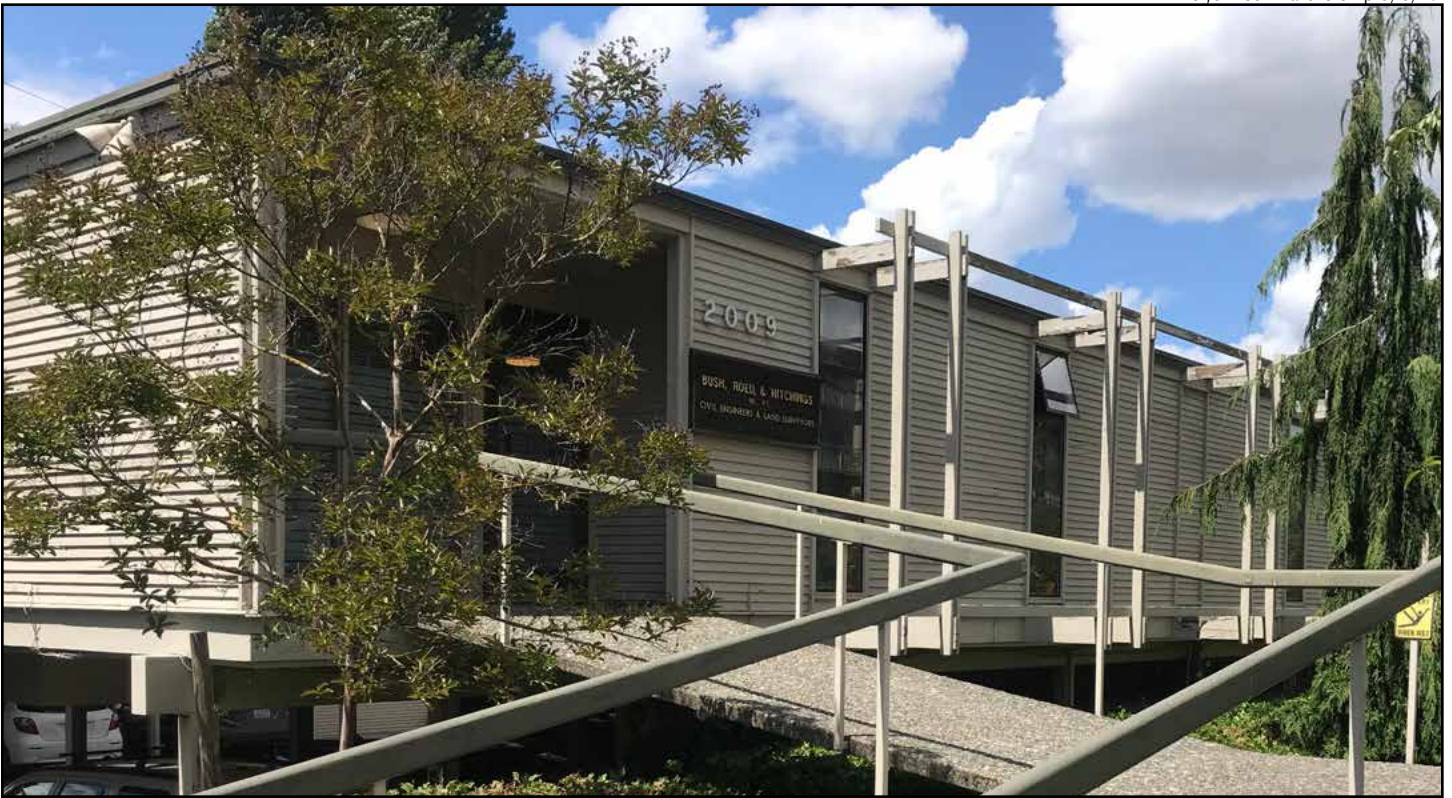
Figure 16 • 2009 Minor Avenue E, entry at eastern façade
