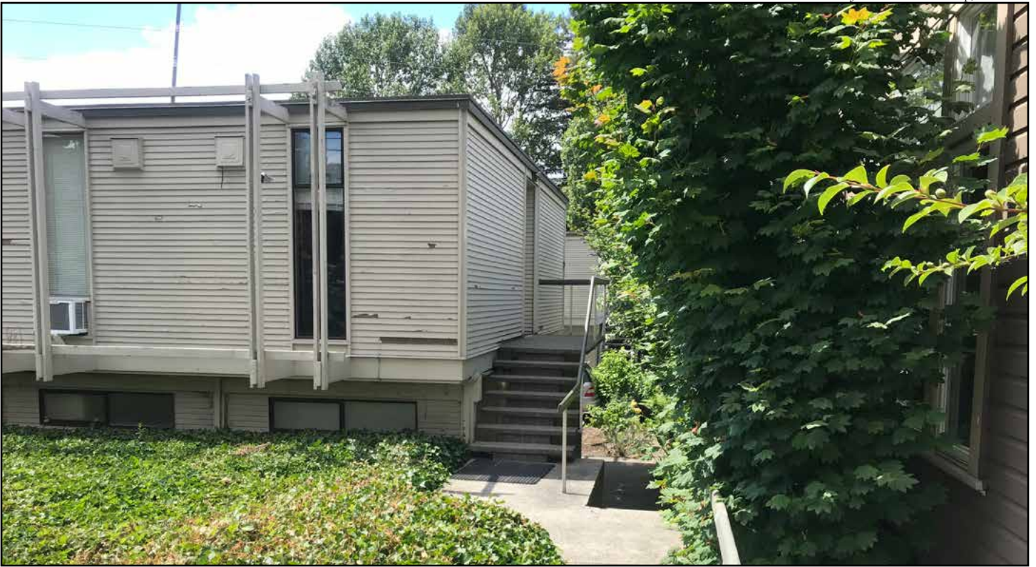
Figure 20 • 2009 Minor Avenue E, viewing west along northern façade at eastern wing
