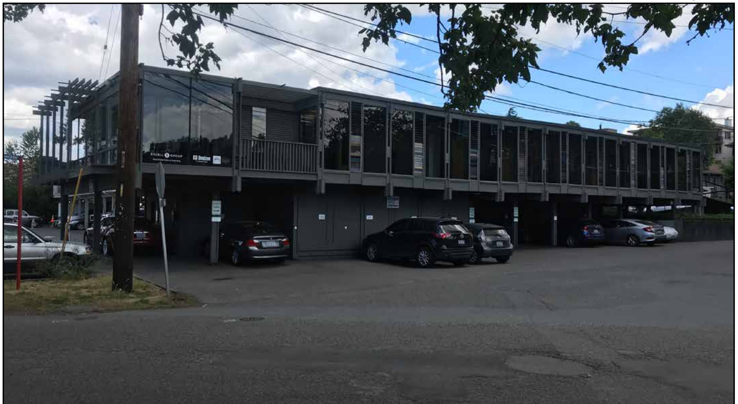
Figure 8 • View F - 2000 Fairview Avenue E, former offices of Kirk, Wallace, McKinley & Associates
