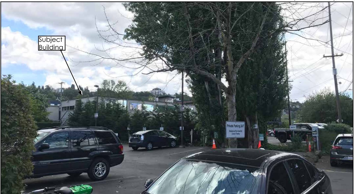
Figure 4 • View B - Viewing southeast across Fairview Avenue E towards subject building
