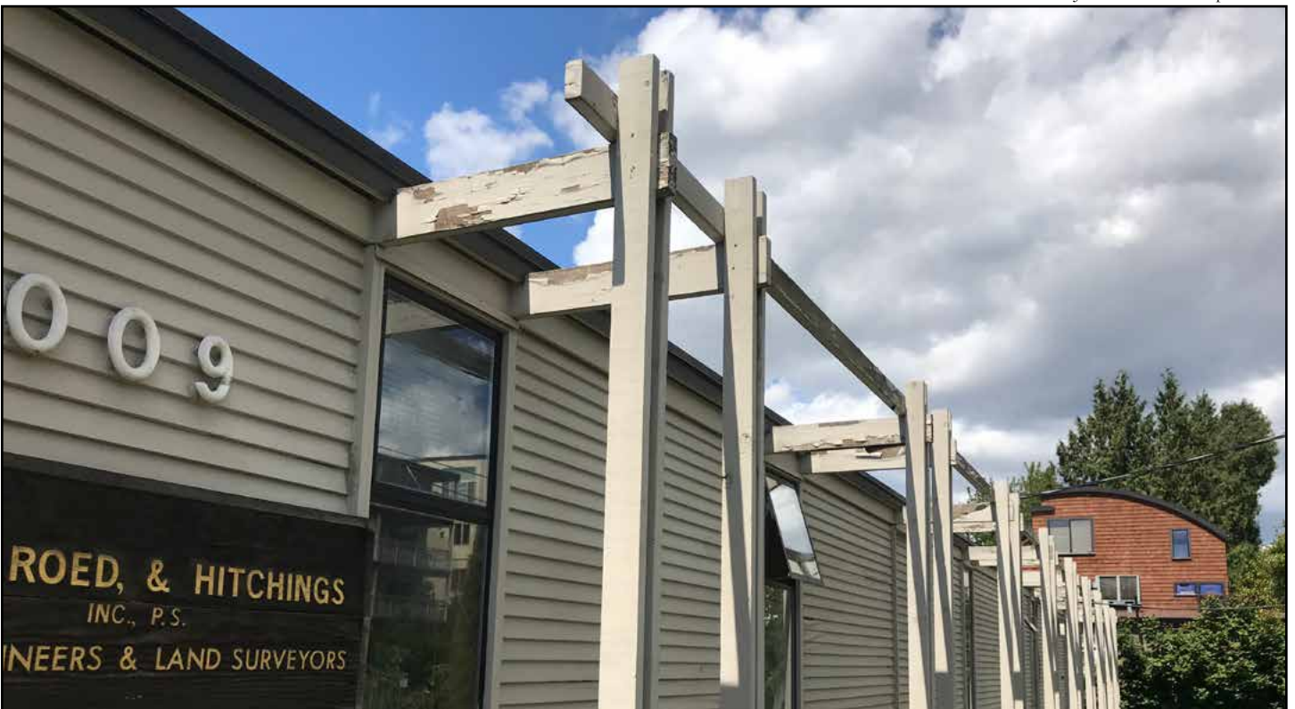
Figure 17 • 2009 Minor Avenue E, detail of brise soleil at eastern façade
