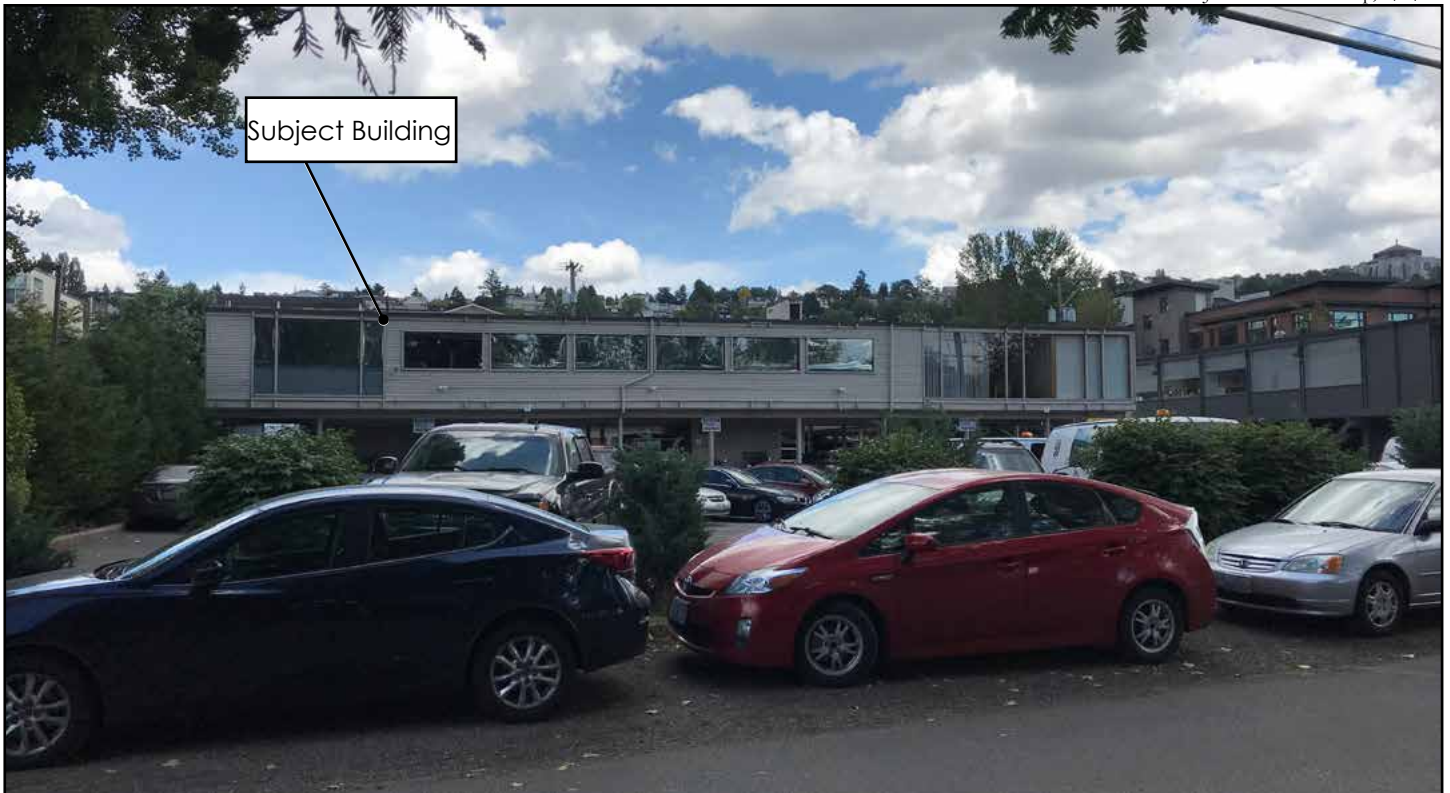
Figure 5 • View C - Viewing east across Fairview Avenue E
