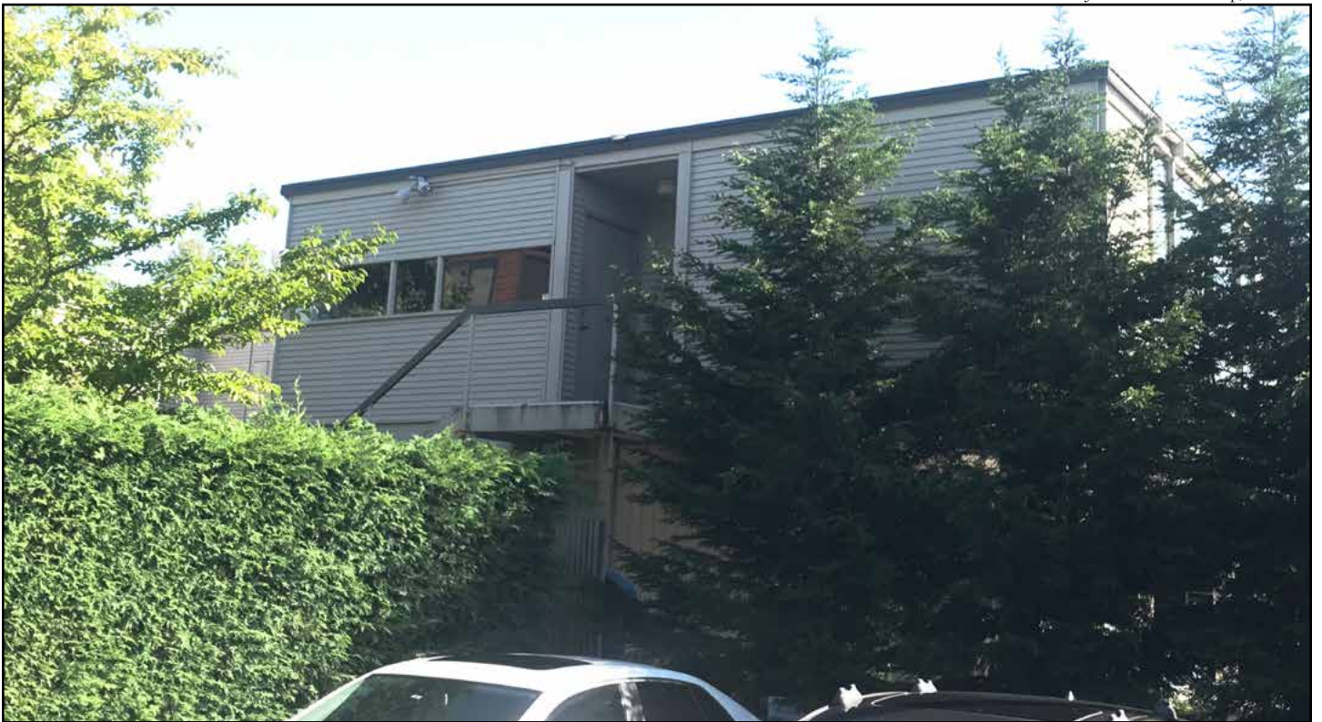
Figure 21 • 2009 Minor Avenue E, northern façade, western wing
