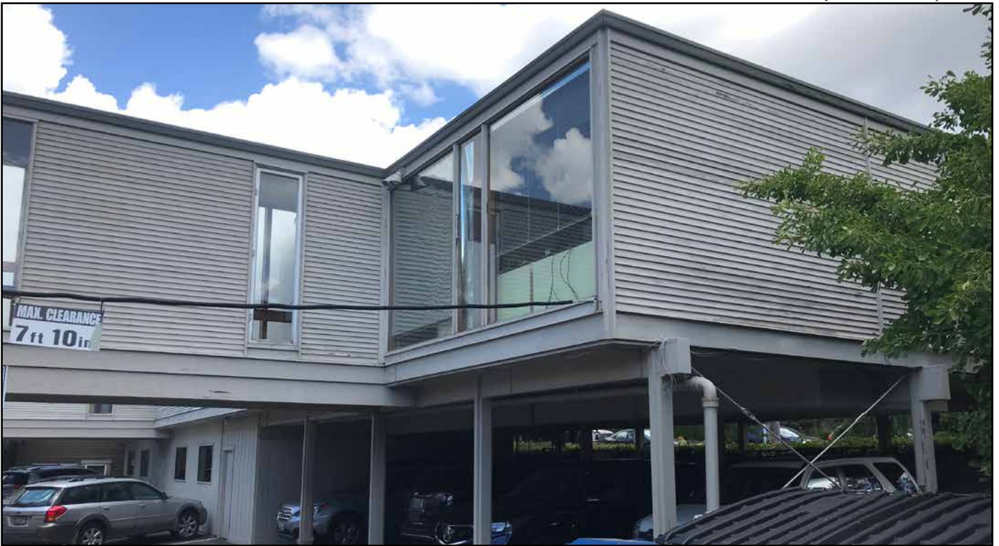
Figure 18 • 2009 Minor Avenue E, partial southern façade
