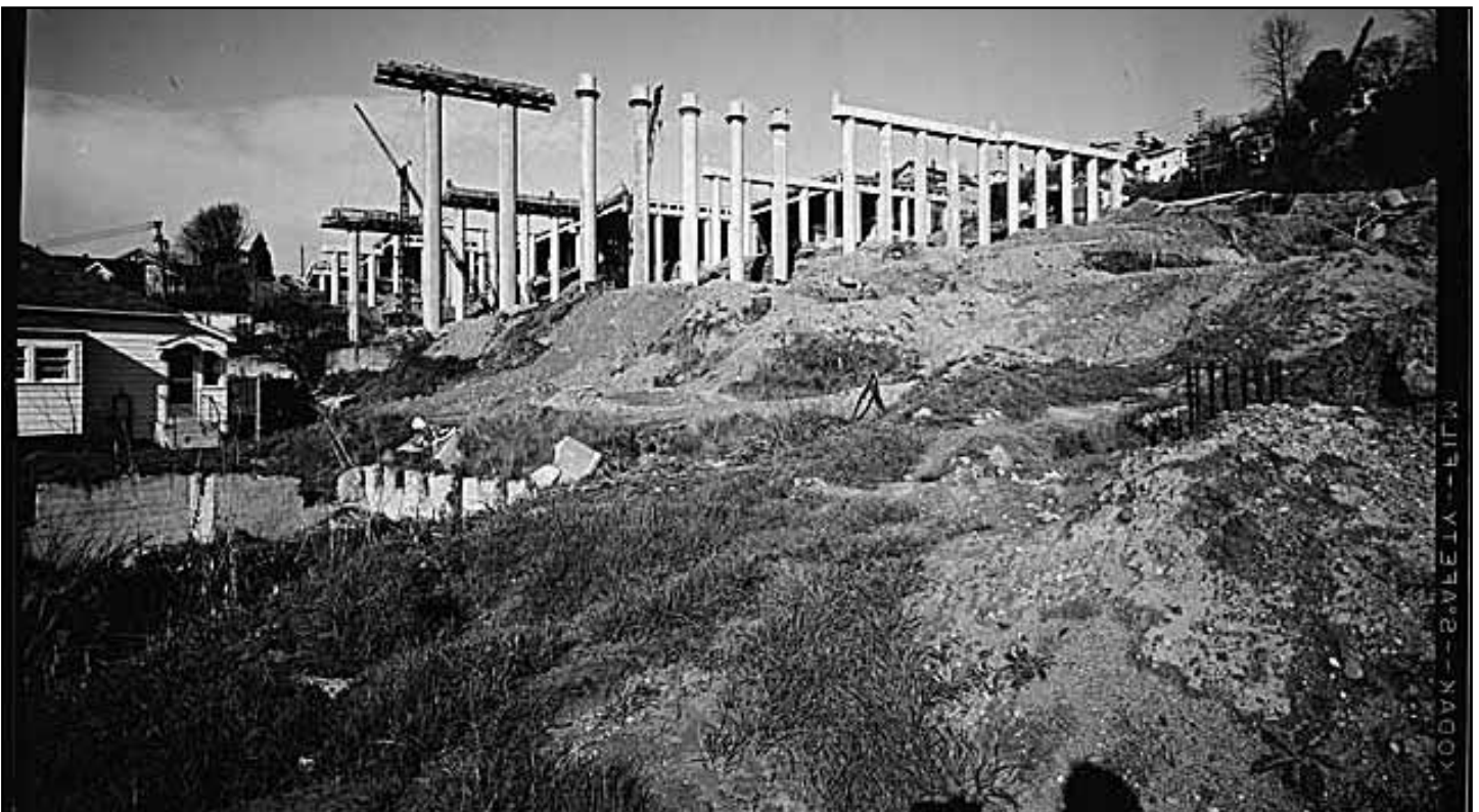
Figure 38 • Construction of Interstate 5, viewing from Eastlake Avenue E and Lakeview Avenue N
