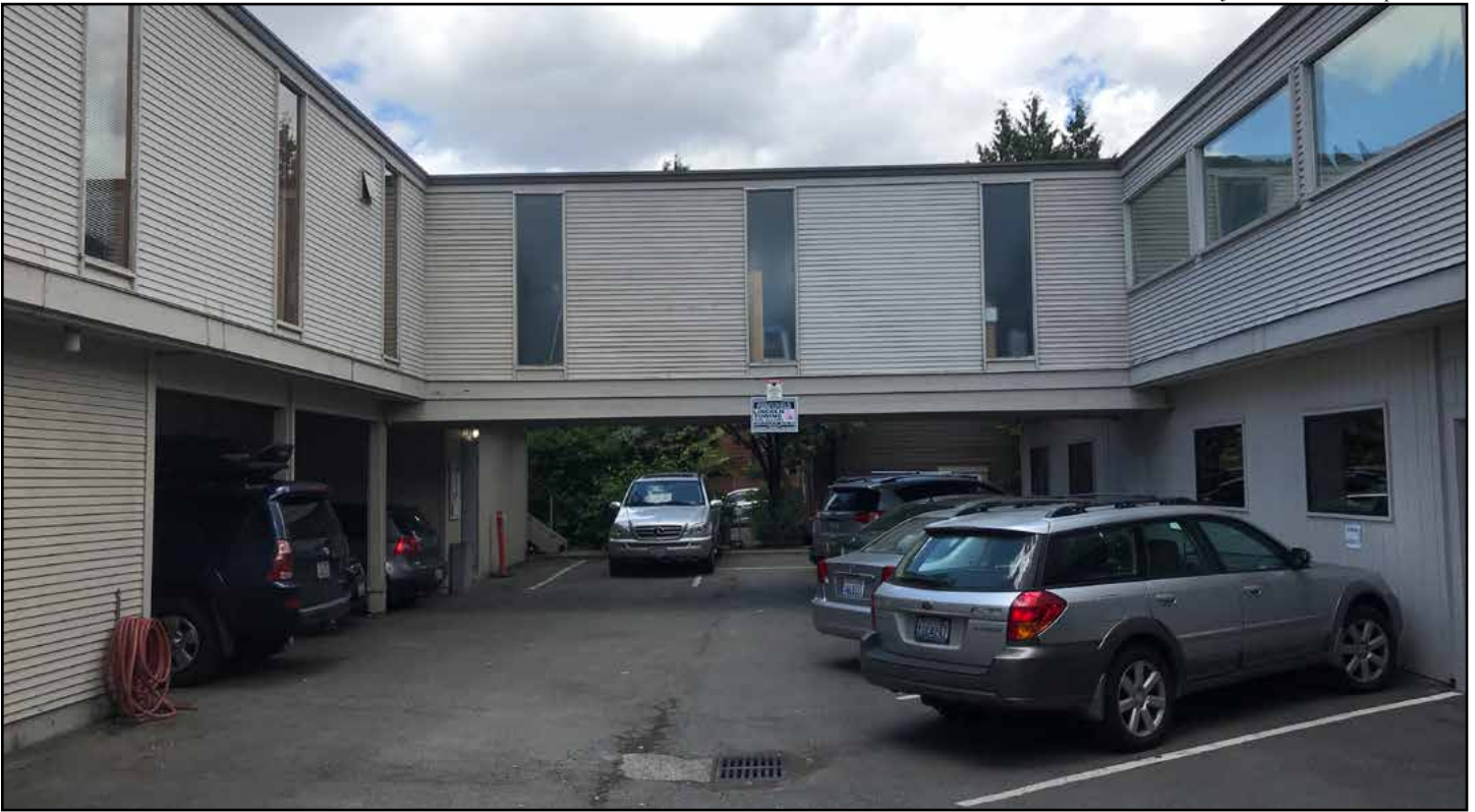
Figure 24 • 2009 Minor Avenue E, central courtyard viewing north
