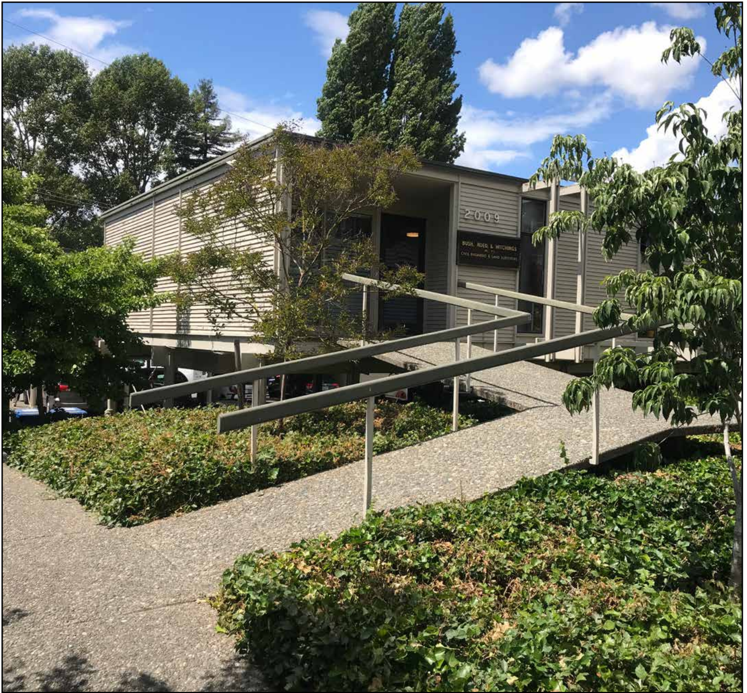
Figure 15 • 2009 Minor Avenue E, entry ramp at eastern façade
