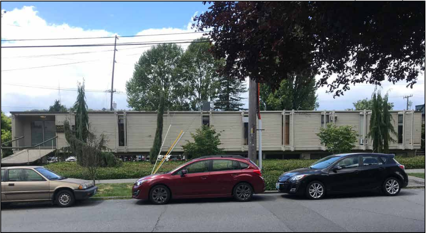
Figure 12 • 2009 Minor Avenue E, eastern façade
