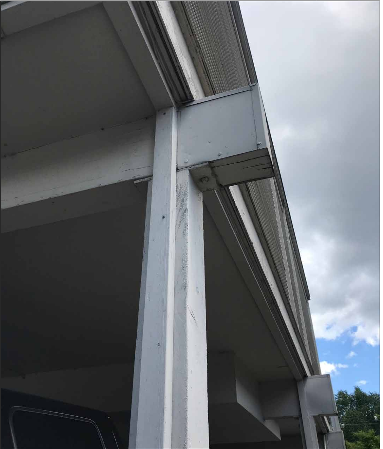
Figure 14 • 2009 Minor Avenue E, detail of column and beam end
