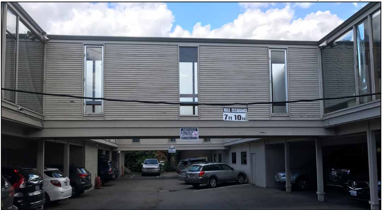
Figure 19 • 2009 Minor Avenue E, southern façade of southern elevated walkway
