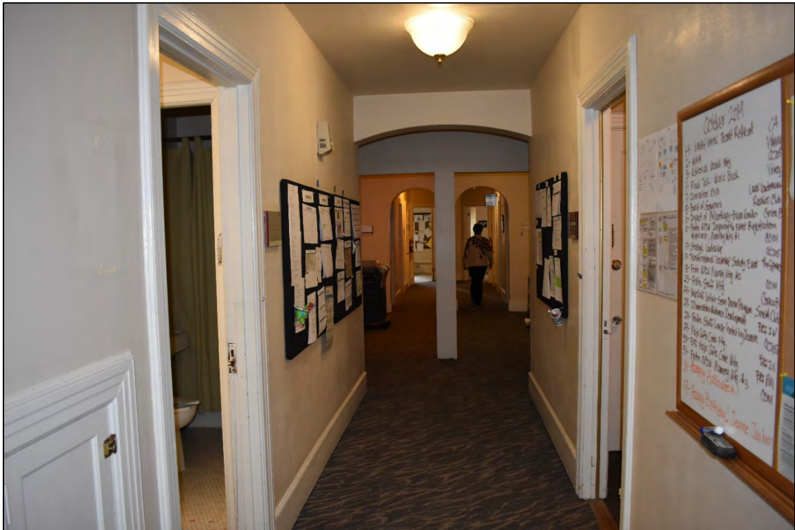
Fig. 26 – Interior, corridor in wing showing split hallway condition (see building plans)
