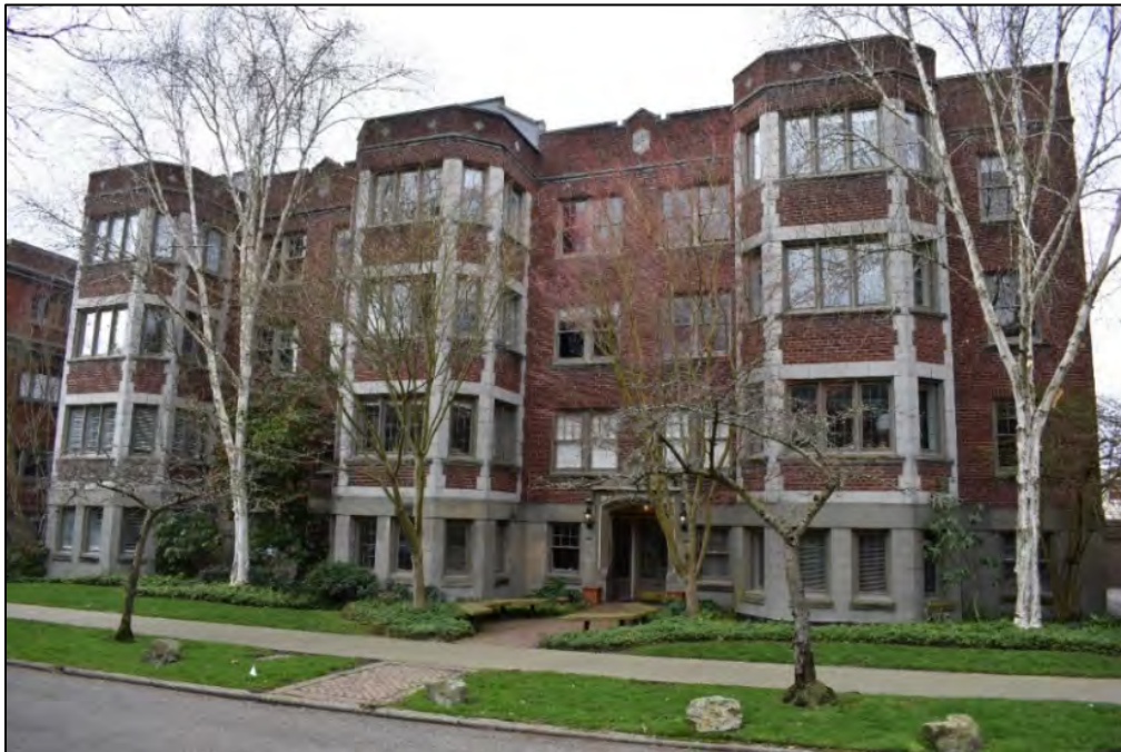
Fig. 62 - Comparable buildings: Highland Apartments (Stuart & Wheatley, 1924) at 931 11 th Avenue E, a Seattle landmark.
