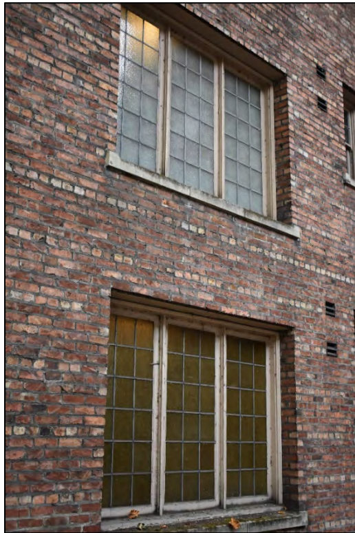
Fig. 16 - East elevation, south part, detail of masonry and windows
