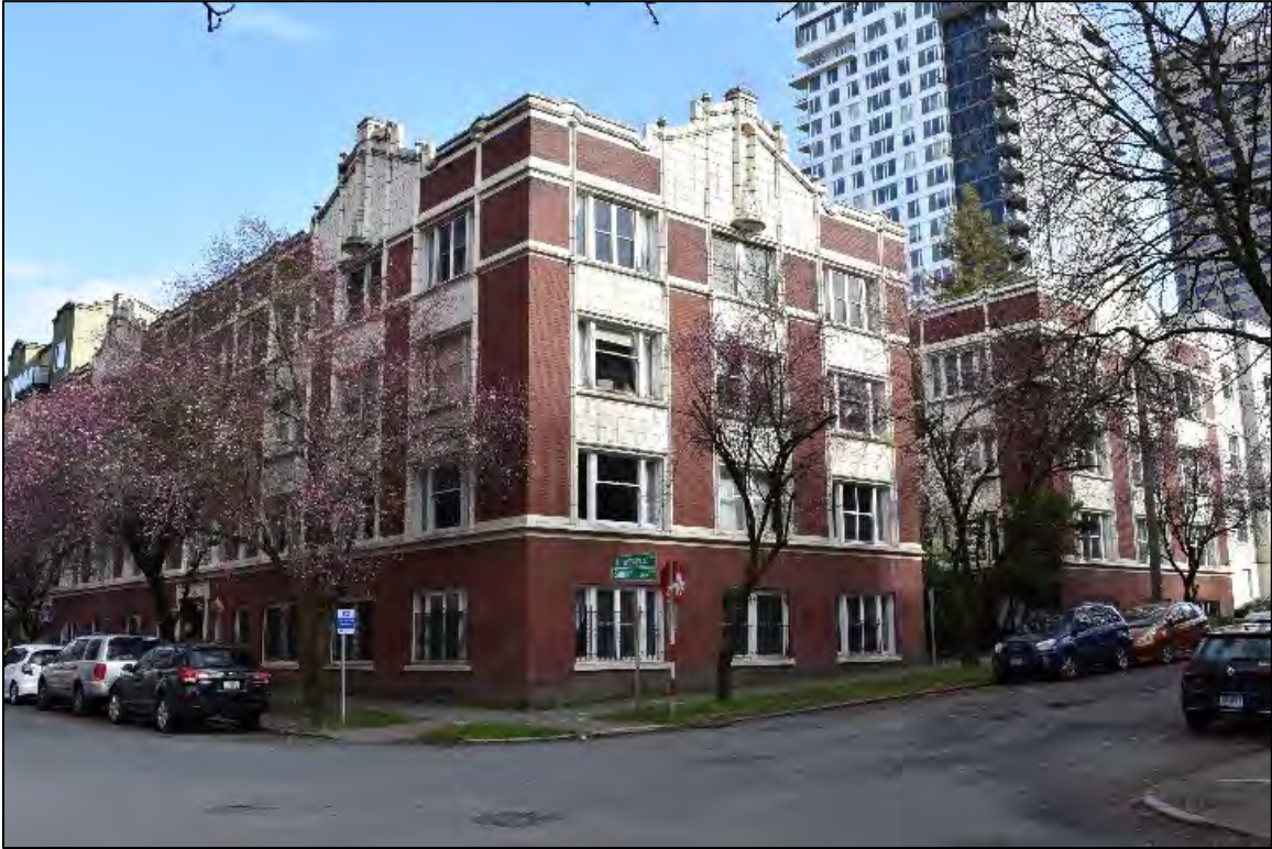
Fig. 53 – Comparable buildings on First Hill: The Arcadia (1916) at 1222 Summit Avenue.
