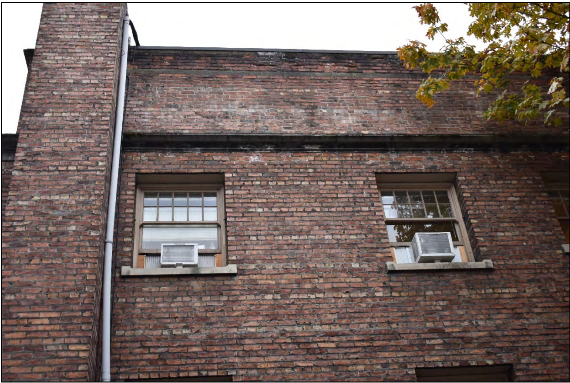
Fig. 15 - East elevation, south part, detail of masonry and windows
