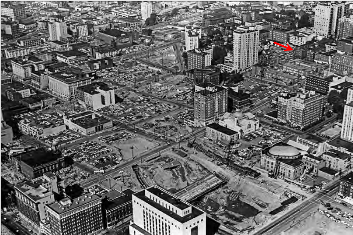
Fig. 47 – Circa 1961 view north showing path of demolition for I-5 highway construction. First Hill on right, downtown on left. Subject building indicated by arrow. (Paul Dorpat)
