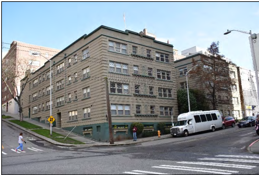
Fig. 55 – Comparable buildings on First Hill: John Alden (1923), top; Paul Revere (1924), middle; John Winthrop (1925), bottom two photos.
