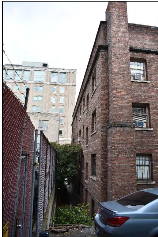
Fig. 18 – South elevation, view west from southeast property corner
