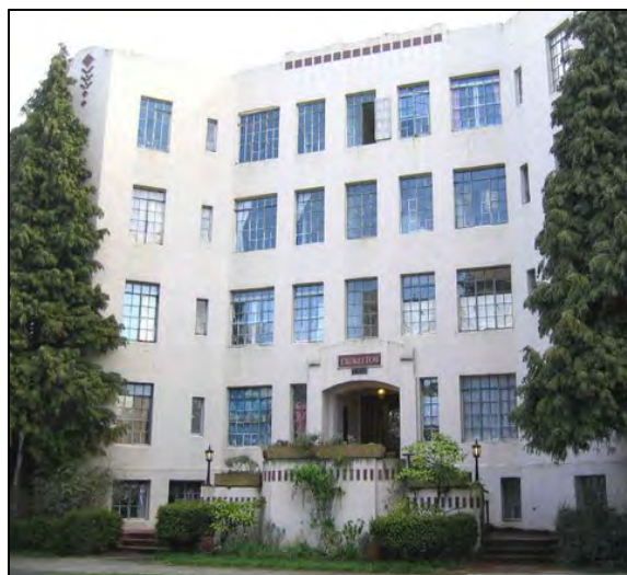
Fig. 52 – Other work by builder Sheble & Snyder: Laurelton Apartments (Frank Baker, 1927) at 1820 16 th Avenue (DON)
