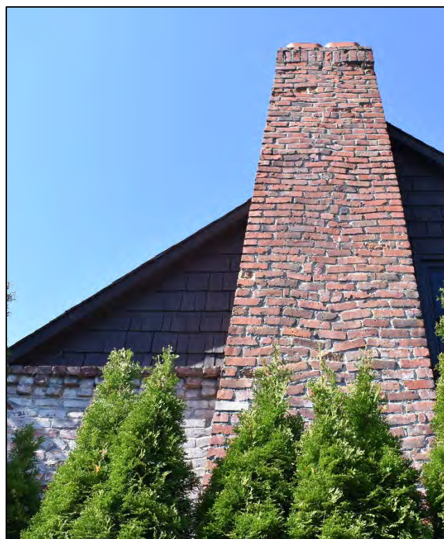
Fig. 41 – Detail showing decorative brickwork.
