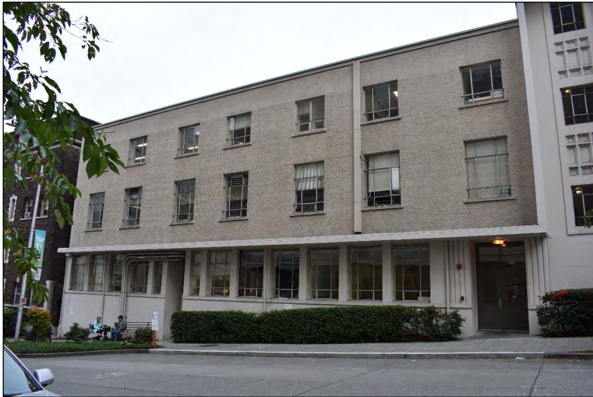
Fig. 8 - West elevation, north part.
