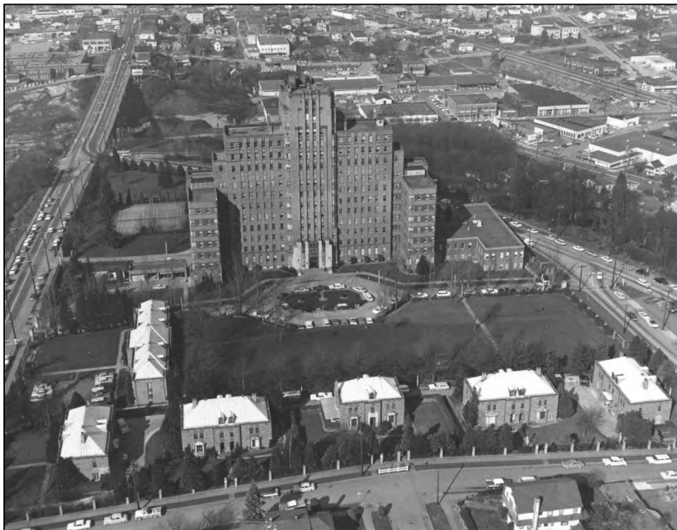
Fig. 76 – U.S. Marine Hospital (Bebb & Gould, 1932-33, with John Graham Sr.). The smaller buildings clustered around the large hospital tower housed physicians and staff; the nurses' home was the larger building in the complex at left. (SMA 181015)
