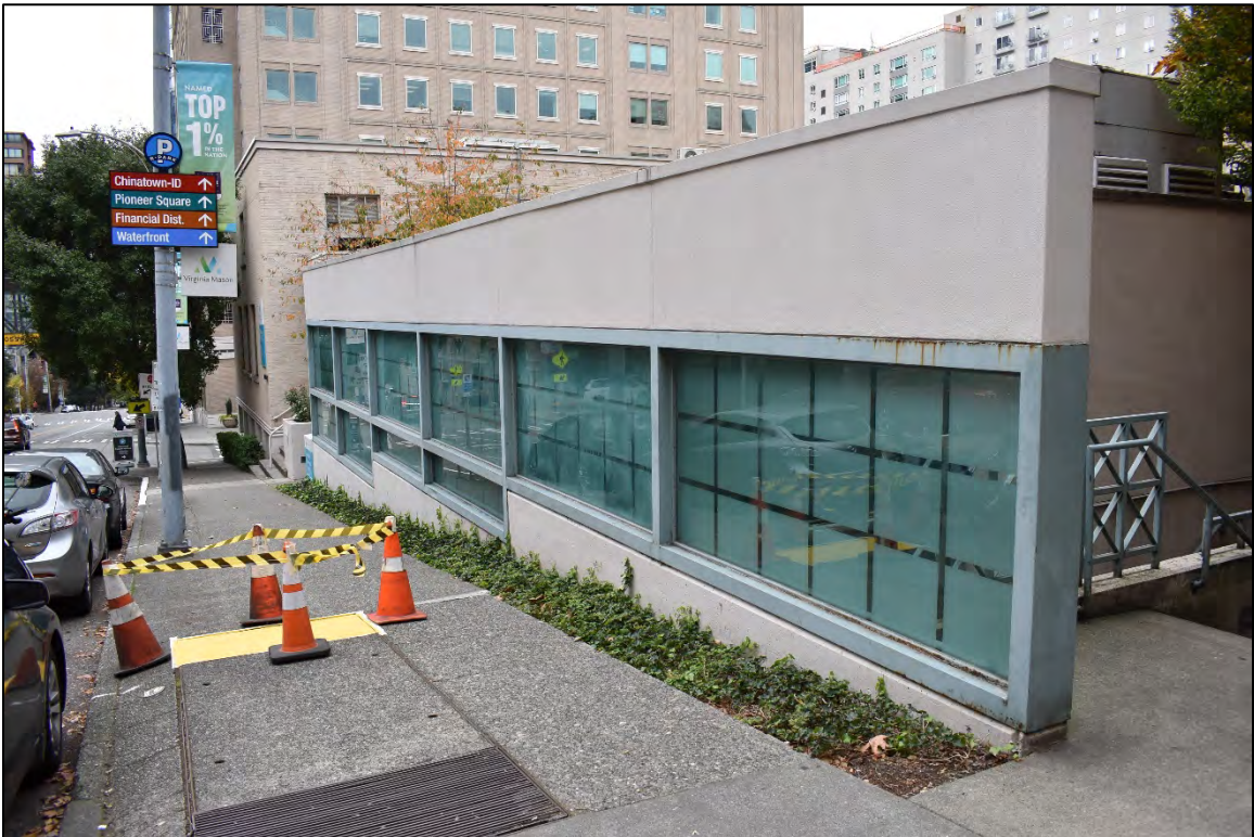
Fig. 30 – MRI Building, south elevation, view west.
