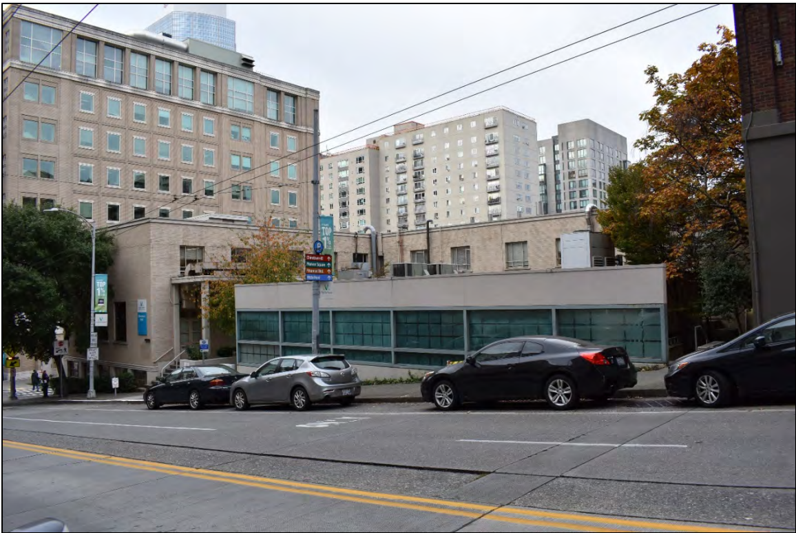
Fig. 13 – South and east elevations, and MRI Building.
