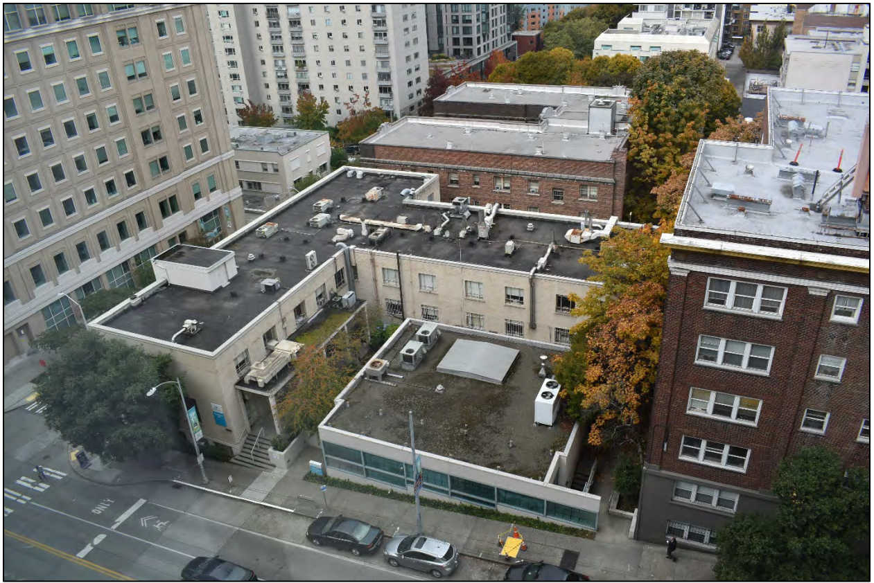
Fig. 5 – Aerial photo of site, oblique view to the northwest.
