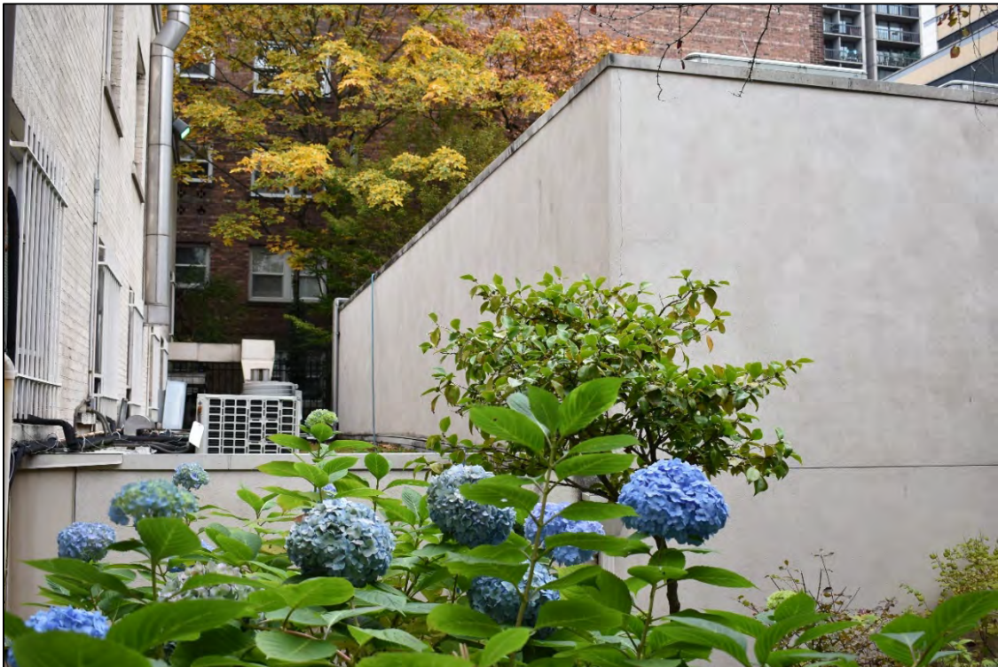
Fig. 32 – MRI Building, north and west elevations at center and right, view east.
