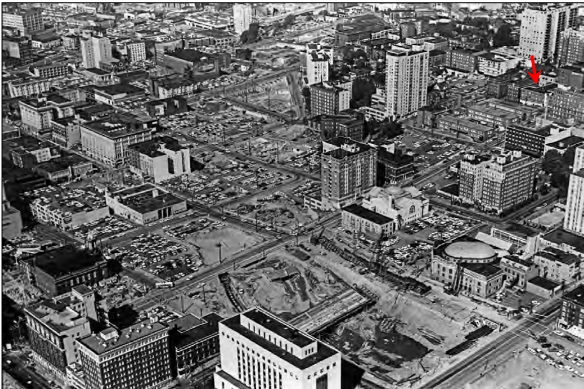
Fig. 47 – c.1961 view north showing path of demolition for I-5 highway construction. First Hill on right, downtown on left. Subject building indicated by arrow. (Paul Dorpat)
