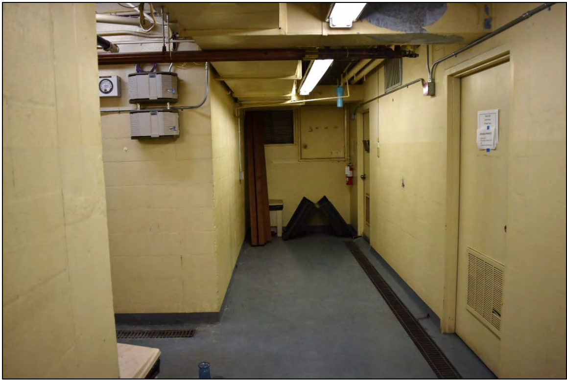
Fig. 21 – Interior, basement level, typical corridor at east side of building.
