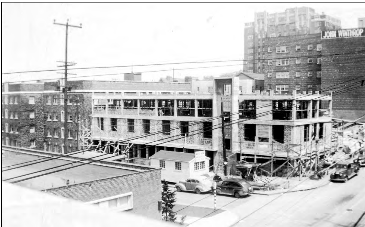
Fig. 56 - 1945 view of Blackford Hall under construction. (VMA PH1312a)
