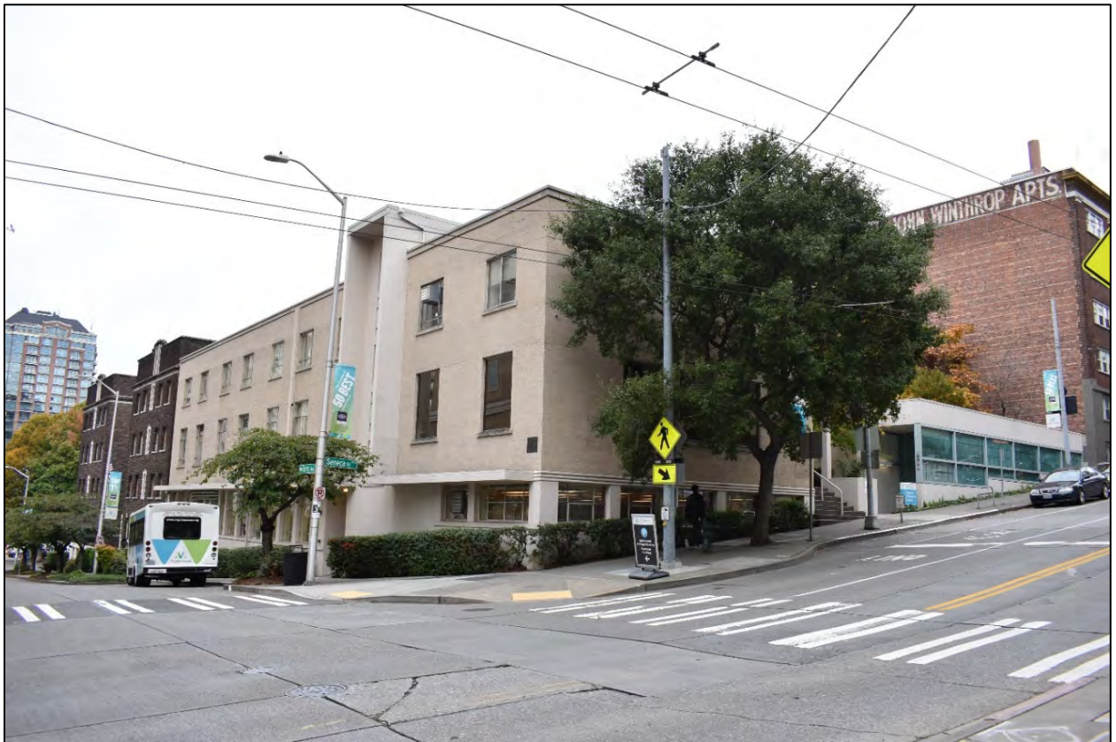
Fig. 6 – Context view towards site from the southwest.
