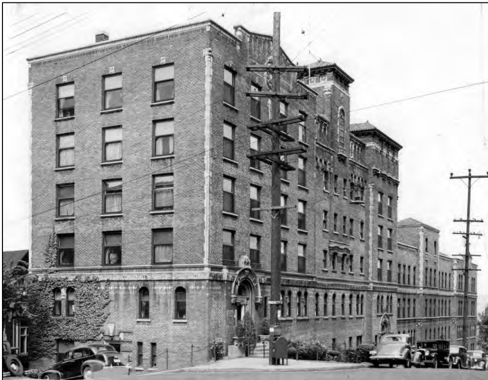
Fig. 49 - Virginia Mason Hospital, original 1920 structure at left, with addition (John Graham Sr., 1928) visible at far right. (Paul Dorpat)
