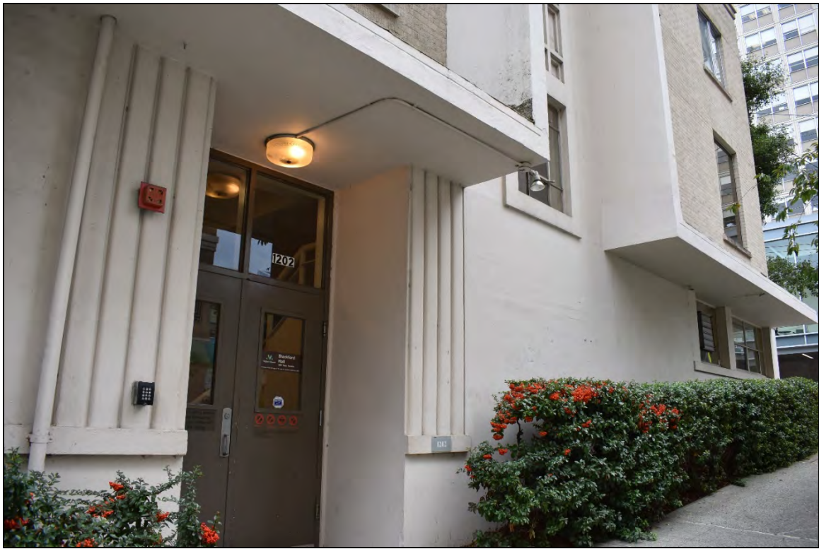
Fig. 11 - West elevation, detail of main entry at basement level.
