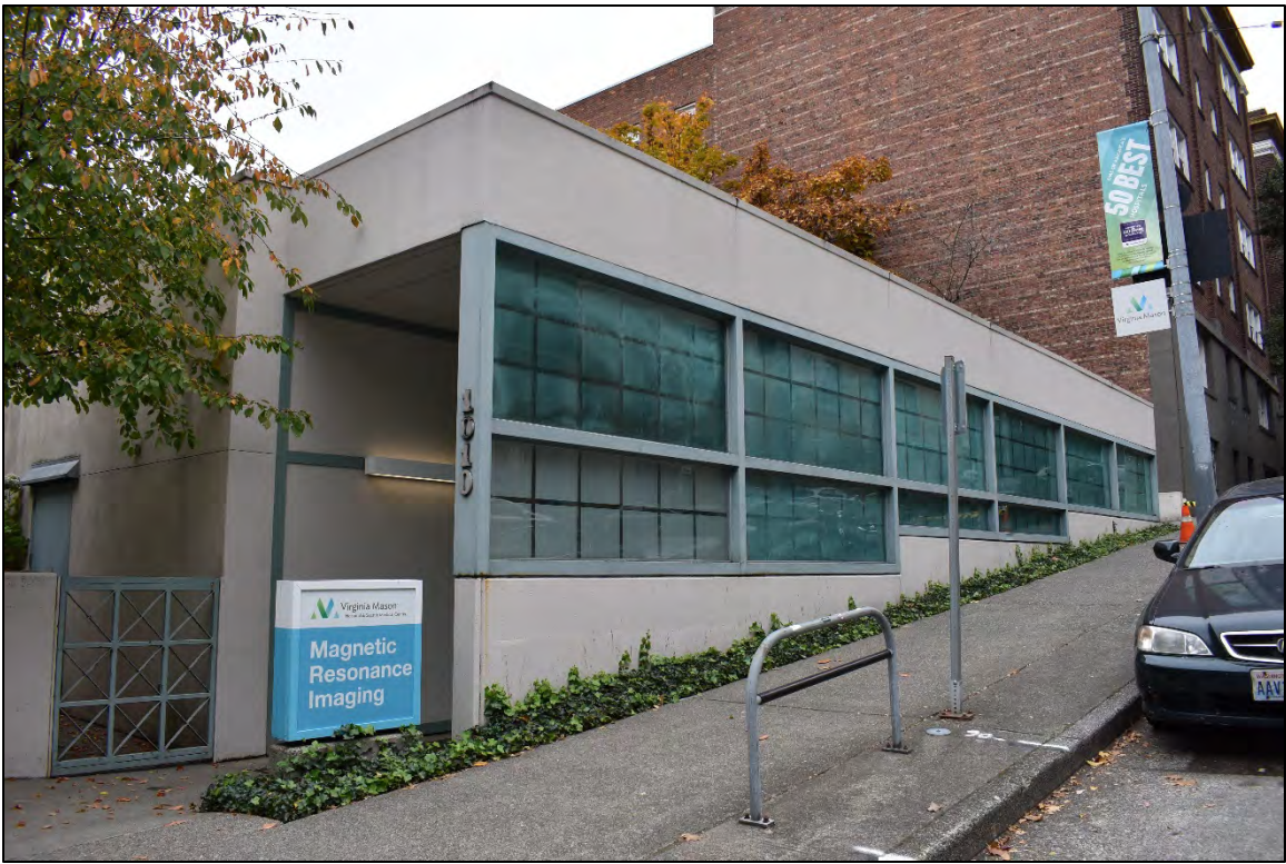
Fig. 29 – MRI Building, south elevation, view east.
