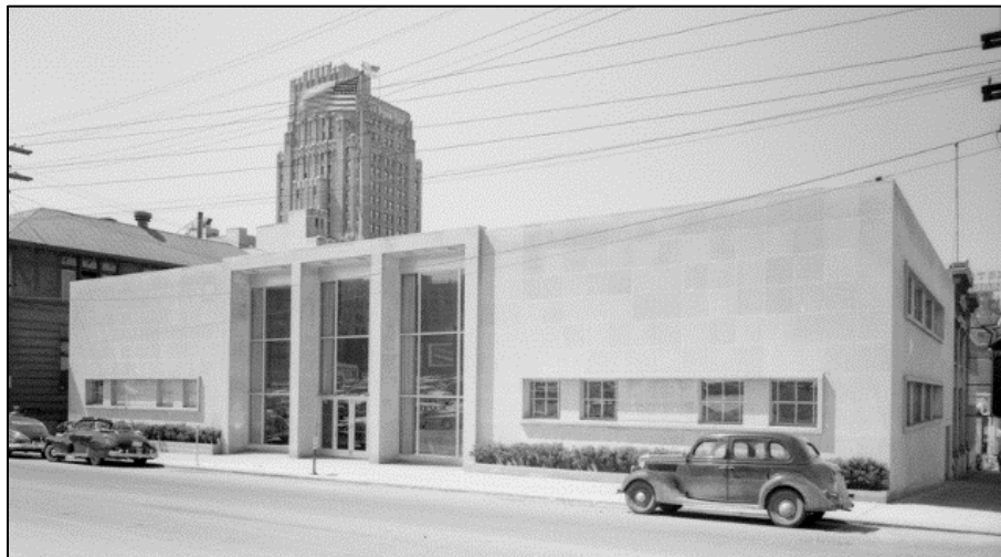
Fig. 97 – American Legion Memorial Building (NBBJ, 1945-46, demolished) at 620 University Street. (UWSC DM3303)
