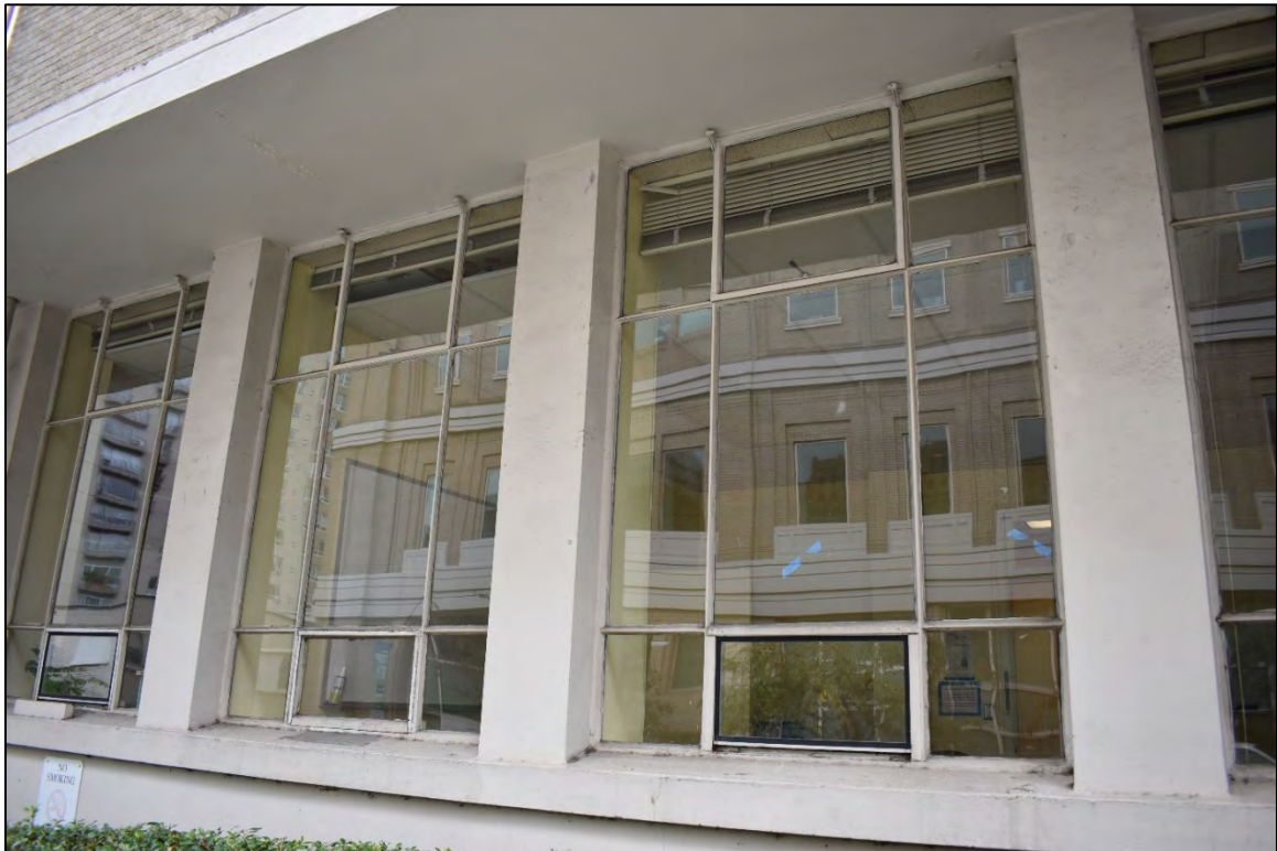
Fig. 12 - West elevation, detail of basement level windows.
