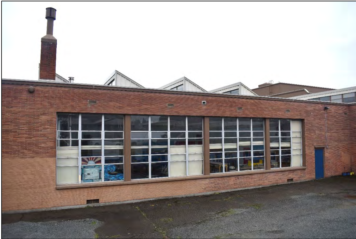
Fig. 42 – West wing, west facade, north part, showing shop classrooms. Note sawtooth roof monitors.
