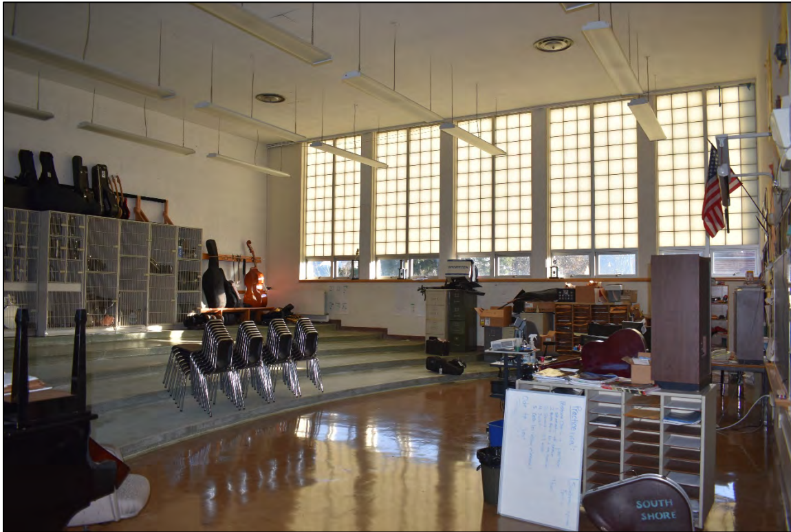
Fig. 76 – Interior, orchestra room. Windows are Kalwall replacements of original glass block.
