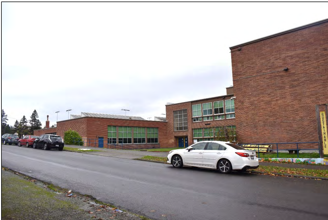
Fig. 43 – West wing, west facade, central part, view northeast showing small west courtyard. Note sawtooth roof monitors.
