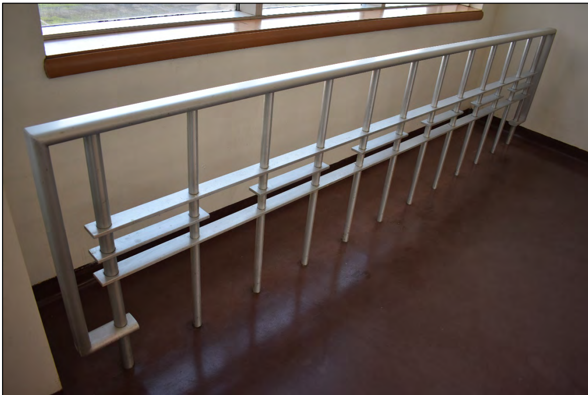
Fig. 59 – Interior, typical secondary building entry and stair, showing stair landing window guardrail.
