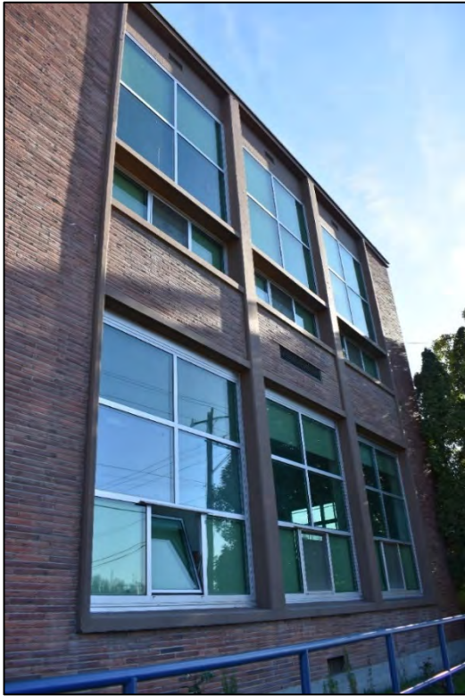
Fig. 52 – West wing, west facade, south part, detail of windows, showing projecting window surround with flush sills, jambs, and headers.
