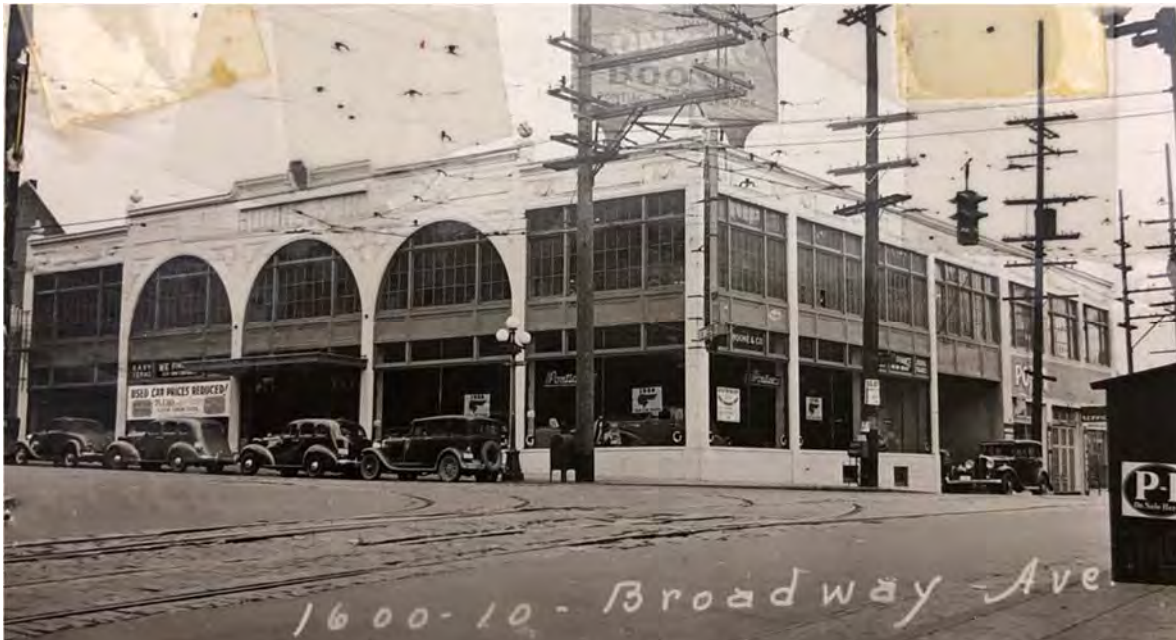
Fig 36 The former Boone & Company Pontiac dealership, at the northeast corner of Broadway and E. Pine, shown in a 1937 tax record photo. (King County Tax Assessor property record card, Puget Sound Regional Archives)
