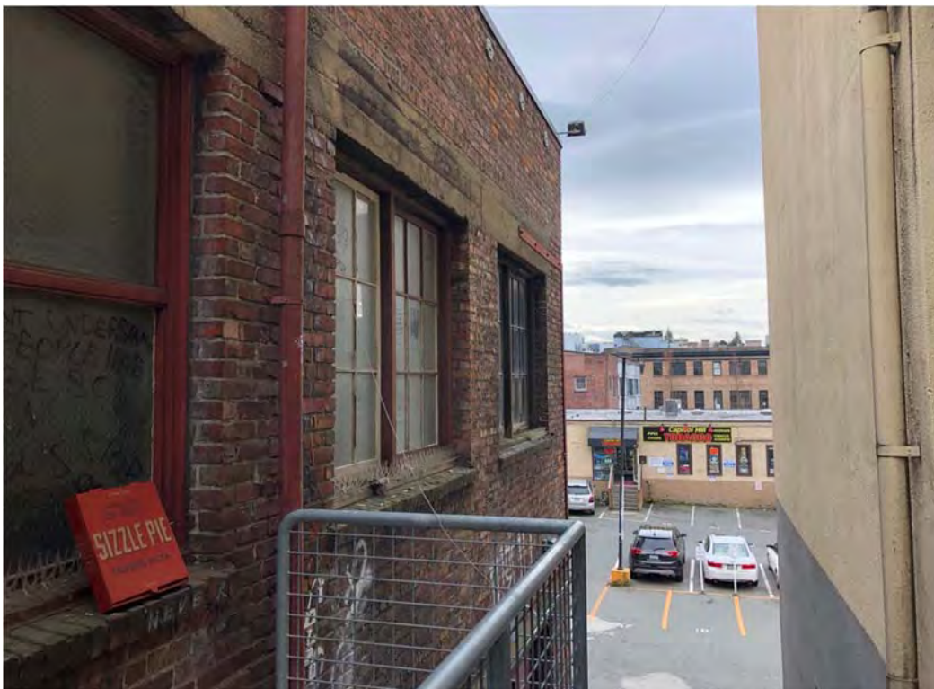
Fig 20 View south from the exterior landing between the buildings, second story.
