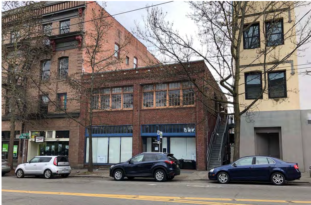
Figs 11 & 12 View looking southeast across E. Pine Street, toward the primary north façade and west façade of the building. The top photo is the 1937 tax record photo (Puget Sound Regional Archives), for comparison with the same view of the building today.
