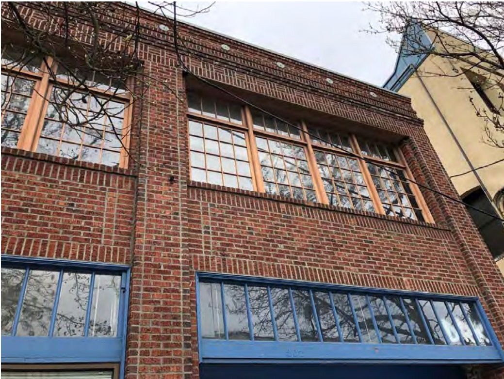
Fig 17 View looking up at the original windows, primary north façade.
