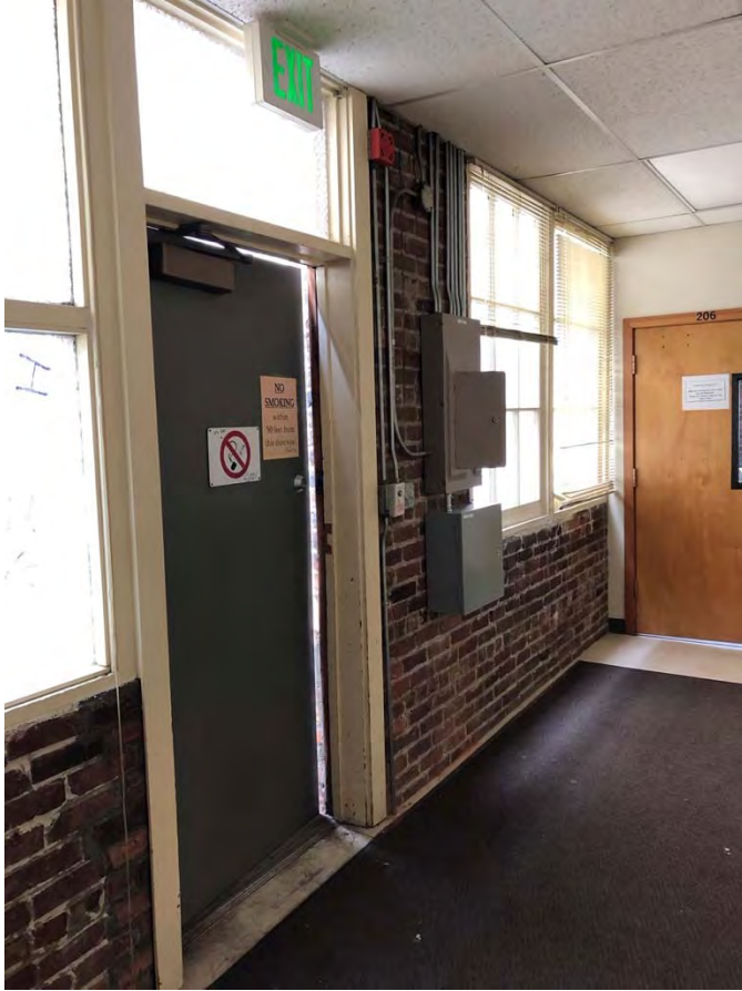
Fig 29 Left, view at the second-floor "entry lobby" off the exterior landing.
