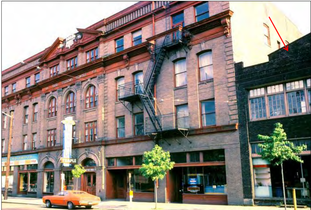
Fig 42 A ca. 1975 view of the Odd Fellows Temple includes the eastern portion of the subject building. (Seattle Municipal Archives, item no. 182276)
