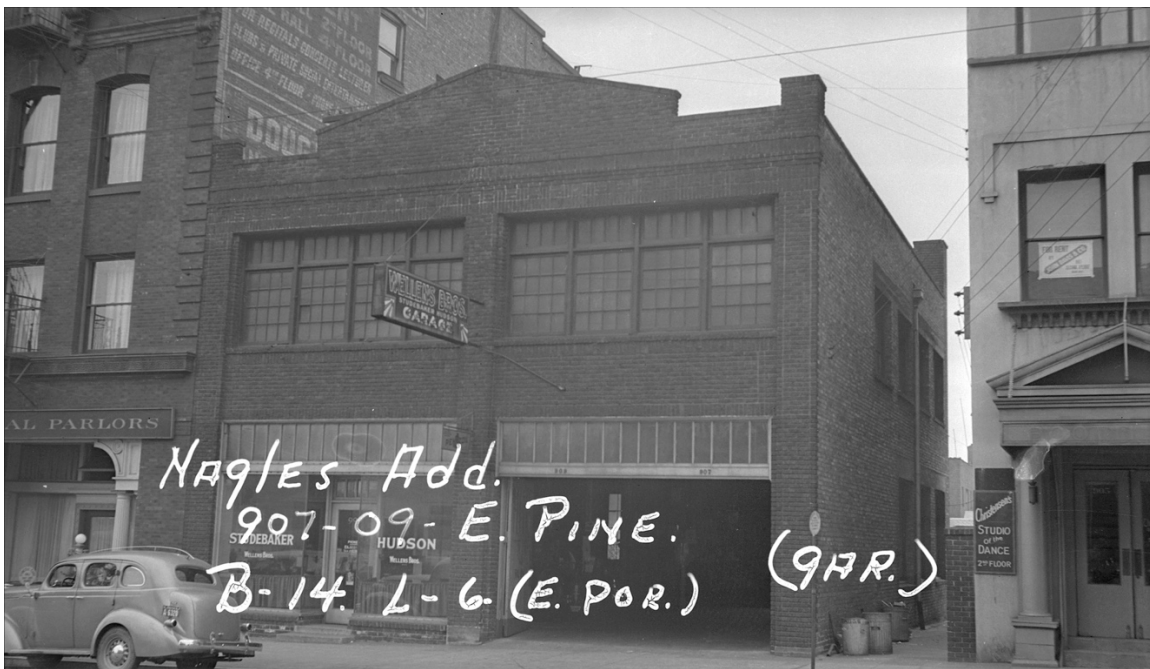
Figs 39 & 40 Two 1937 views show the north façade (top) and the north and west façades (above). (King County Tax Assessor property record card, Puget Sound Regional Archives)
