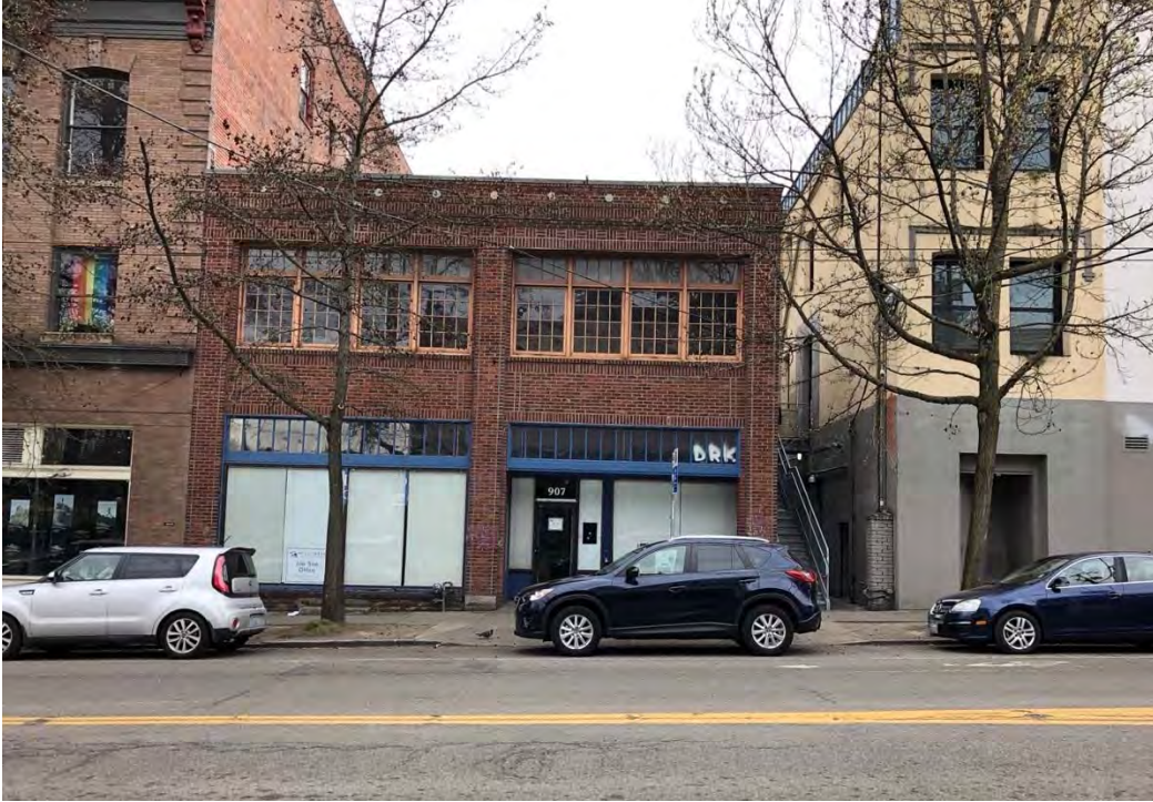
Fig 13 View looking south at the primary north façade.
