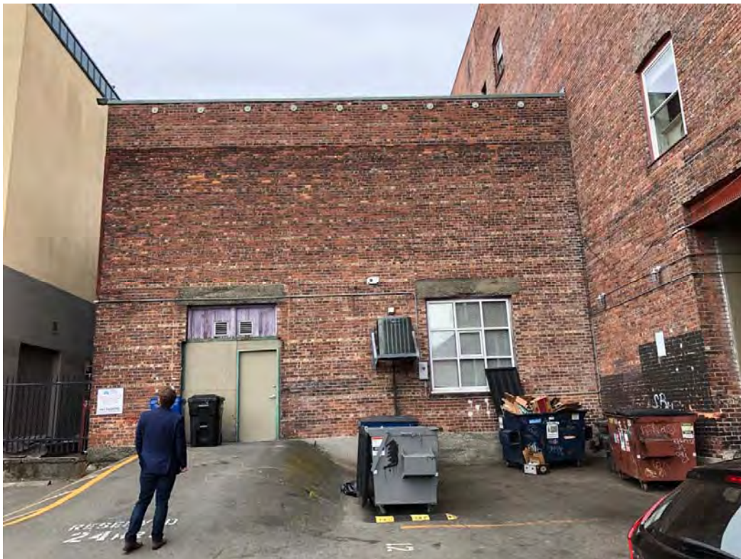
Fig 22 View north at the south façade.
