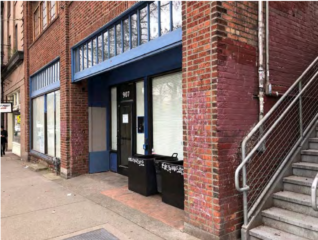
Fig 14 View northeast along the storefront portion of the north façade.
