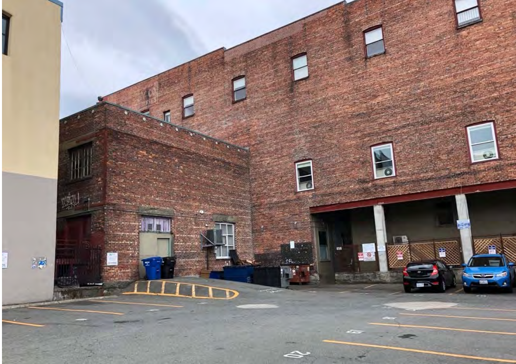
Fig 21 View northeast from the parking lot behind the building, showing south façade. (Immediately east is the west wall of the Odd Fellows Temple.)
