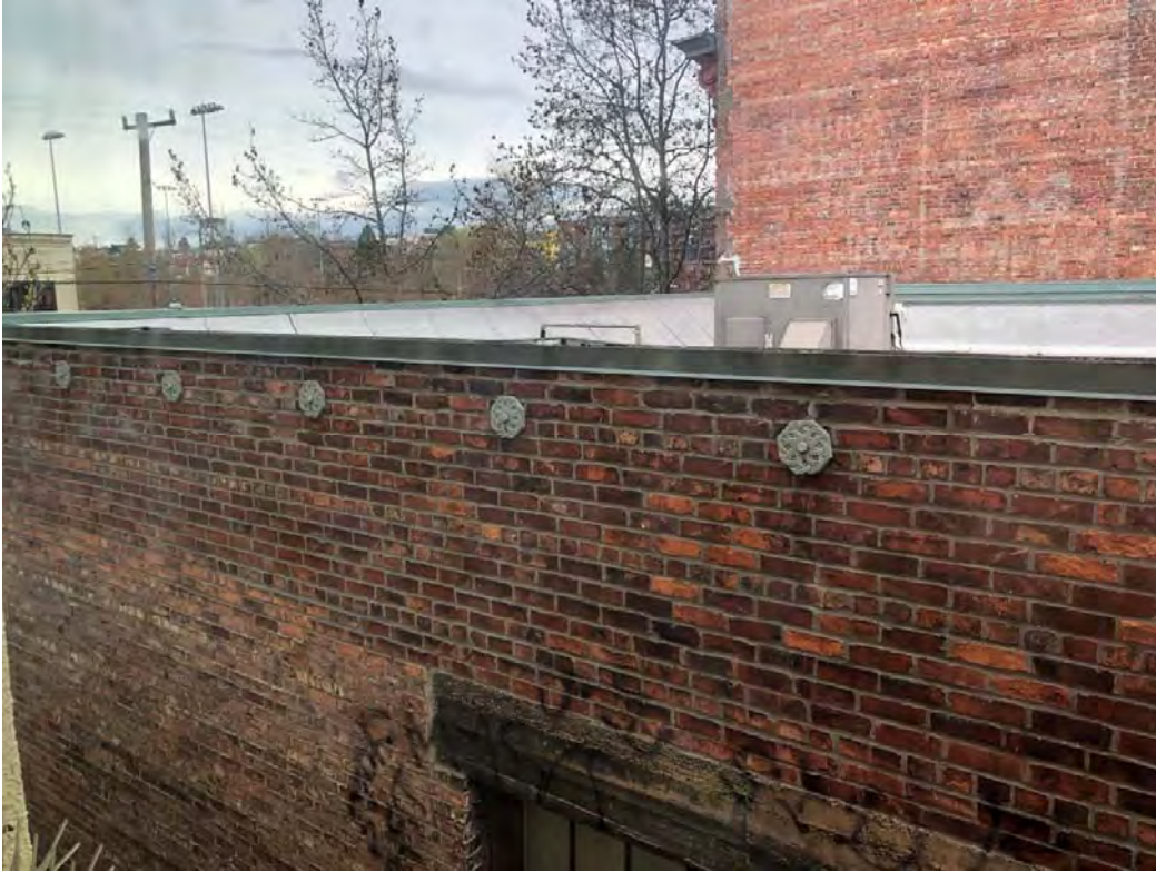
Fig 23 View northeast, partially showing the west parapet.
