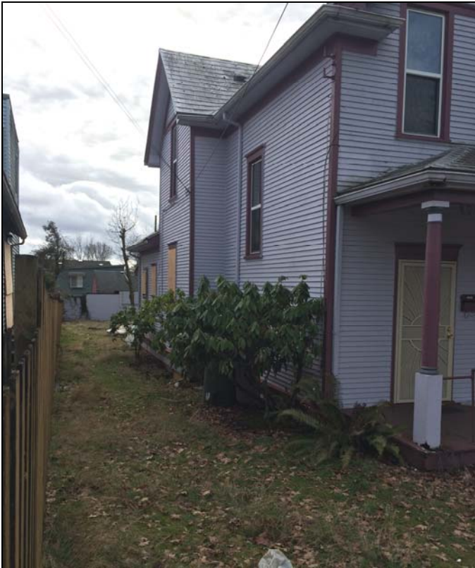
Fig. 21 View southwest along the east façade of the house.
