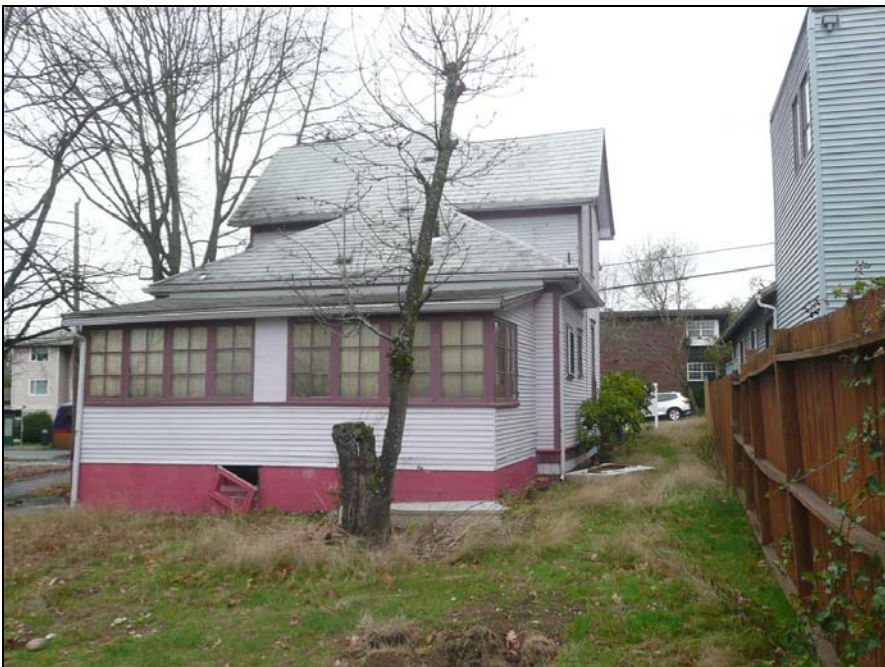
Fig. 22 View north/northwest from the backyard showing the south side of the house, which is now an enclosed sunroom.
