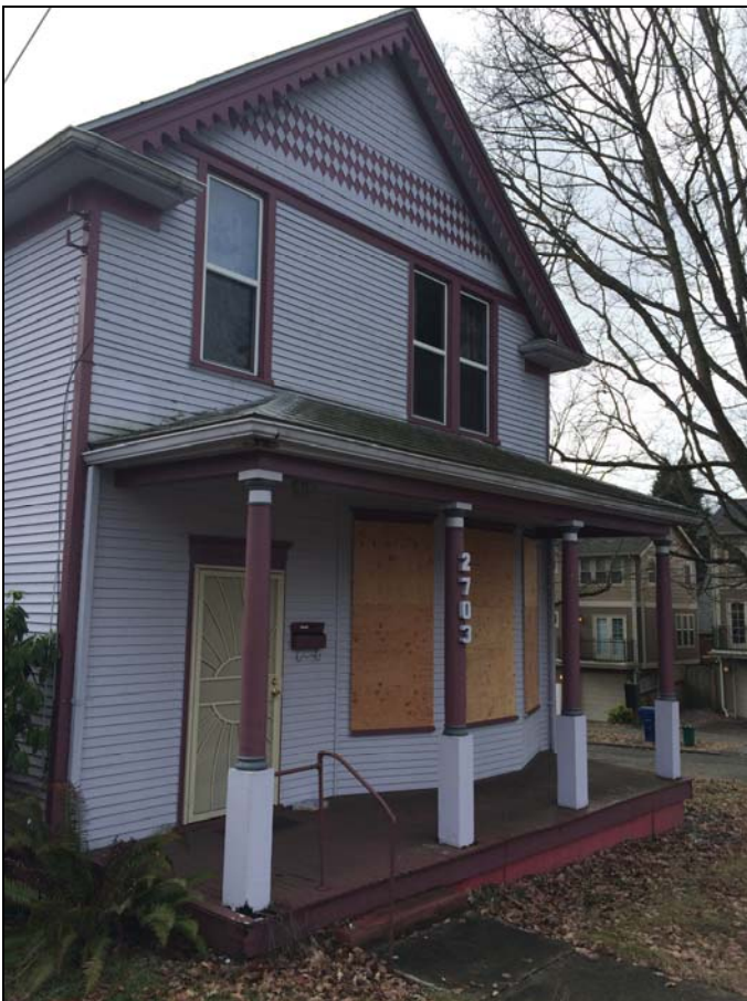
Fig. 20 Looking southwest at the primary north façade.
