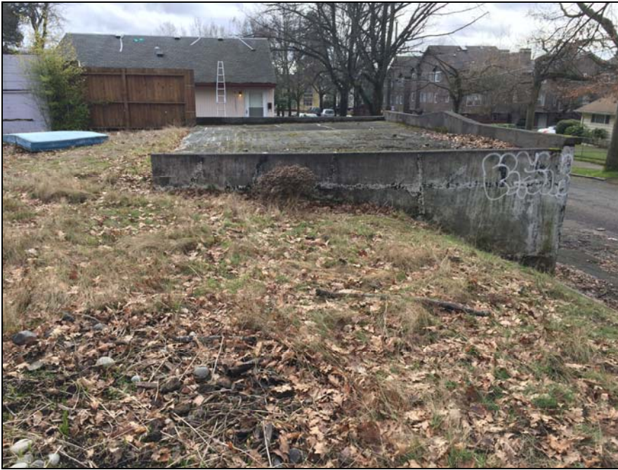
Fig. 22a View south showing the southwest corner of the backyard, including the north wall and roof of the garage.
